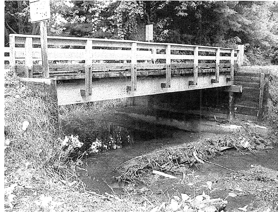
8.2843901 B-3614 BUNCOMBE Co. Bridge 300 on SR-1141 OVER HOMINY CREEK
