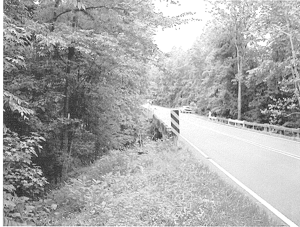
Photograph 5: View of Left Profile Upstation (Looking from EB1-A)
