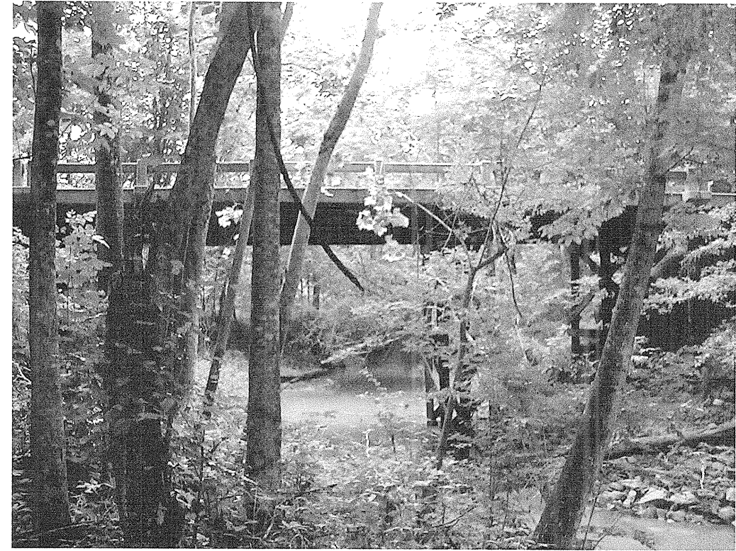
Photograph 7: View of Bridge 108 Over Lower Barton's Creek Looking Downstream
