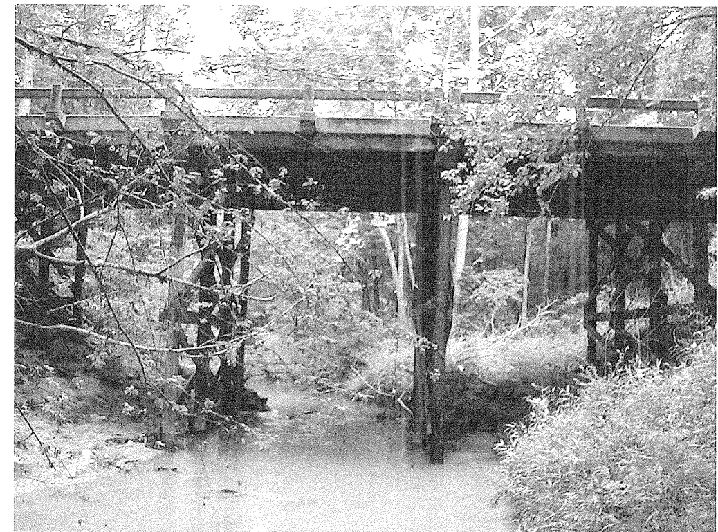
Photograph 8: View of Bridge 108 Over Lower Barton's Creek Looking Upstream
