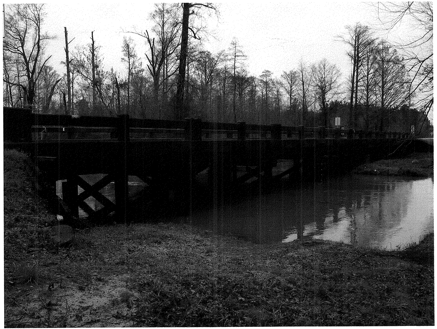
Looking northeast towards End Bent 2
