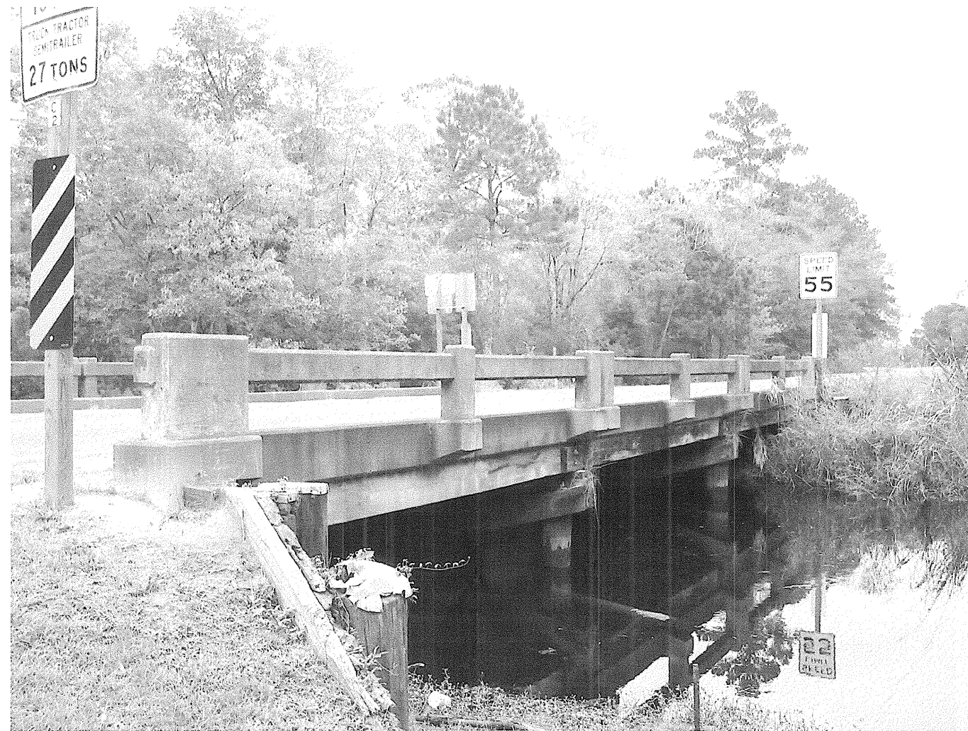
Looking east towards End Bent 2
