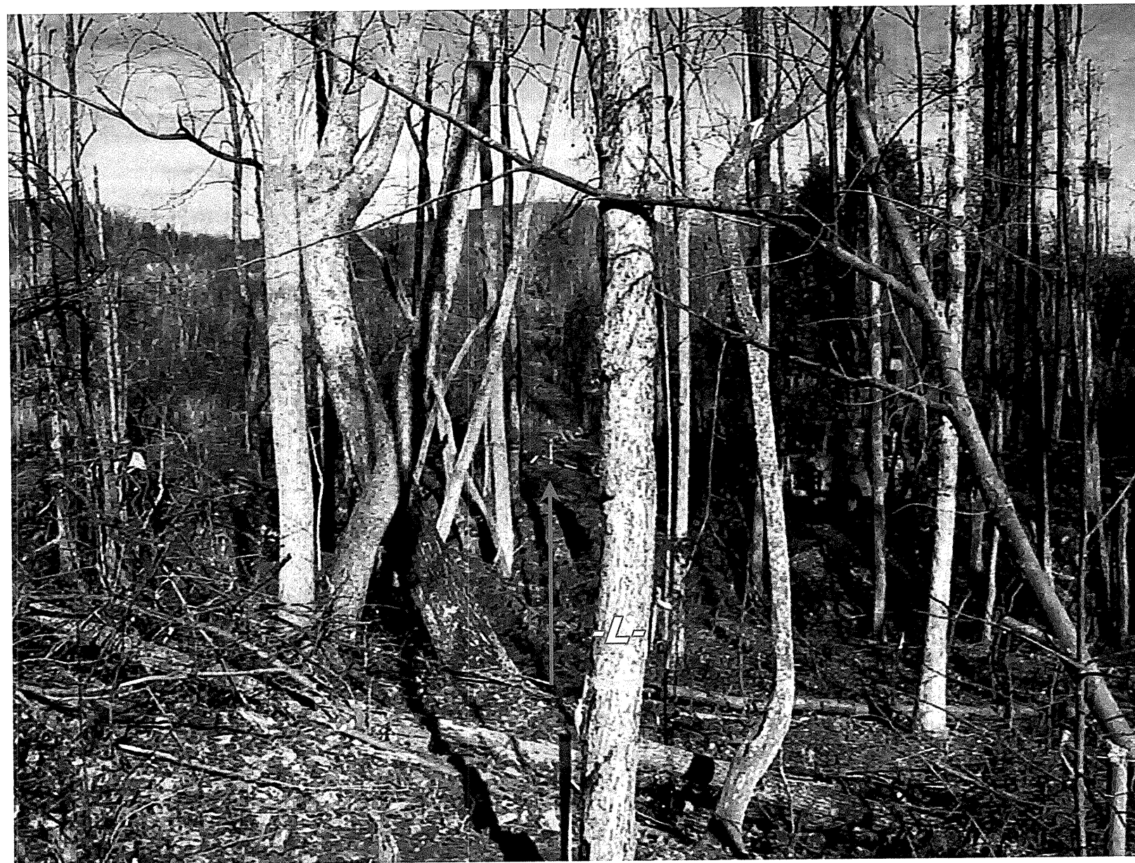
Photo looking up station along -L- from End Bent 1 toward End Bent 2. SBL to left and NBL to right.
