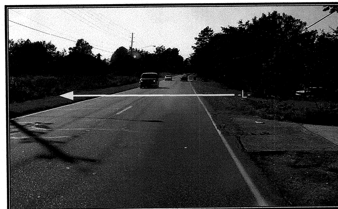
View behind (west) along existing -Y3- (NC 42). -L- shown approximately.
