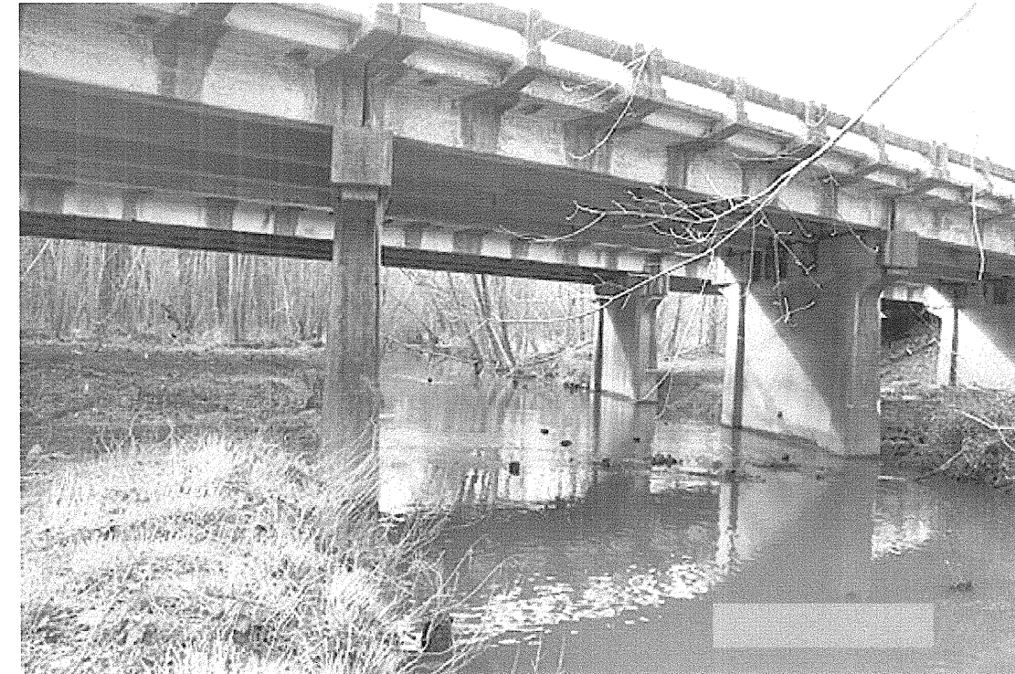
Photograph 7: View Downstream from Upstream Side of Bridge
