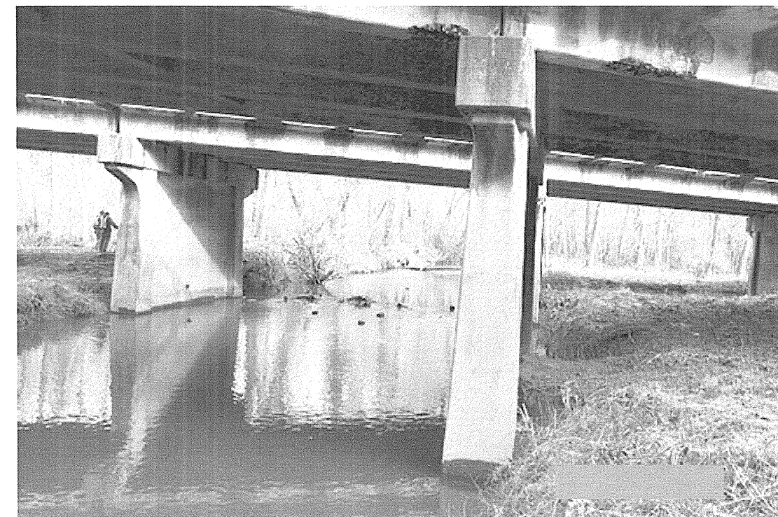
Photograph 8: View Upstream from Downstream Side of Bridge
