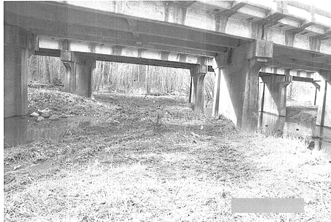
Photograph 5: View Along Bent-2 From Left to Right
