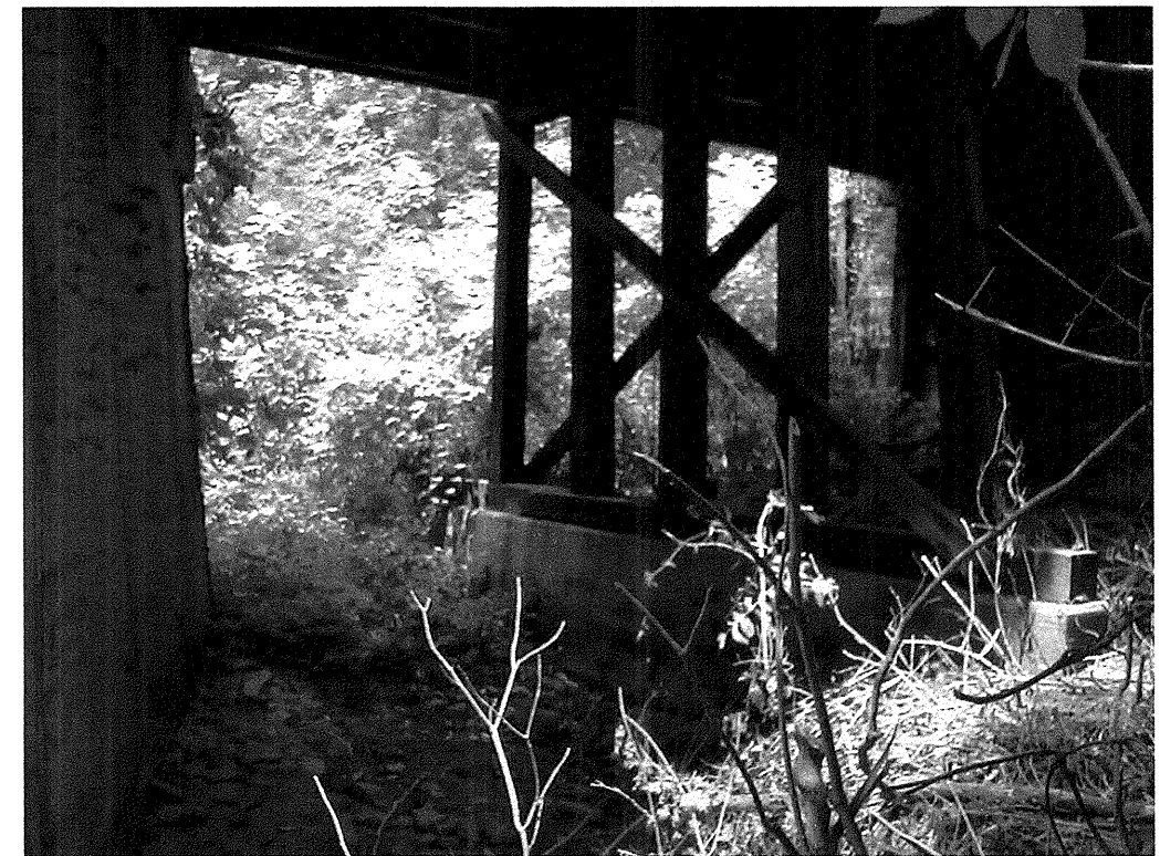
Photograph 3: View of Proposed Bent 2 From Right to Left
