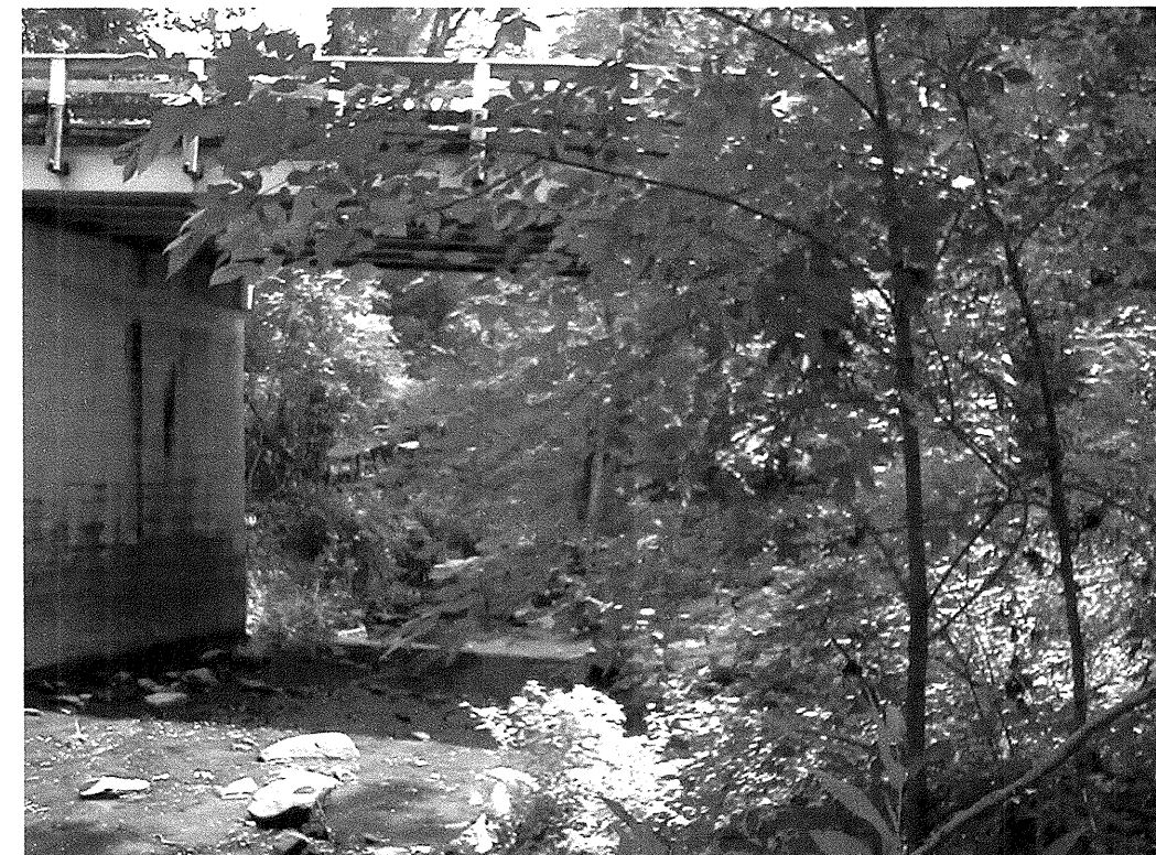
Photograph 8: View of Existing Bridge No. 174 Over Cane Creek From Down-Stream
