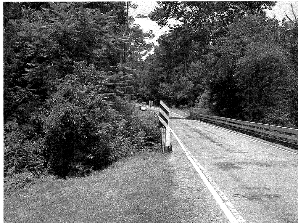
Photograph 6: View of Left Profile Looking Up-Station (From End Bent 1)
