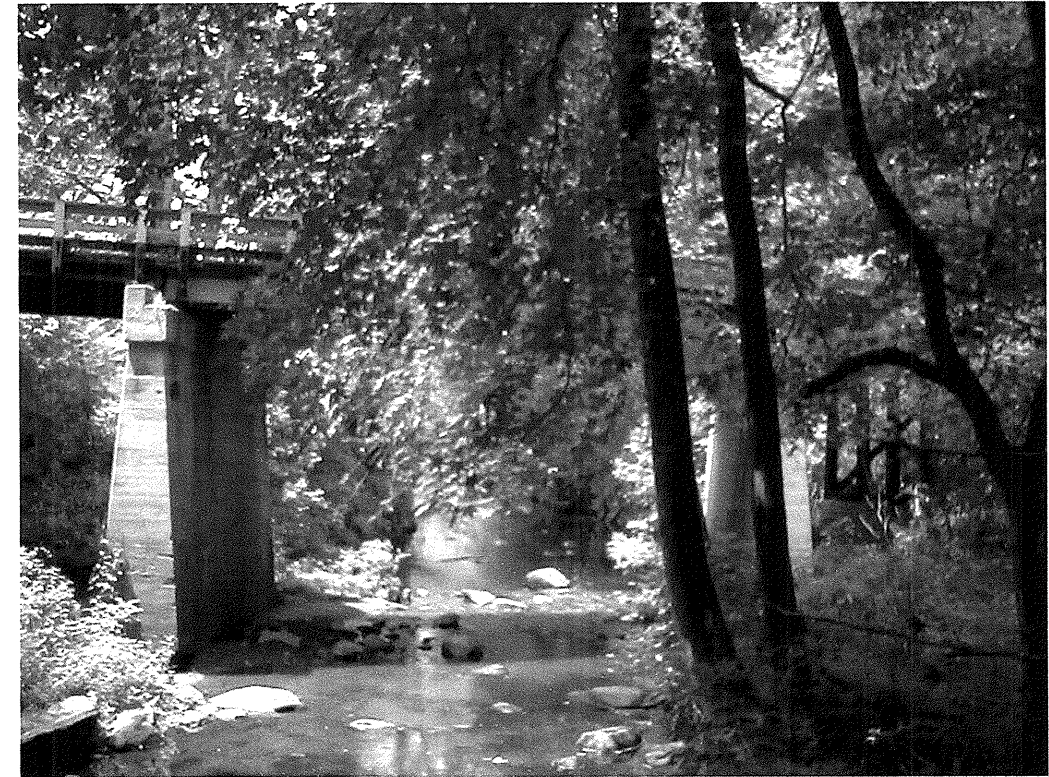
Photograph 7: View of Existing Bridge No. 174 Over Cane Creek From Up-Stream
