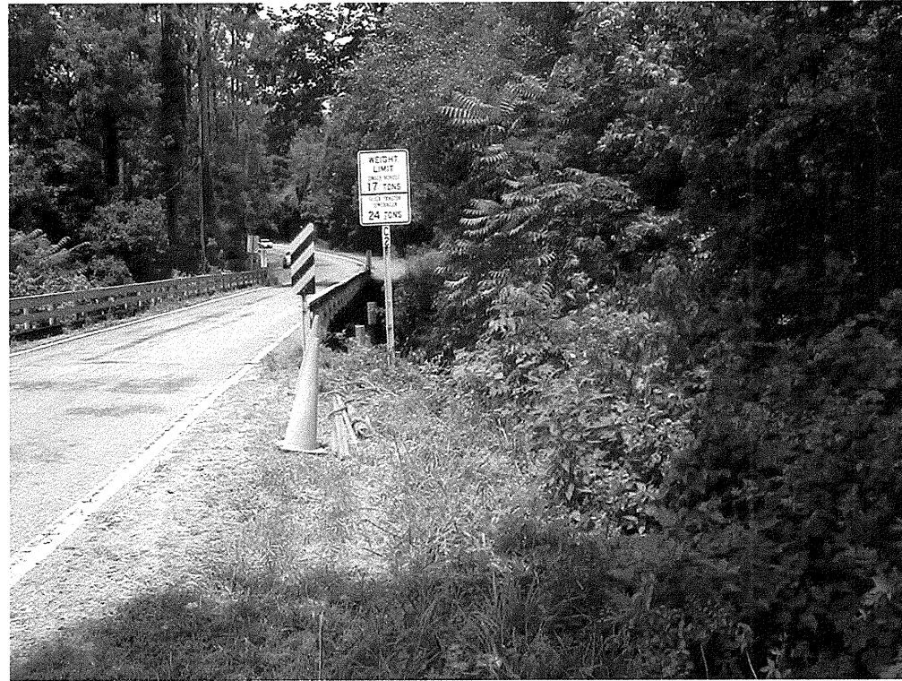
Photograph 5: View of Right Profile Looking Up-Station (From End Bent 1)
