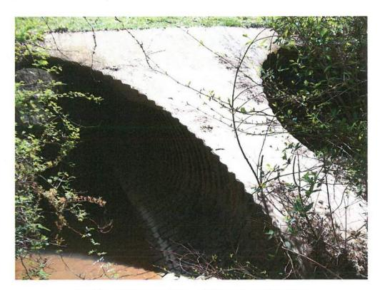
Looking at Upstream Face of Downstream Structure (2 @ 9.5' x 6.75' CMPA)
