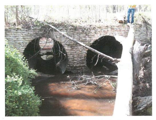
Looking at Upstream Face of Downstream Structure (2 @ 92" CMP)
