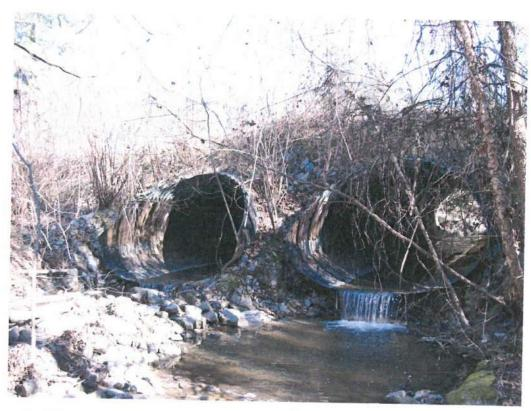
Looking at Downstream Face of Downstream Structure (2@ 9.5'x6.4' CMPA)
