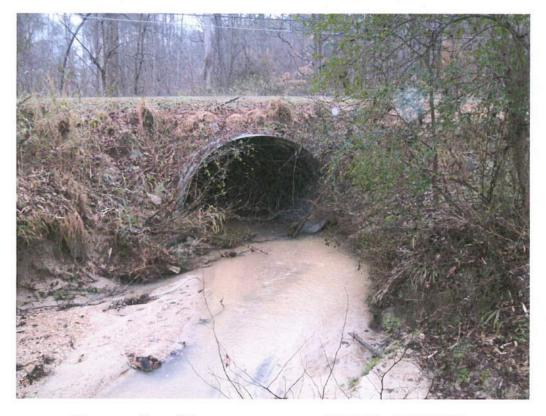
Upstream face of downstream structure 1@ 9'-6" x 6'-5" CMPA.
