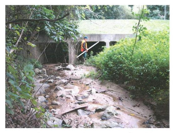
Looking at Downstream Face of Upstream Structure. (3@7'x5' RCBC)
