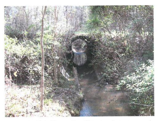
Looking at Upstream Face of Downstream Structure (1@84" CMP)
