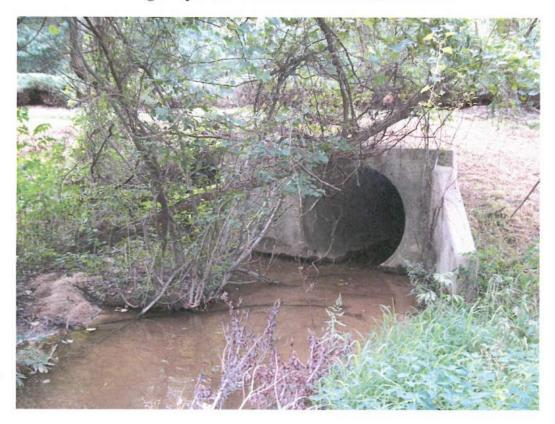
Looking at Upstream Face of Downstream Structure (2@60"RCP)
