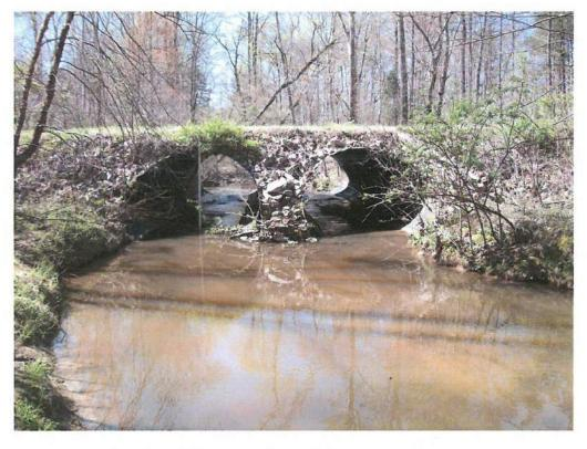
Looking at Upstream Face of Downstream Structure. (2 @ 10'x7'CSPA)
