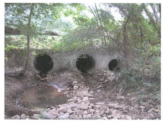
Looking at Downstream Face of Downstream Structure. (2@60"RCP with 42"RCP from Roadway)
