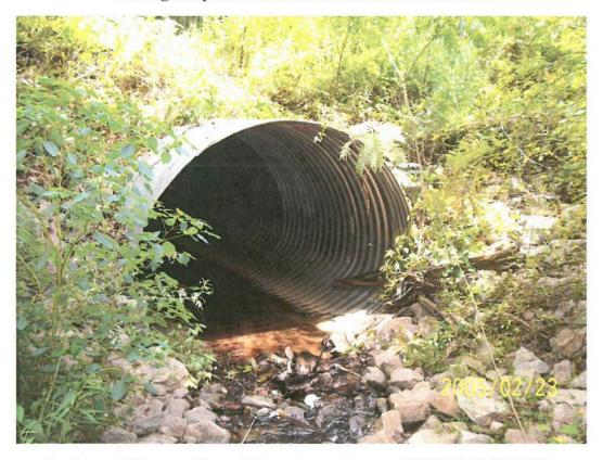
Looking at Upstream Face of Downstream Structure 1@11'-5"x7'-3" CMPA
