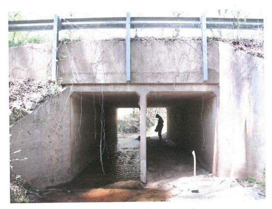
Looking at Upstream Face of Downstream Structure (2 @ 6' x 8' RCBC)
