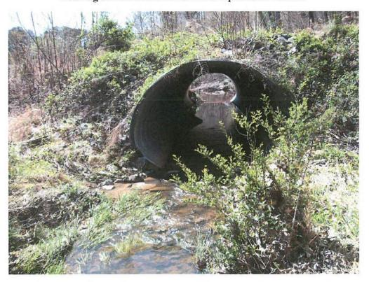
Looking at Upstream Face of Downstream Structure (1 @ 120"x84" CSPA)
