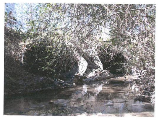
Looking at Upstream Face of Downstream Structure (2@ 9.5'x6.4' CMPA)
