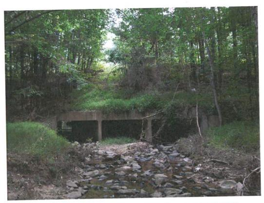
Looking at Downstream Face of Upstream Structure 3@9'x5' RCBC
