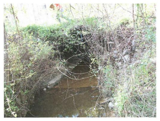
Looking at Upstream Face of Downstream Structure (1 @  $10.5^{\circ}$  x  $7.25^{\circ}$  CMPA)
