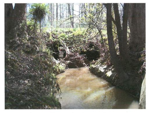
Looking at Upstream Face of Upstream Structure (2 @ 6.5' CMP)
