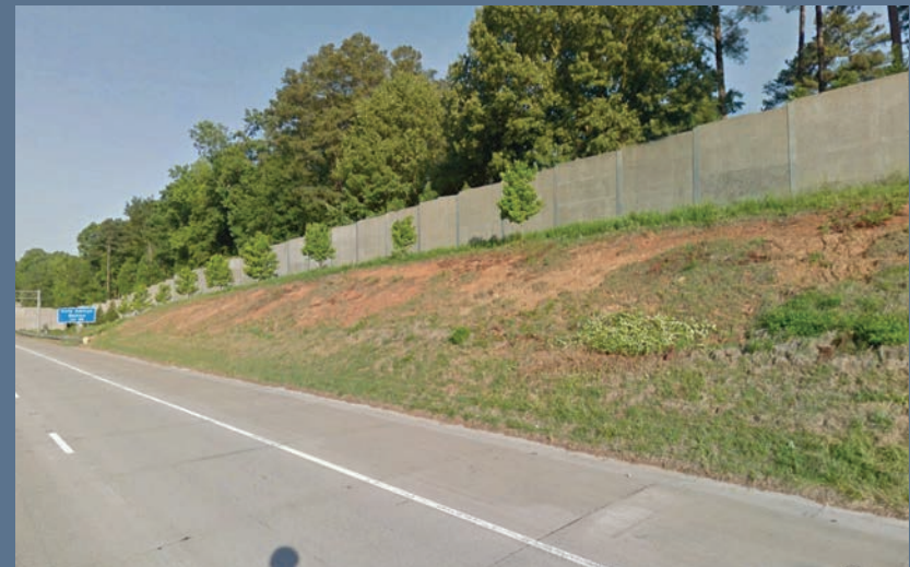
An important part of the noise analysis conducted for projects such as Complete 540 is determining locations where noise walls would be warranted.
