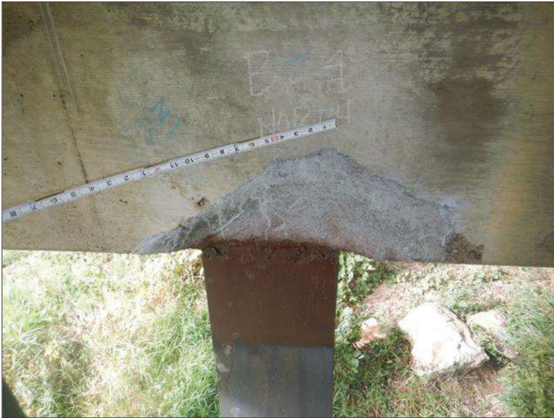
Bent 4 Cap 1: NEW REPAIR: NORTH FACE AT PILE 3, SPALL, (28 INCHES LONG X 9.5 INCHES HIGH X UP TO 3.5 INCHES DEEP) WITH EXPOSED RUSTED REINFORCING, NO LOSS NOTED-PATCHED SINCE PREVIOUS INSPECTION 2023
