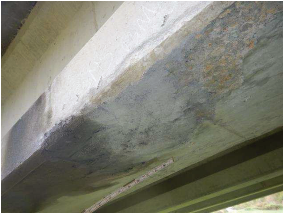
Span 5 Beam 1: NEW REPAIR: UNDERSIDE BOTTOM FLANGE AT 14 FEET FROM BENT 4, SPALL (20 INCHES LONG X 14 INCHES WIDE X UP TO 1.5 INCH DEEP) WITH MULTIPLE EXPOSED PRESTRESS STRANDS, LOSS UP TO 100 PERCENT ON INDIVIDUAL STRANDS-PATCHED SINCE PREVIOUS INSPECTION 2023
