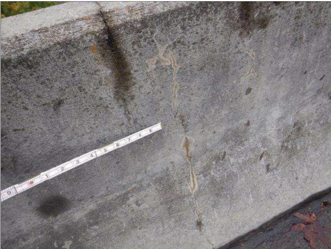
Span 2 Left Bridge Rail: ALONG LENGTH AT MULTIPLE LOCATIONS, VERTICAL CRACKS (UP TO FULL HEIGHT X UP TO 1/32 INCH WIDE) SOME WRAPAROUND AND SOME EFFLORESCENCE
