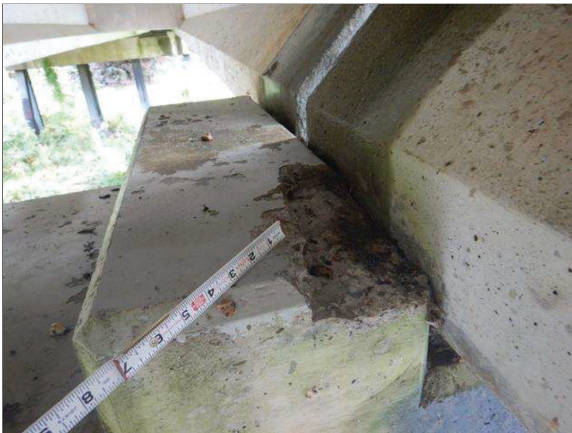
Bent 3 Cap 1: KEEPER BLOCK AT SPAN 3 BEAM 4, SPALL (UP TO 5 INCHES LONG X 8 INCHES WIDE X UP TO 2 INCHES DEEP)
