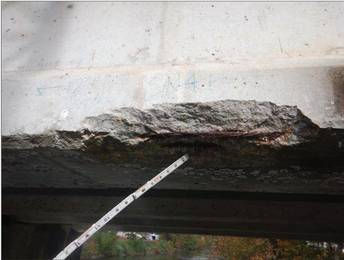
Span 4 Beam 4: (PAR) AT 12 FEET FROM BENT 3, EAST FACE OF BOTTOM FLANGE, SPALL (26 INCHES LONG X 7 INCHES WIDE X UP TO 4 INCHES DEEP) WITH TWO (2) EXPOSED AND RUSTED PRESTRESSED STRANDS (80 PERCENT REMAINING)
