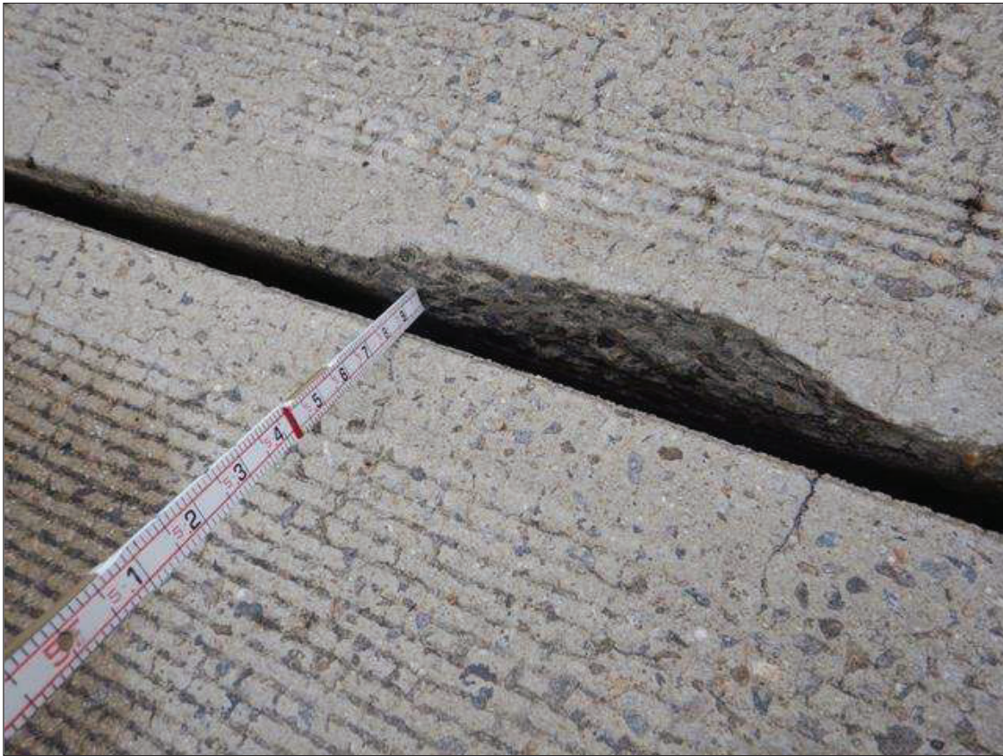
Span 3 Expansion Joint: NEAR CENTERLINE AT BENT 2 JOINT ON SPAN 2 SIDE, SPALL (4 INCHES LONG X 12 INCHES WIDE X 2 INCHES DEEP)
