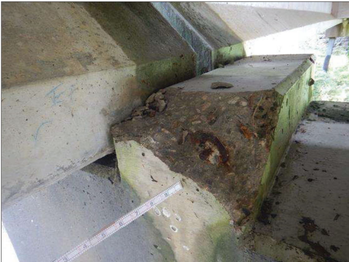
Bent 3 Cap 1: KEEPER BLOCK AT SPAN 3 BEAM 1, SPALL (12 INCHES LONG X 9 INCHES HIGH X UP TO 4 INCHES DEEP)
