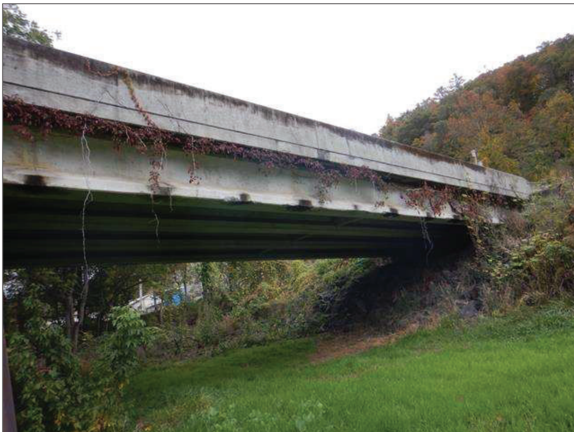
General: ALONG RIGHT OVERHANG AT SPANS 4 AND 5, VEGETATION GROWTH
