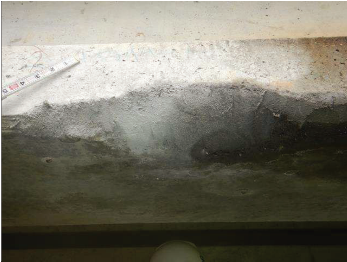
Span 4 Beam 4: NEW REPAIR: EAST FACE BOTTOM FLANGE 15 FEET SOUTH OF BENT 4, SPALL (26 INCHES LONG X 5 INCHES WIDE X UP TO 2.5 INCHES DEEP) WITH ONE EXPOSED PRESTRESSED STRANDS WITH LOSS UP TO 100 PERCENT ON MULTIPLE INDIVIDUAL STRANDS-PATCHED SINCE PREVIOUS INSPECTION 2023
