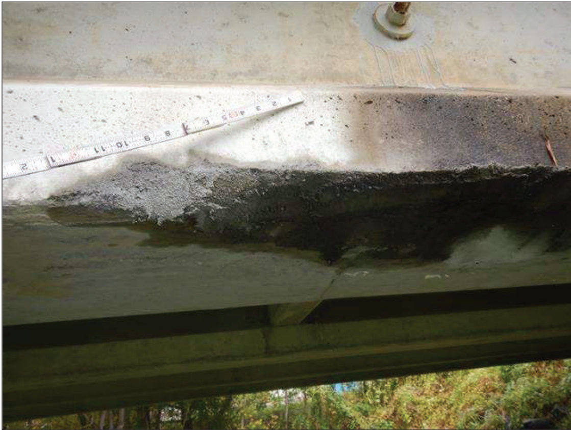
Span 5 Beam 4: NEW REPAIRS: UNDERSIDE OF BOTTOM FLANGE AT 12 FEET (FOR 40 INCHES), AT 17 FEET (FOR 61 INCHES), AT 23 FEET (FOR 54 INCHES), AT 30 FEET (FOR 35 INCHES), AT 41 FEET (FOR 34 INCHES) FROM BENT 4, SPALLS (UP TO 14 INCHES X UP TO 2.75 INCHES DEEP) WITH MULTIPLE EXPOSED PRESTRESSED STRANDS, LOSS UP TO 100 PERCENT ON INDIVIDUAL STRANDS-ALL SPALLS HAVE BEEN PATCHED SINCE PREVIOUS INSPECTION 2023
