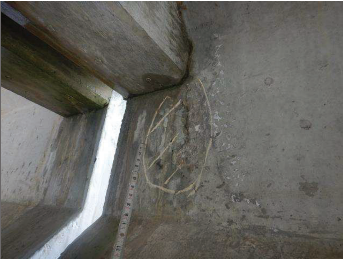
Span 2 Beam 4: WEST FACE OF WEB AT BENT 2, SPALL (4 INCHES LONG X 10 INCHES HIGH X 1 INCH DEEP) WITH ADJACENT DELAMINATION (10 INCHES LONG X 12 INCHES HIGH)
