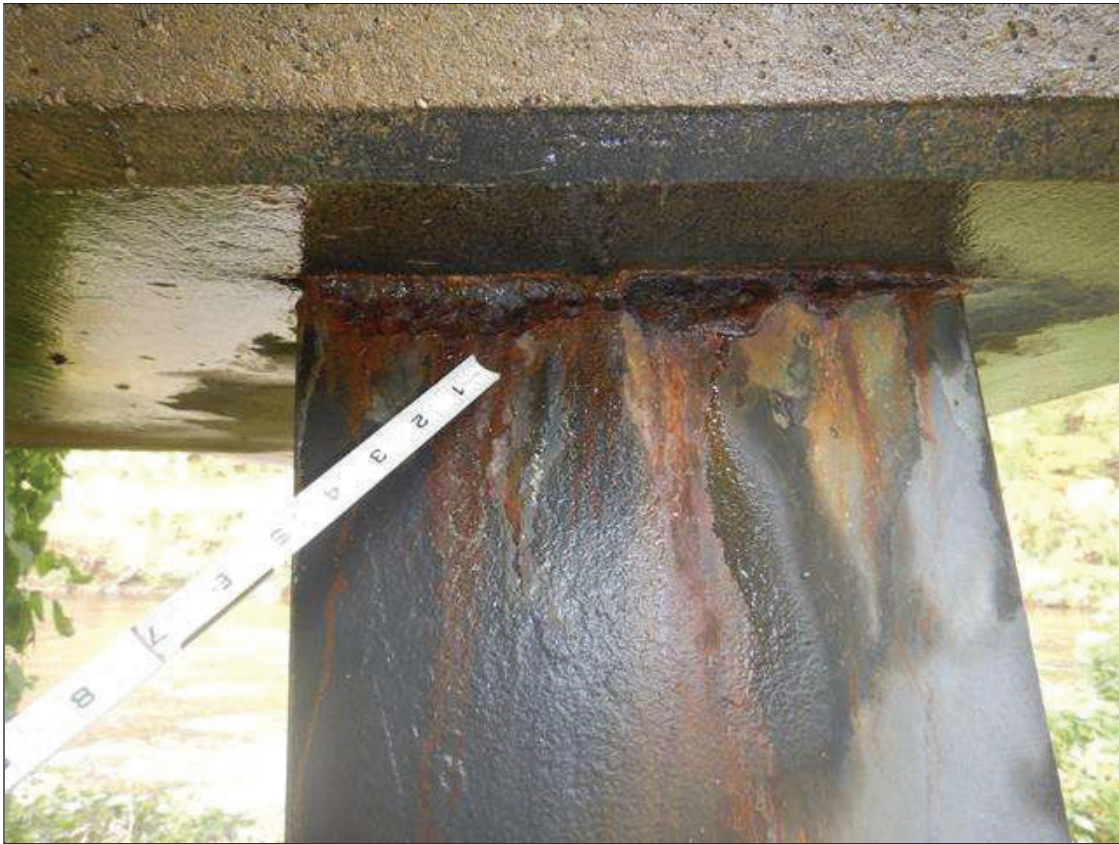
Bent 4 Row 2 Pile 1: (PAR) NORTH FACE AT CAP, ACTIVE CORROSION WITH SECTION LOSS (FULL WIDTH X 1 INCH HIGH X 0.3125 INCH AVERAGE REMAINING)
