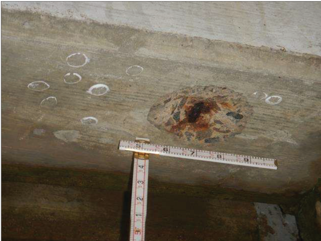
Span 3 Beam 3: END DIAPHRAGM AT BAY 3 BENT 2, SPALL WITH EXPOSED REBAR (4 INCH DIAMETER X 1/2 INCH DEEP) WITH EXPOSED REBAR (90 PERCENT REMAINING)
