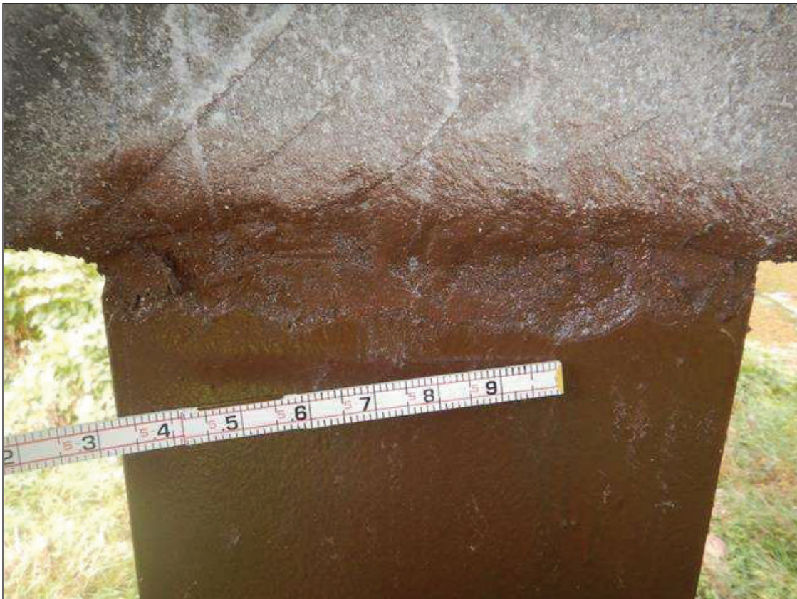
Bent 4 Row 2 Pile 3: (PAR) TOP NORTH FACE AT CAP, ARRESTED CORROSION WITH SECTION LOSS (FULL WIDTH X UP TO 2 INCHES HIGH X 0.25 INCH AVERAGE REMAINING)
