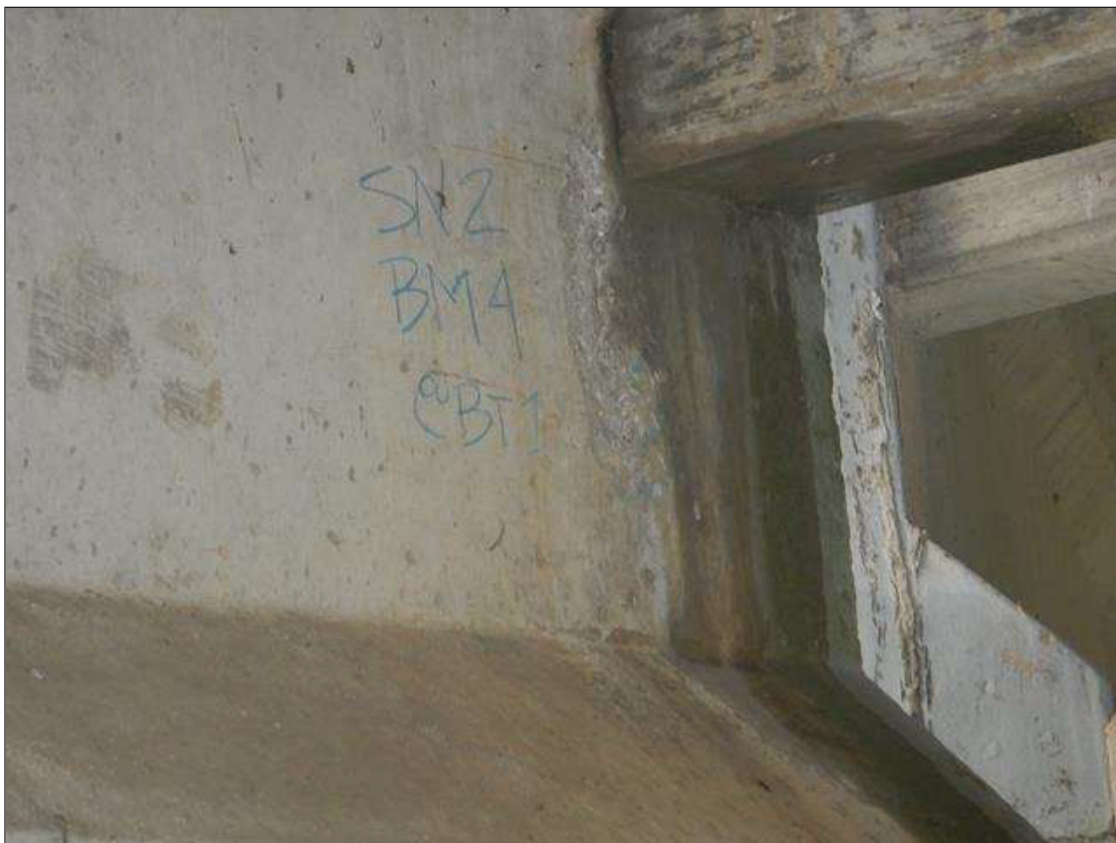
Span 2 Beam 4: WEST FACE OF WEB AT BENT 1, SPALL (11 INCHES LONG X 3 INCHES HIGH X 3/4 INCH DEEP) WITH ADJACENT DELAMINATION (11 INCHES LONG X 4 INCHES HIGH)
