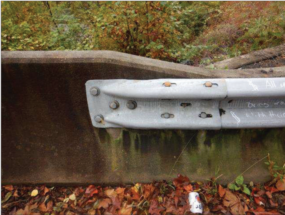
TYPICAL GUARDRAIL TO BRIDGE RAIL CONNECTION
