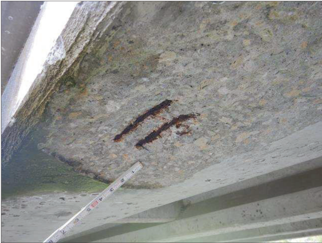
Span 4 Beam 1: (PAR) AT 24 FEET FROM BENT 3, UNDERSIDE OF BOTTOM FLANGE, SPALL (20 INCHES LONG X UP TO 18 INCHES WIDE X UP TO 1 INCH DEEP) WITH TWO (2) EXPOSED AND RUSTED PRESTRESSED STRANDS (75 PERCENT REMAINING)
