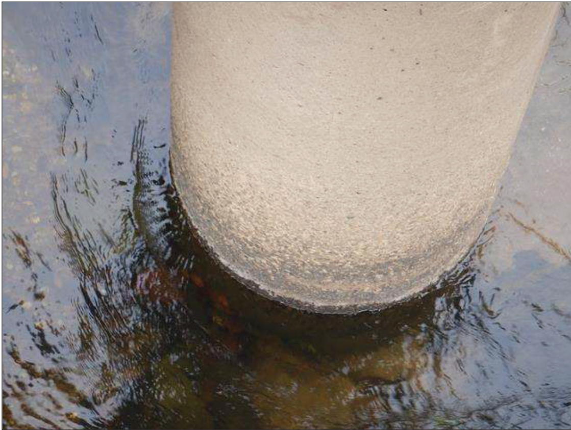
Bent 2 Pile 1: AT BASE OF COLUMN, ABRASION WITH EXPOSED AGGREGATE
