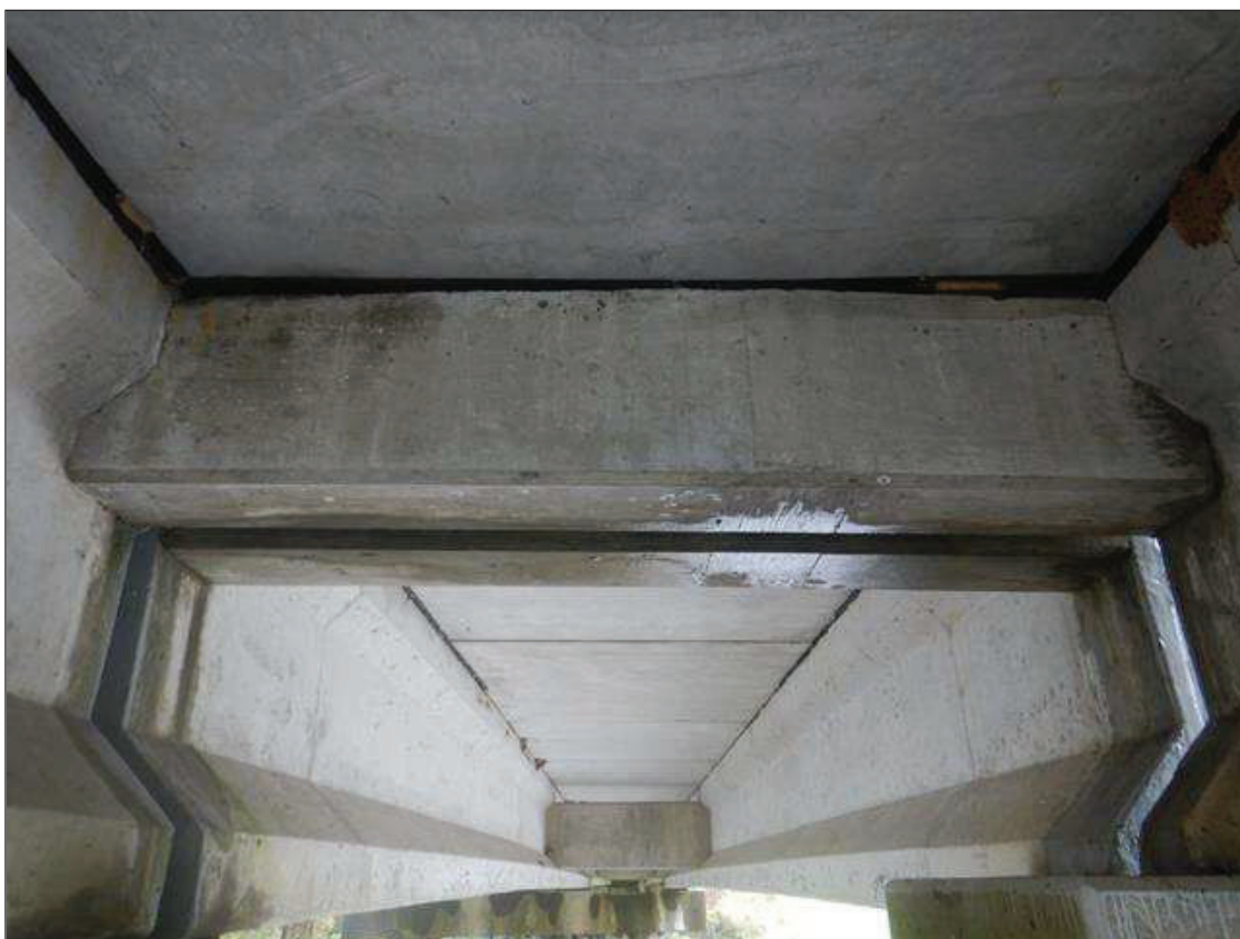
TYPICAL END DIAPHRAGM
