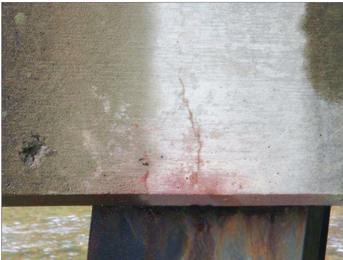
Bent 4 Cap 1: NORTH FACE OVER PILE 4, VERTICAL CRACK (6 INCHES HIGH X UP TO 1/32 INCH WIDE)
