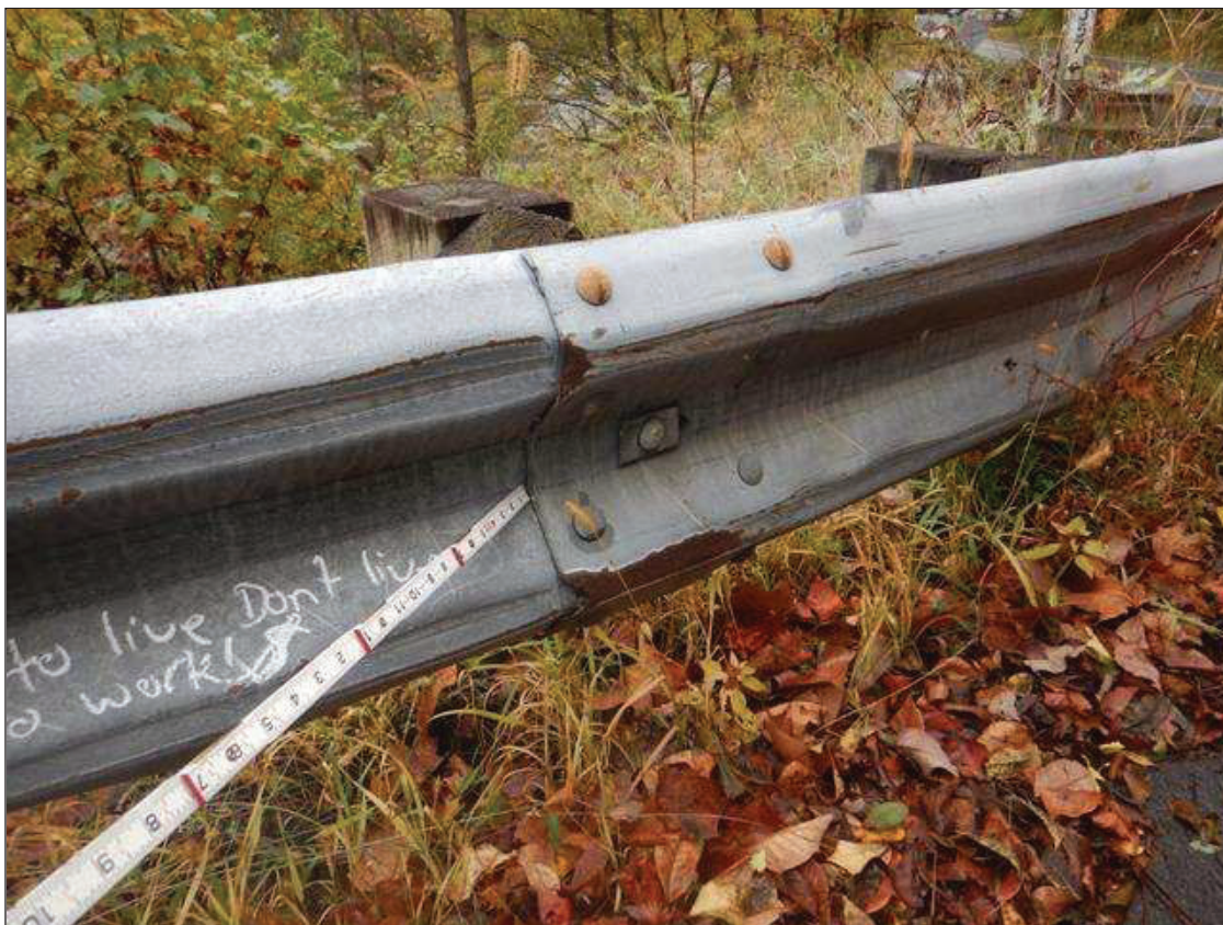
Guardrails: SOUTHEAST GUARDRAIL NEAR SOUTH APPROACH, SCRAPE MARKS (10 FEET LONG)
