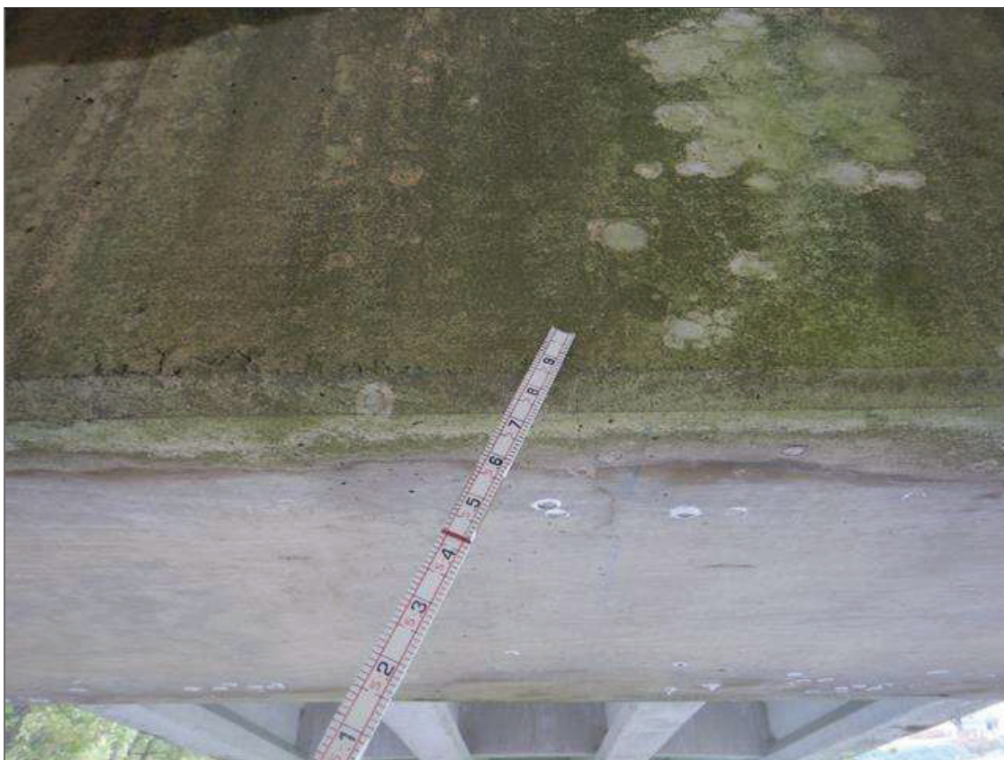
Bent 3 Cap 1: UNDERSIDE BETWEEN COLUMNS, MULTIPLE TRANSVERSE CRACKS (8 INCHES LONG X HAIRLINE) SOME EXTEND UP TO VERTICAL FACE
