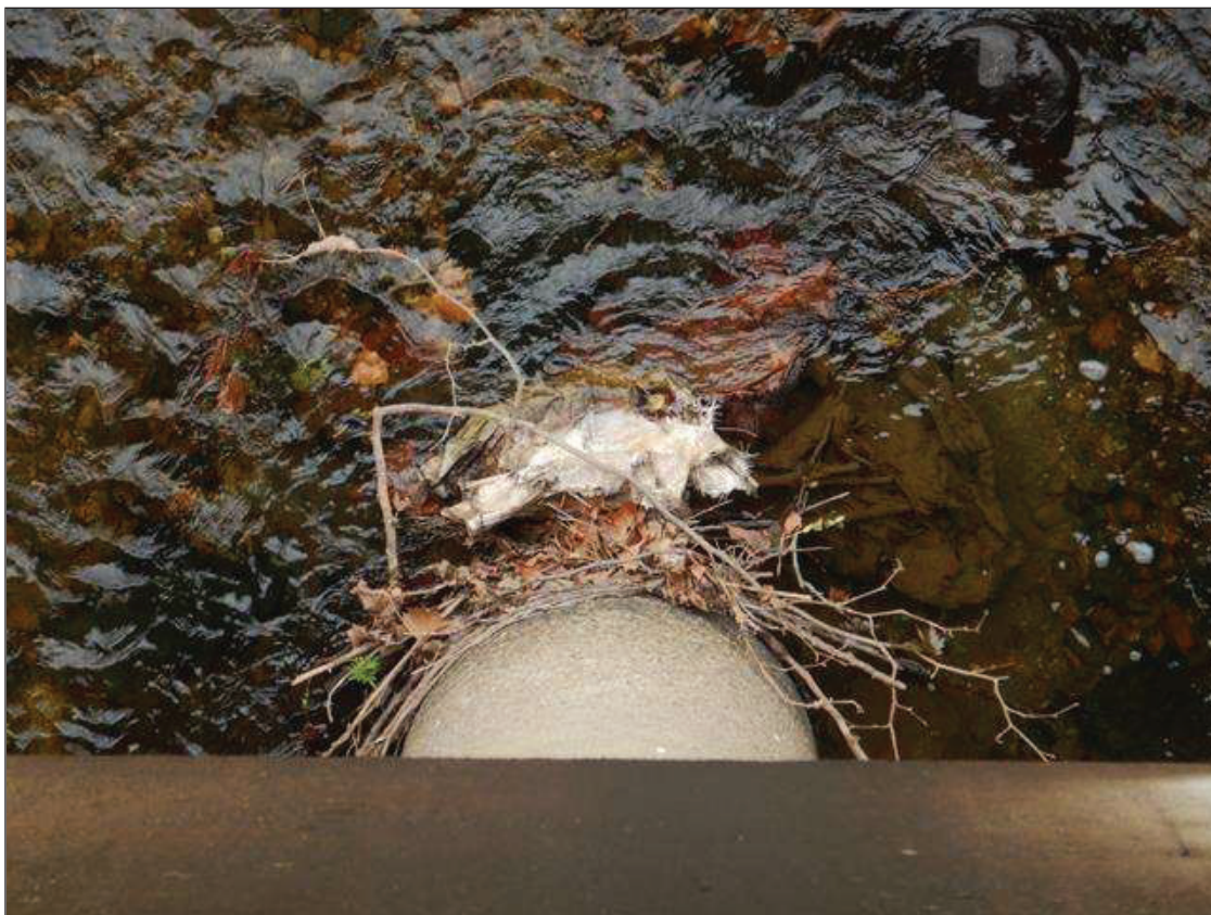
Drift: AT SOUTHEAST FACE OF BENT 3, DRIFT ACCUMULATION (2 FEET LONG X 4 FEET WIDE X UP TO 1 FOOT HIGH)
