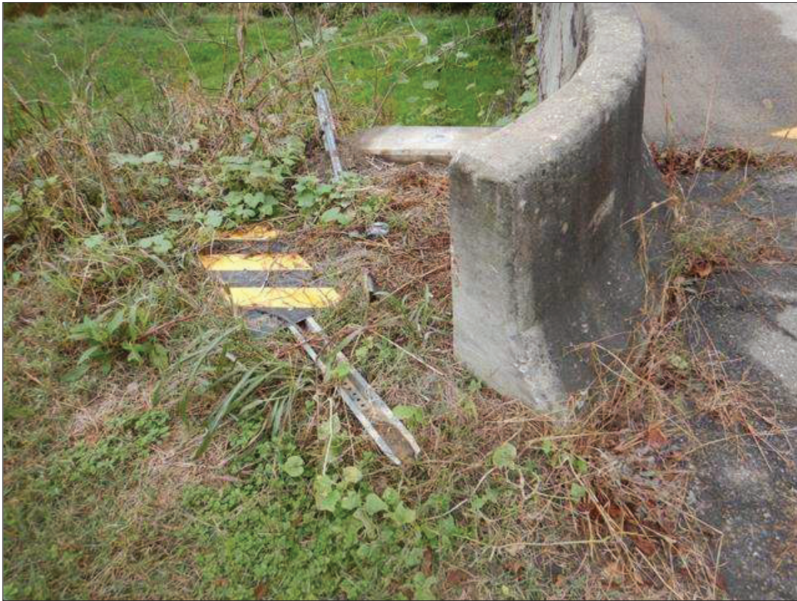
Span 5 Northeast Delineator: (PAR) NORTHEAST DELINEATOR IS LAYING ON GROUND
