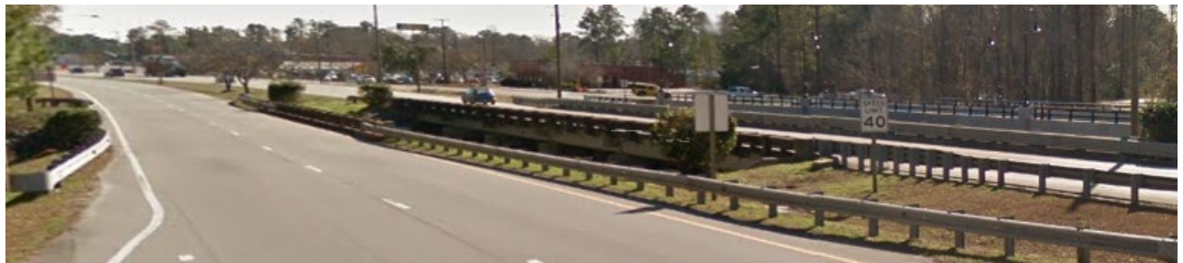
#1 Bridges 91 and 92: Google StreetView
