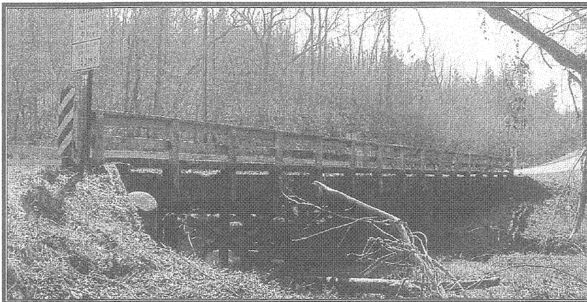
STRUCTURE PROFILE UPSTREAM
