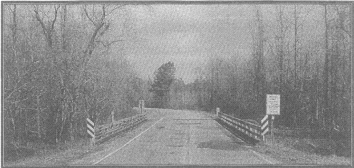
LOOKING NORTH ACROSS BRIDGE
