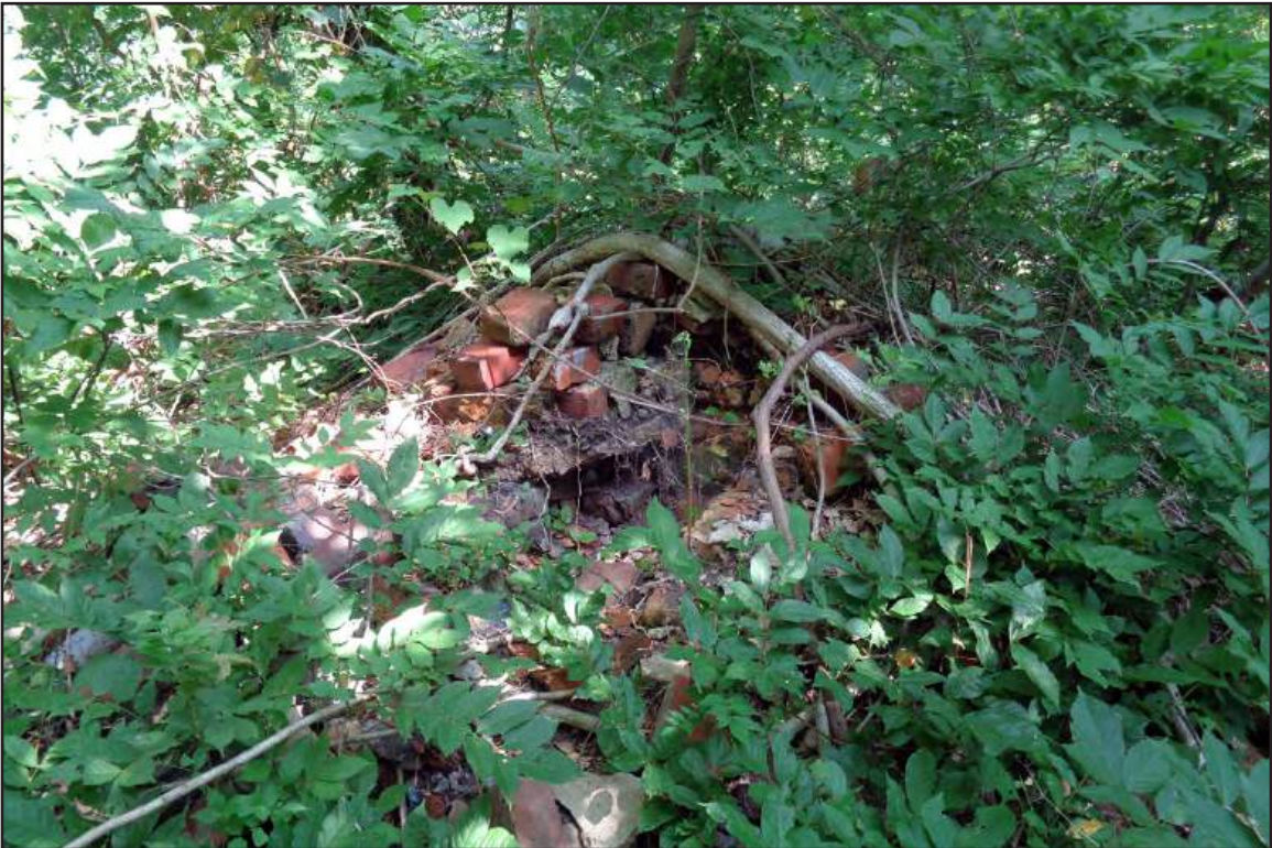
PLATE 4: View of Brick Chimney Remains, Site 31GS376, View to North
