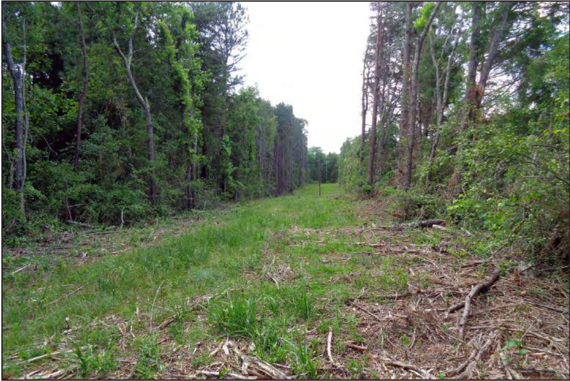
PLATE 13: Utility Right-of-Way in Section 3, View to West
