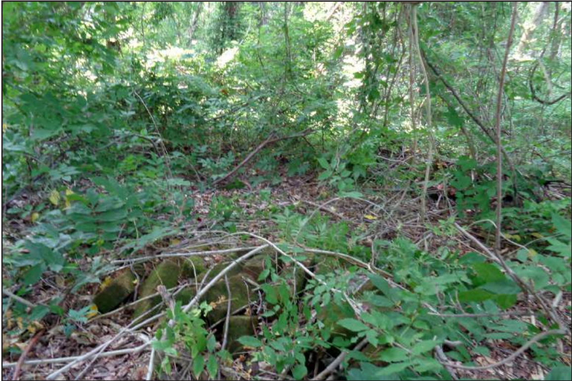
PLATE 5: View of Brick Pier and Cellar Depression, Site 31GS376, View to East
