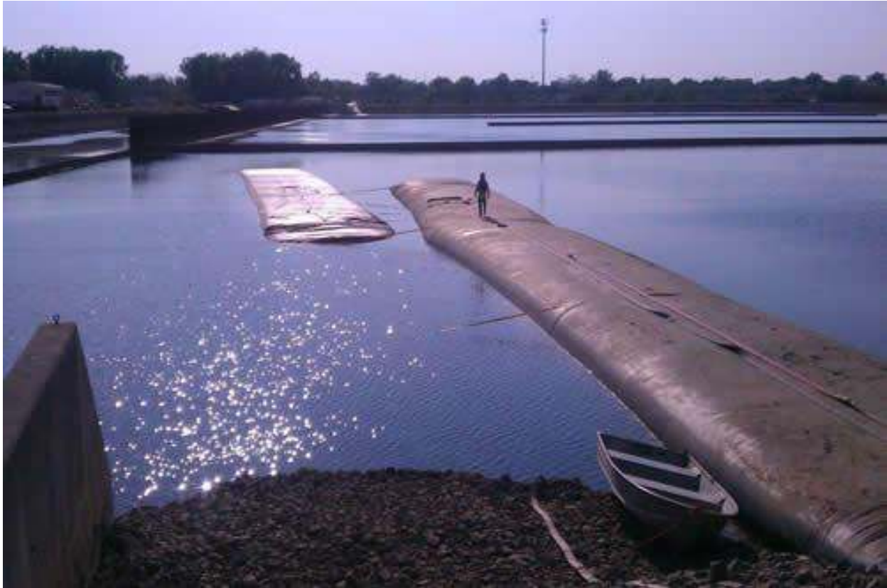
Figure 27 – An additional cofferdam is being prepared for coupling.
