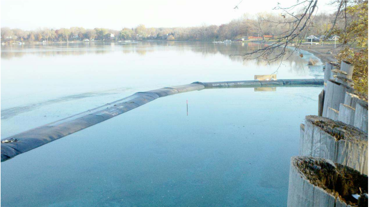
Figure 9 – A long cofferdam with coupling collar connections.
