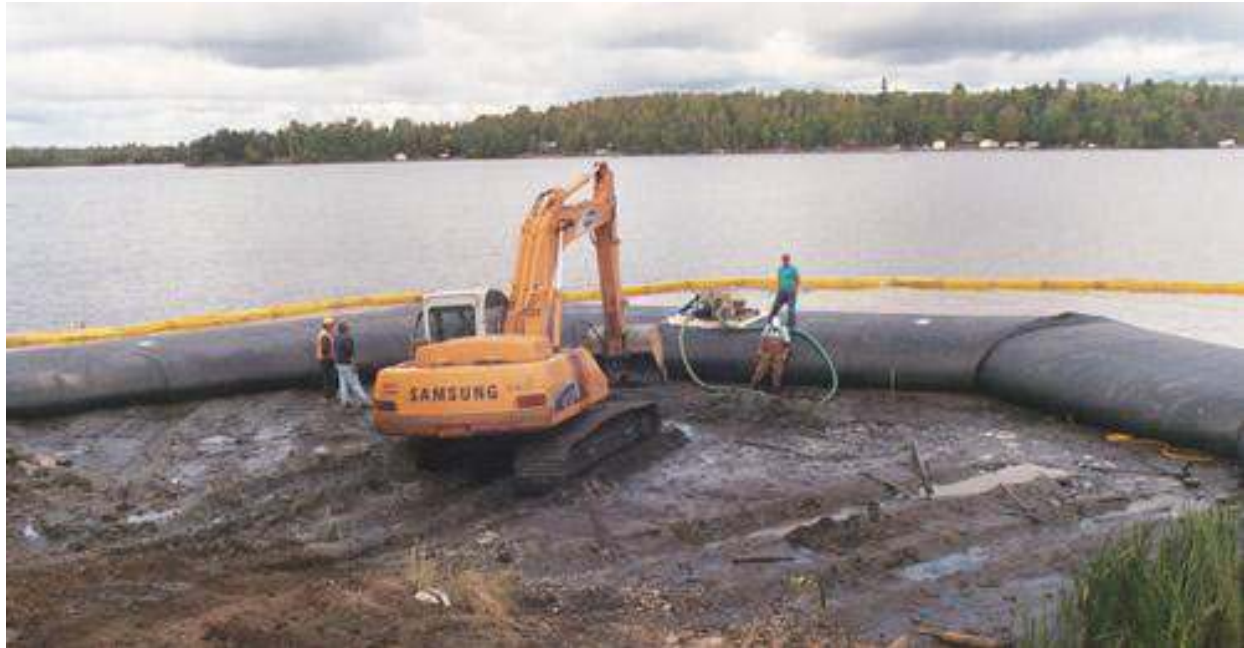
Figure 6 – A cofferdam holding back water so work can proceed.
