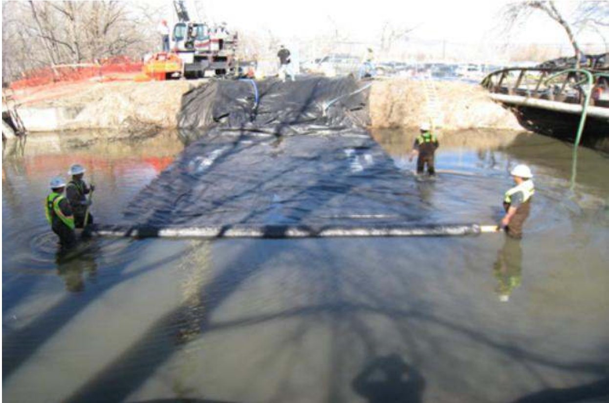
Figure 2 – Workers unroll a cofferdam in preparation for inflation.
