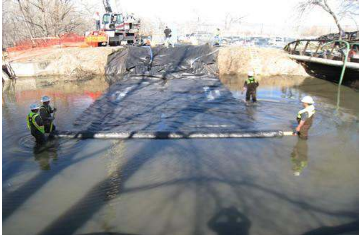
Figure 18 – Workers work in unison as the cofferdam inflates and unrolls.
