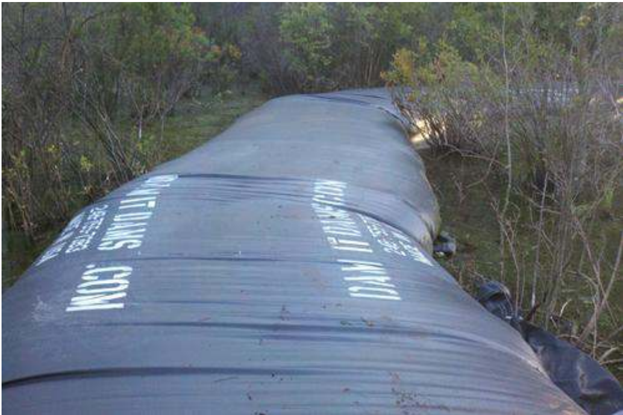
Figure 25 – A fully inflated large cofferdam.
