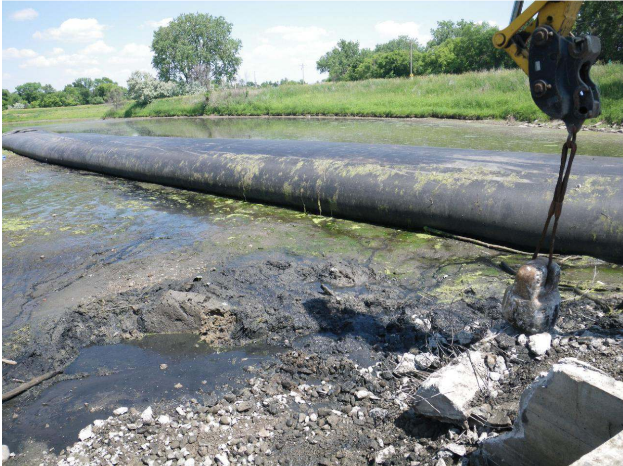
Figure 19 – A fully inflated cofferdam.
