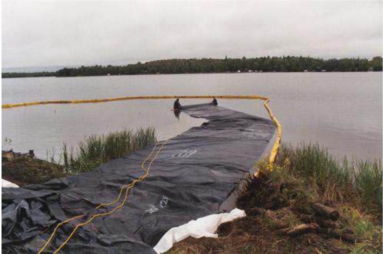
Figure 22 – A large cofferdam properly positioned at the Starting Point.
