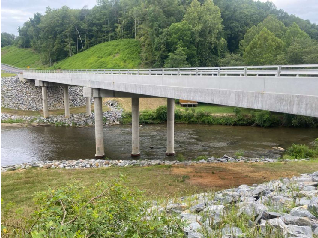
Rip rap free benches under Stokes 8 on NC 742 over Dan River.
