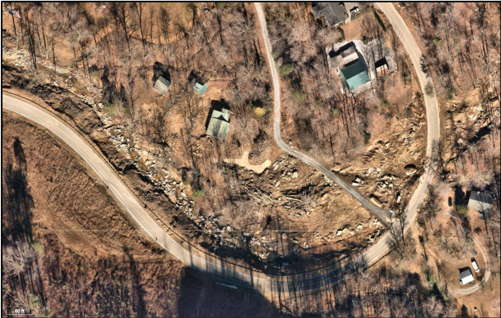
Figure 3. Detail from aerial imagery showing the nature and scale of the altered landscape after the Helene floods along a bend on NC 9 at the crossing of Grassy Creek (image extracted from Nearmap, image date January 25, 2025). Note the heavy erosion, shift of the creek banks, and alluvium deposits which swept and redeposited massive amounts of soil, large boulders, and other debris.
