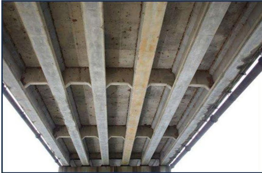
**Halifax County Bridge No. 51 (HX2158).** Detail of typical prestressed concrete span, underside of superstructure (above) and looking N from Halifax County (below).
