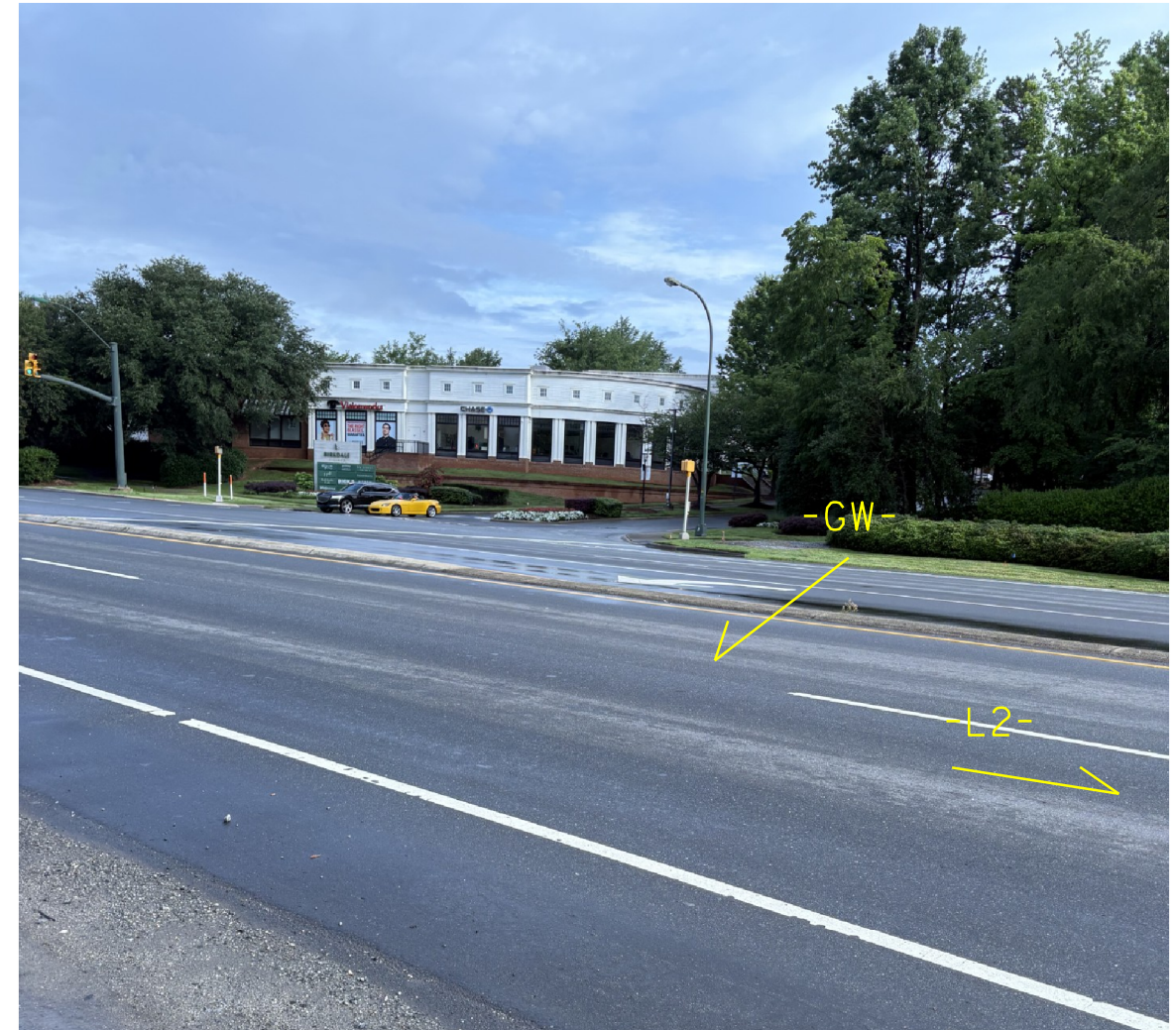
PHOTO #2: LOOKING NORTHWEST FROM BENT #6.
