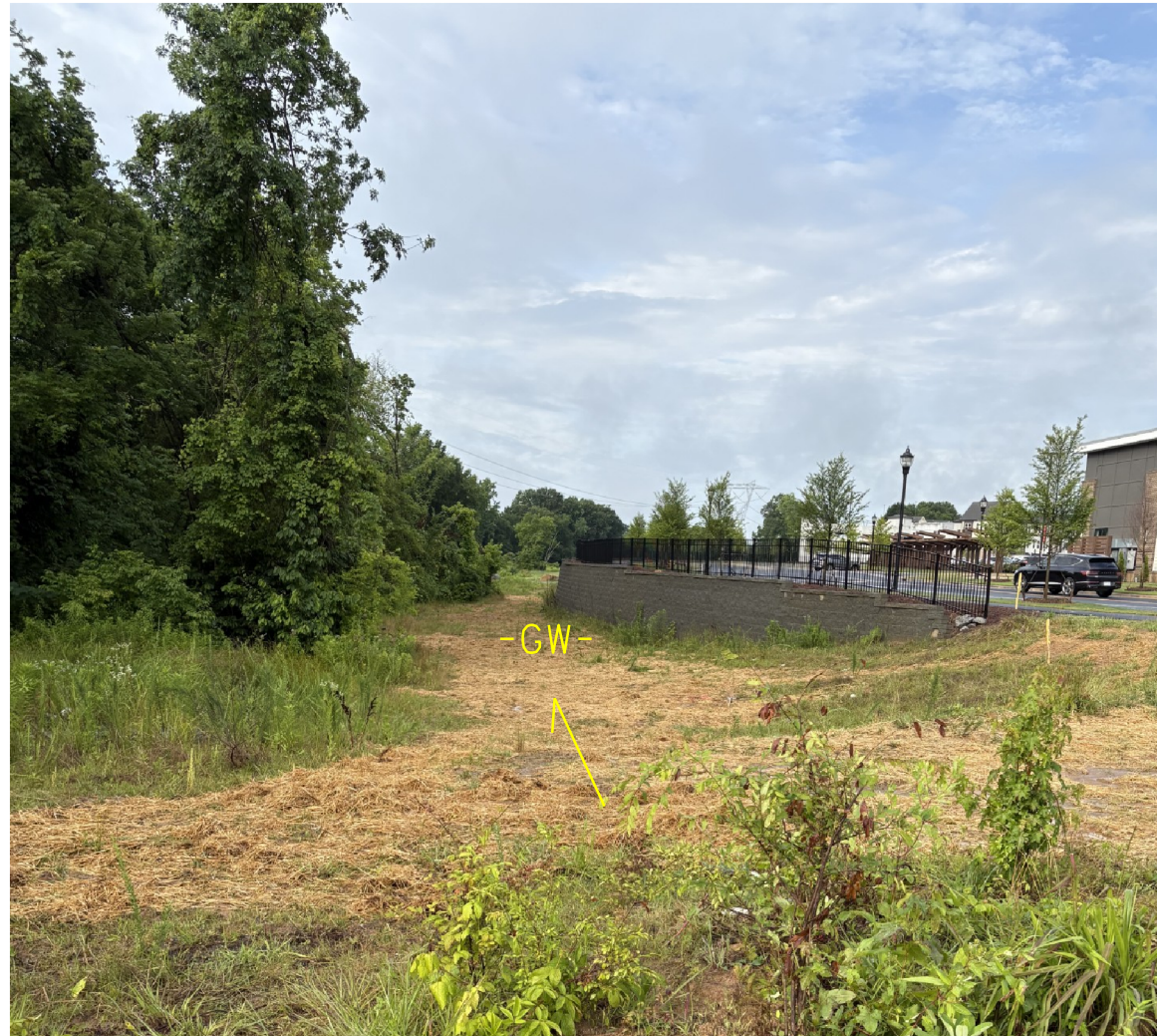
PHOTO #1: VIEW ALONG -GW- ALIGNMENT, FACING SOUTH FROM BENT #9.
