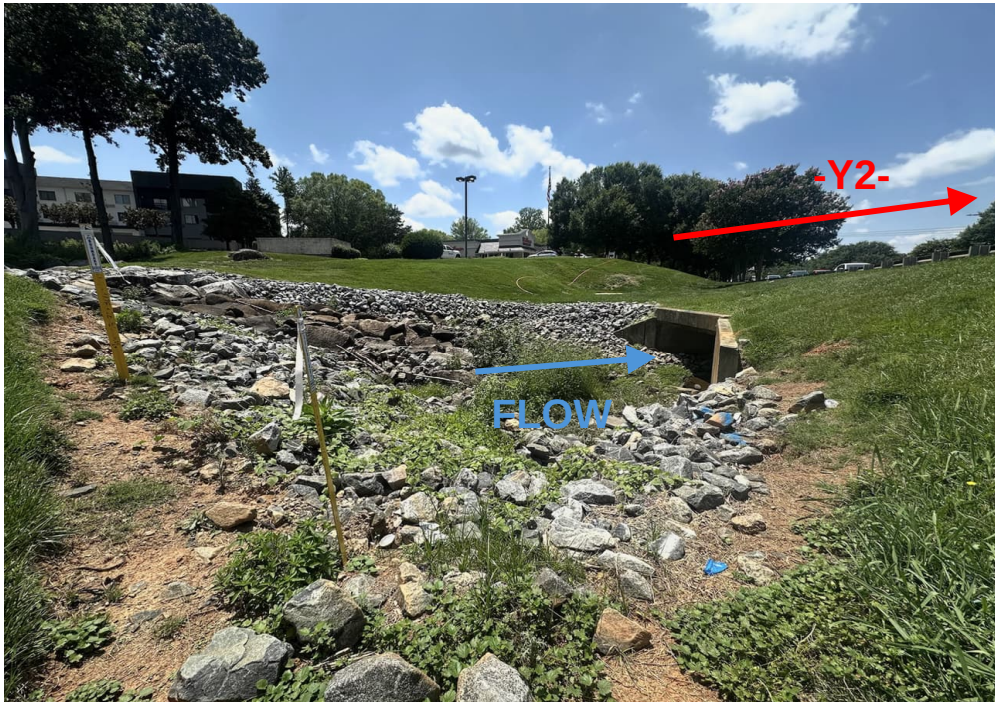
VIEW FROM EAST OF CULVERT OUTLET LOOKING NORTHWEST
