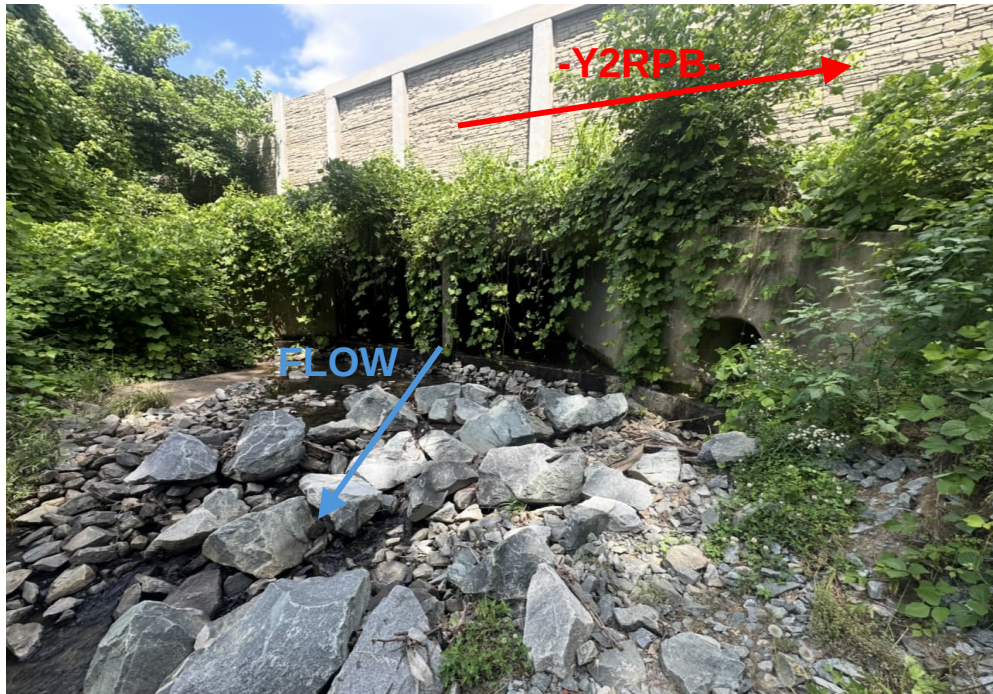
VIEW FROM SOUTH OF CULVERT OUTLET LOOKING NORTH
