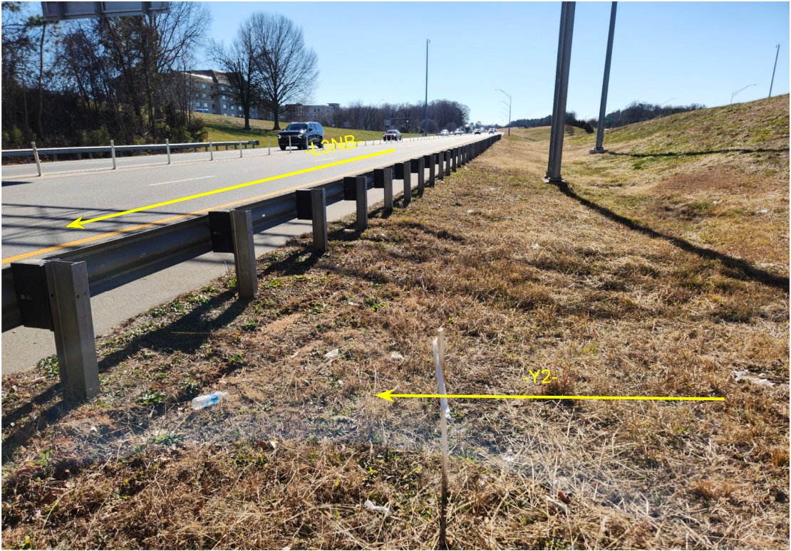
BENT NO. LOOKING SOUTH ALONG I-77 NORTHBOUND
