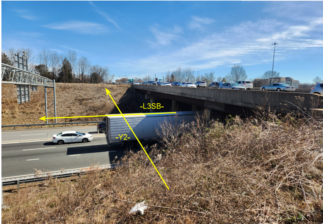
END BENT NO. 1 LOOKING EAST ALONG NORTH SIDE OF BRIDGE
