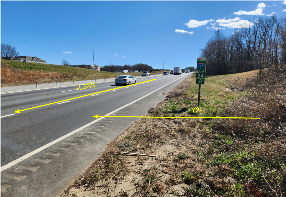
BENT NO. 1 LOOKING SOUTH ALONG I-77 SOUTHBOUND
