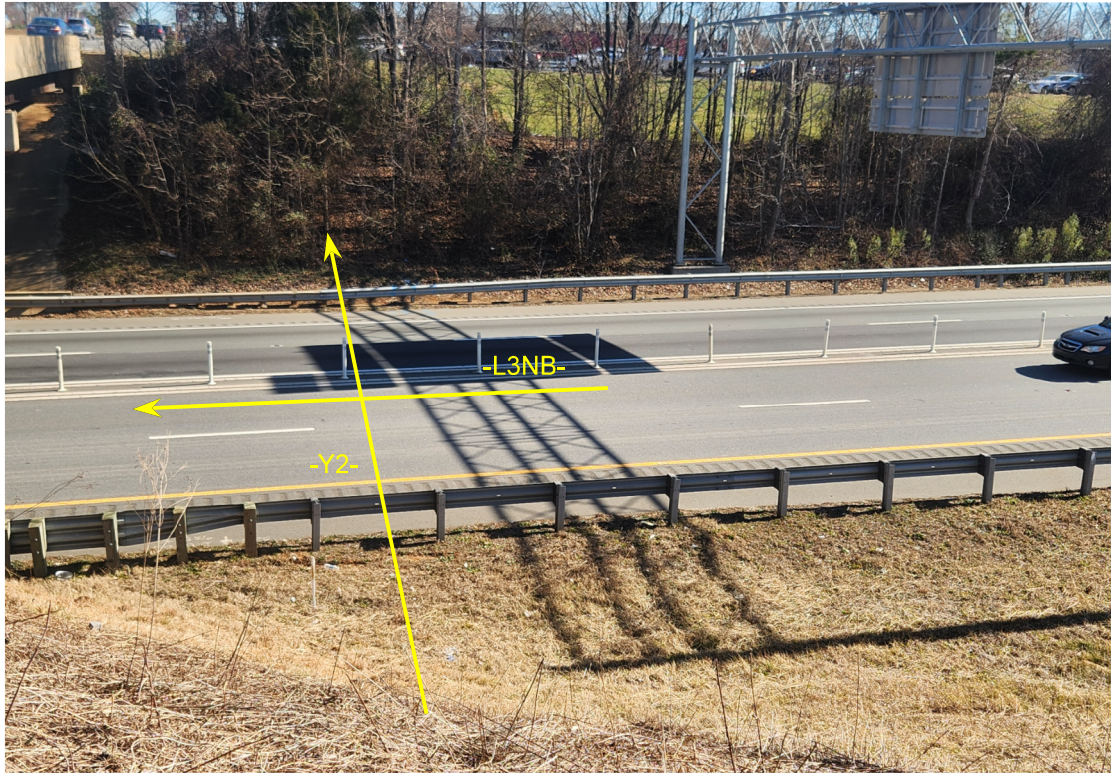
END BENT NO. 1 LOOKING EAST ALONG SOUTH SIDE OF BRIDGE
