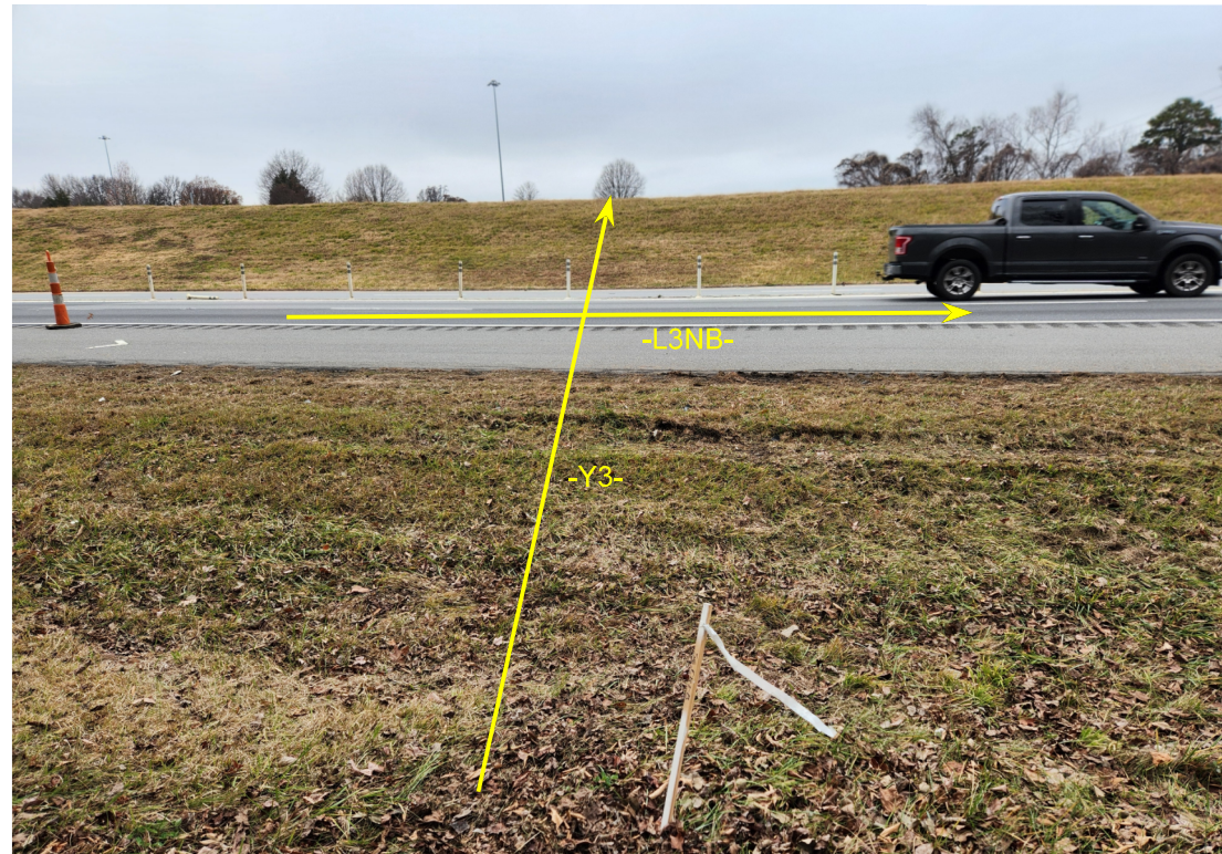
END BENT NO. 2 LOOKING WEST ALONG THE I-77 NORTHBOUND CROSSING
