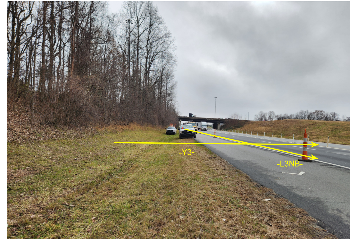
NORTH OF THE I-77 NORTHBOUND CROSSING LOOKING SOUTH
