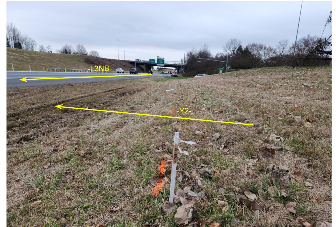
END BENT NO. 1 LOOKING SOUTH ALONG I-77 SOUTHBOUND
