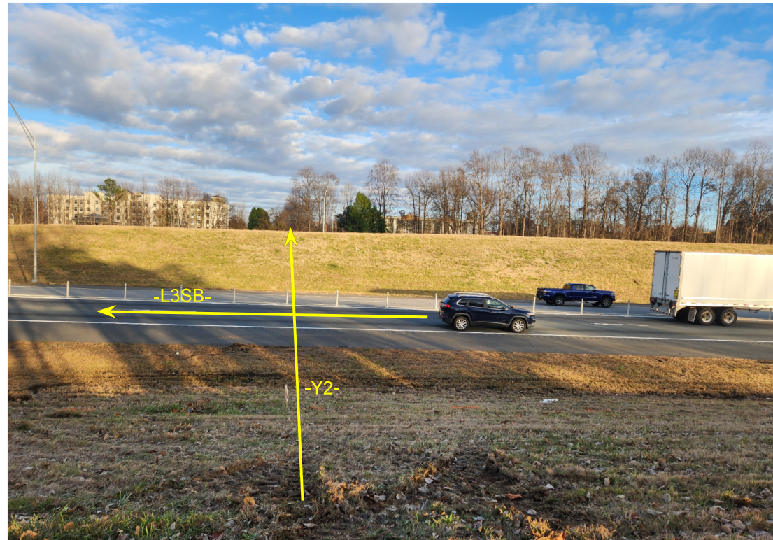
END BENT NO. 1 LOOKING WEST ALONG I-77 NORTH CROSSING
