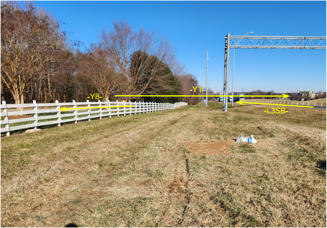
SOUTH OF BENT NO. 1 LOOKING NORTH
