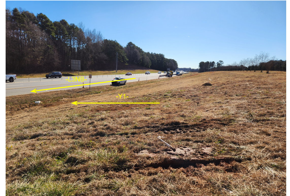
NORTHWEST OF END BENT NO. 1 LOOKING SOUTHEAST
