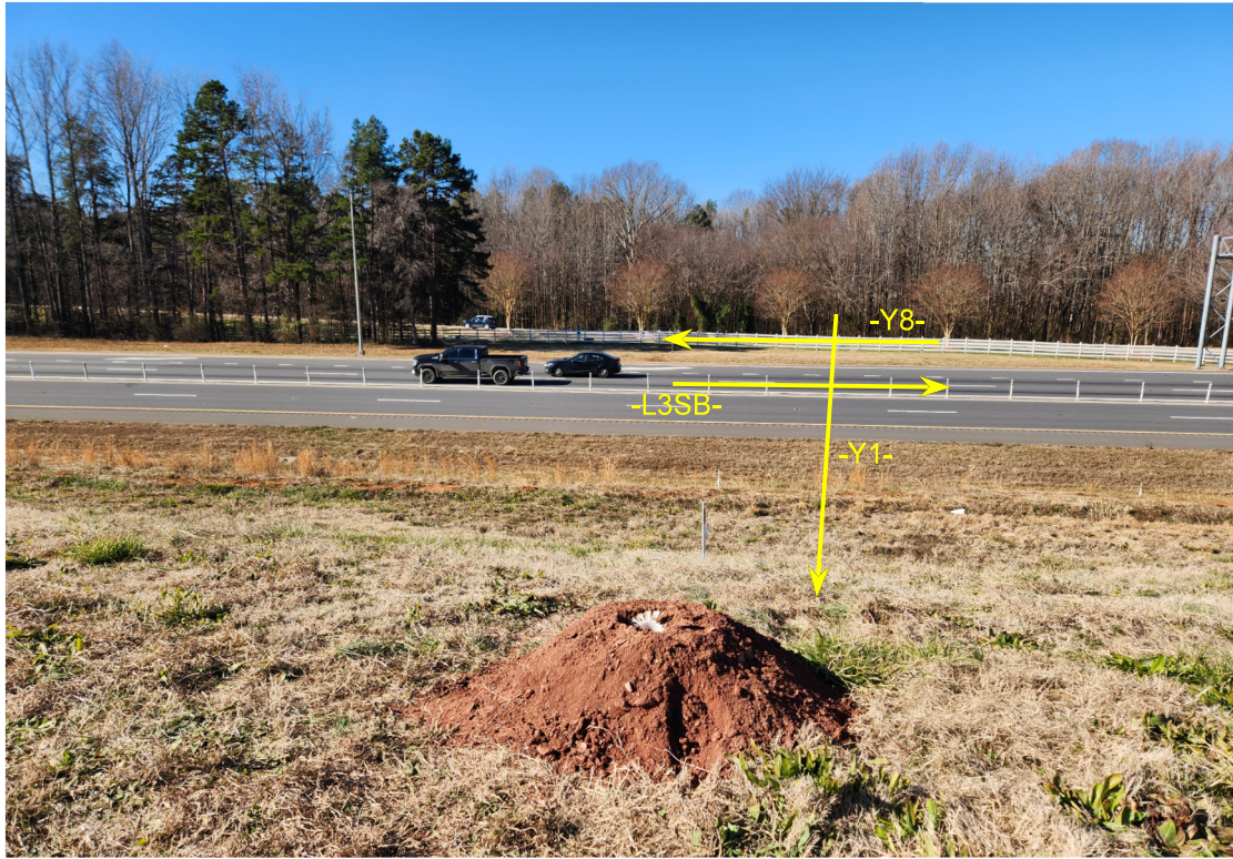
EAST OF END BENT NO. 2 LOOKING WEST
