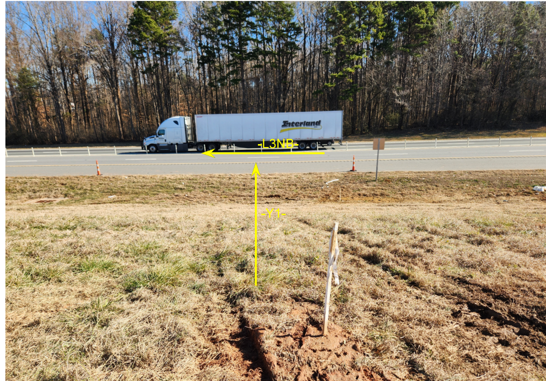
WEST OF END BENT NO. 1 LOOKING EAST
