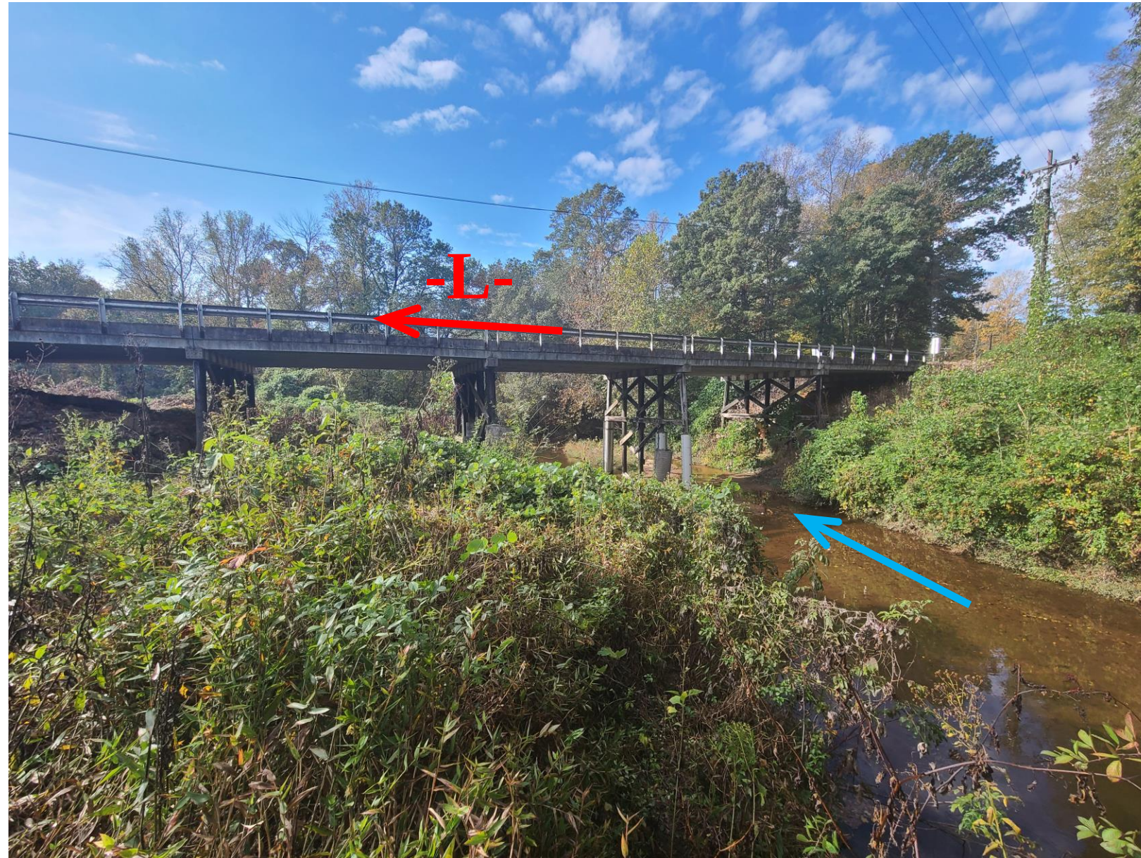
Facing South towards existing bridge
