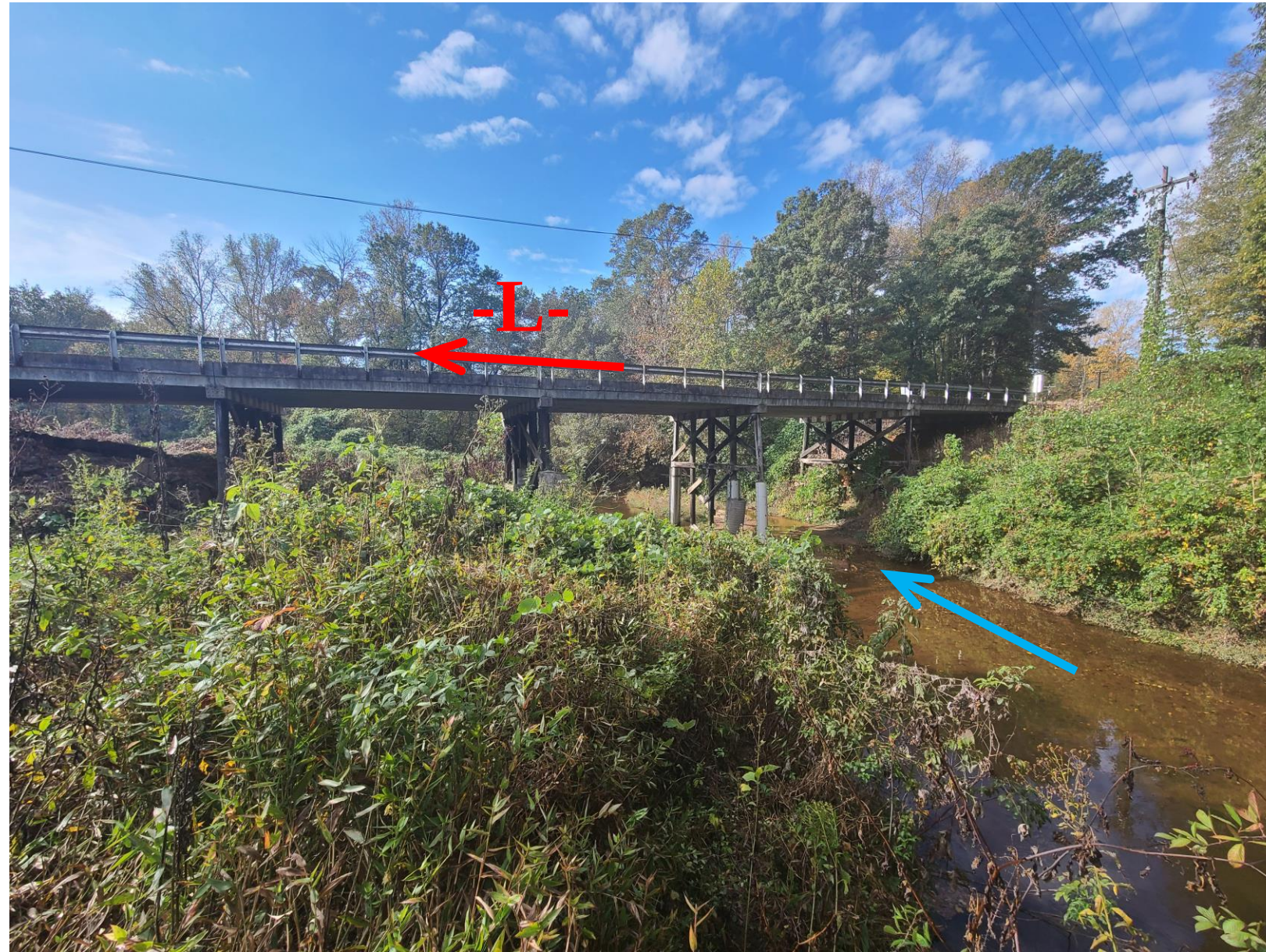
Facing South towards existing bridge
