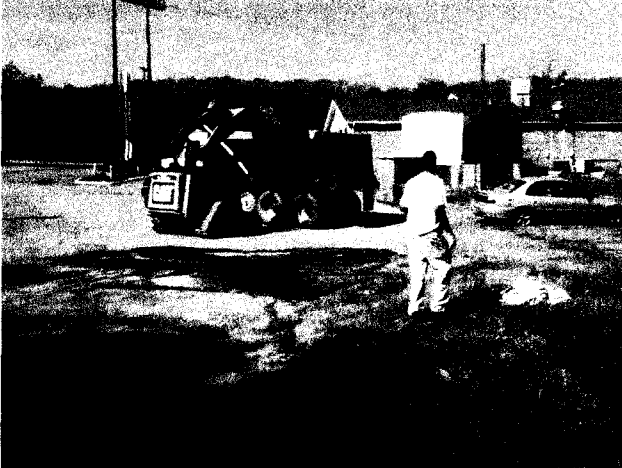
Scraping contaminated gravel off the pavement.
