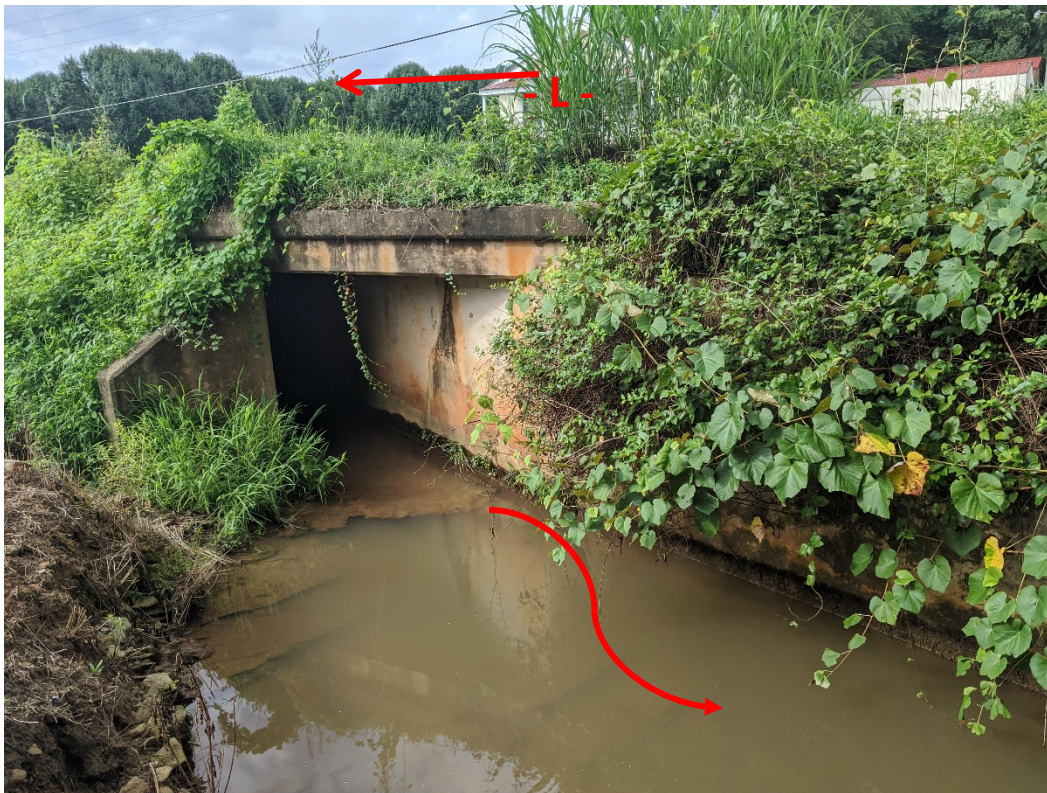
Photograph No. 2: Culvert outlet
