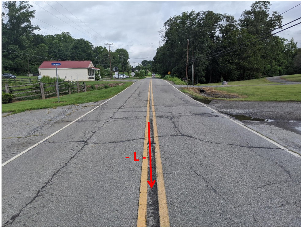
Photograph No. 1: View looking down line
