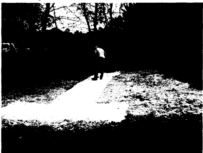
Restoring area with fresh backfill, seed/ straw and erosion control mat.
