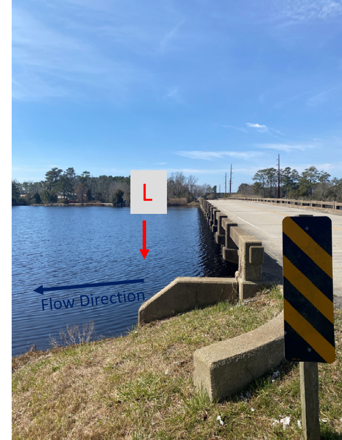
-EB2 facing downstation-
