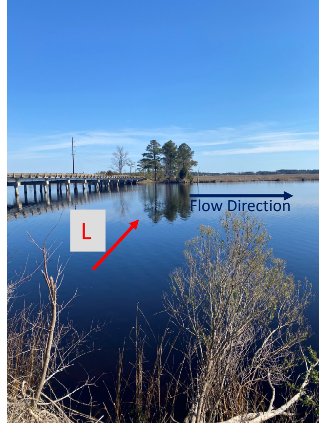
-EB1 facing upstation-
