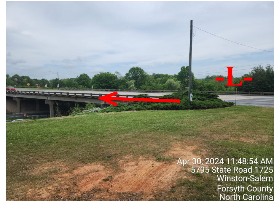
Looking from the west (SW corner)
