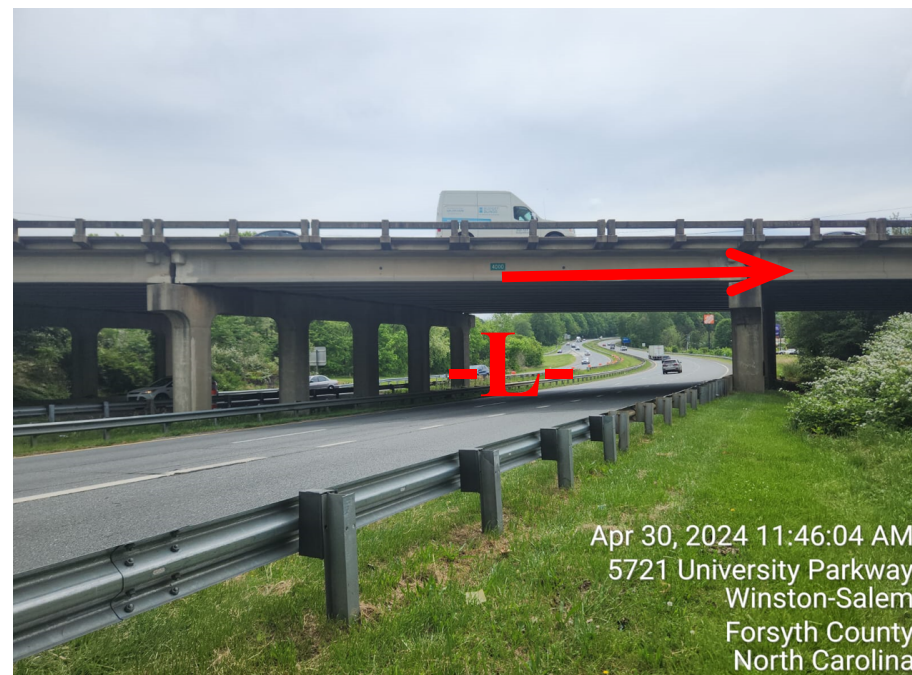
Looking from the East
