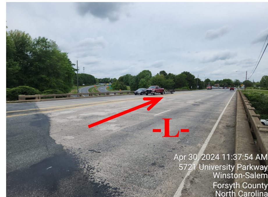
Looking Up-station from SE corner
