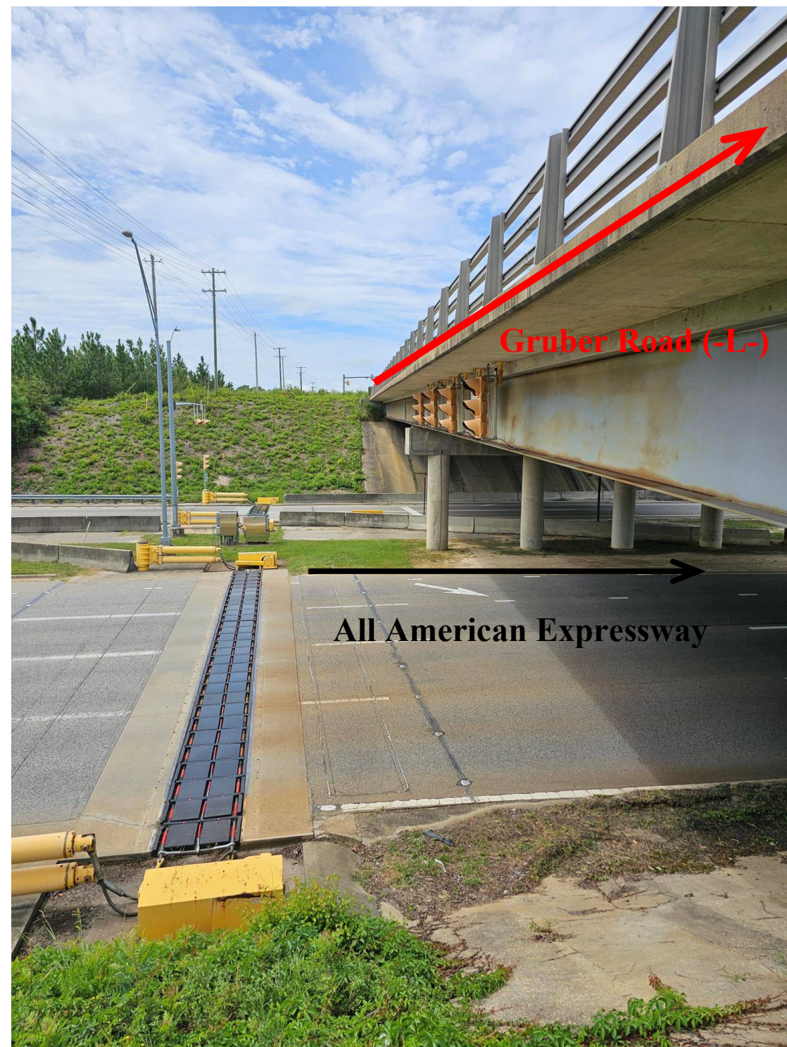
Southeast Corner of Existing Bridge Facing West-Southwest
