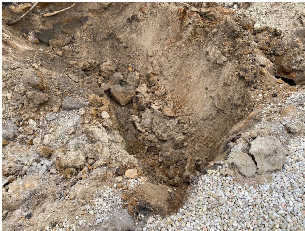
Photo 12 – View of the excavation basin following removal of UST 2 on 1/16/2025.
