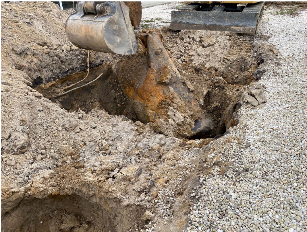
Photo 11 – View of the removal of UST 2 on 1/16/2025.
