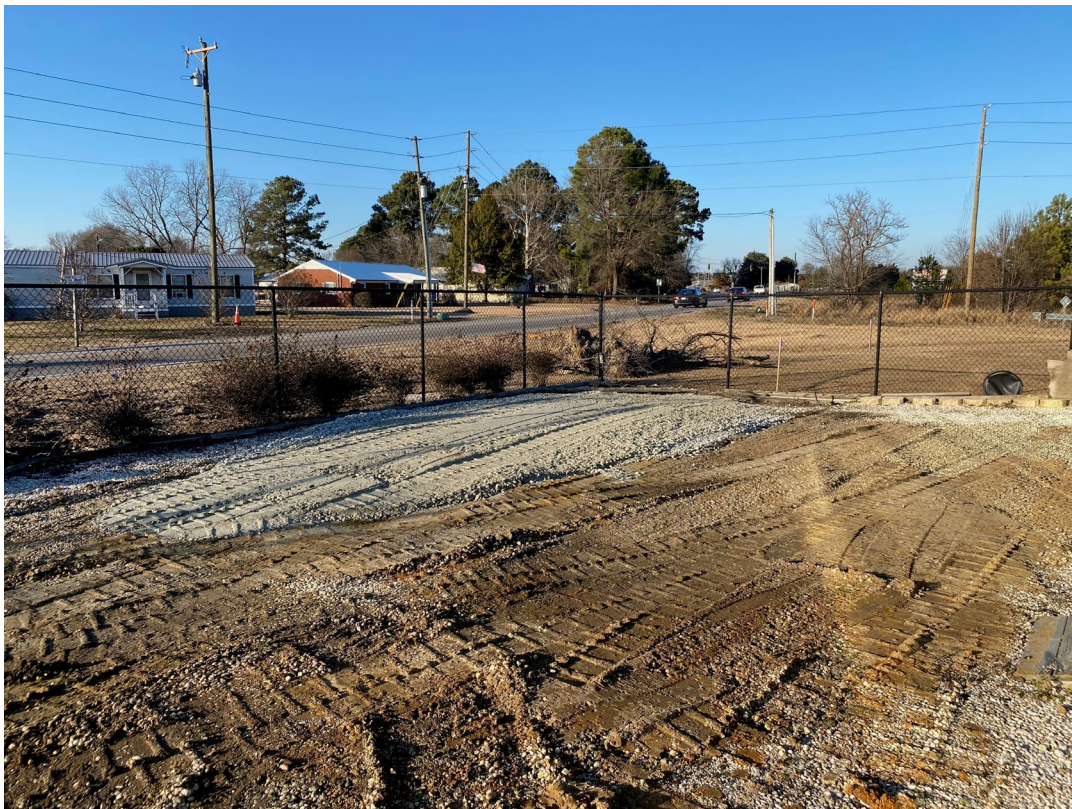
Photo 21 – View of the placement of ABC stone to cap excavation on 1/16/2025.
