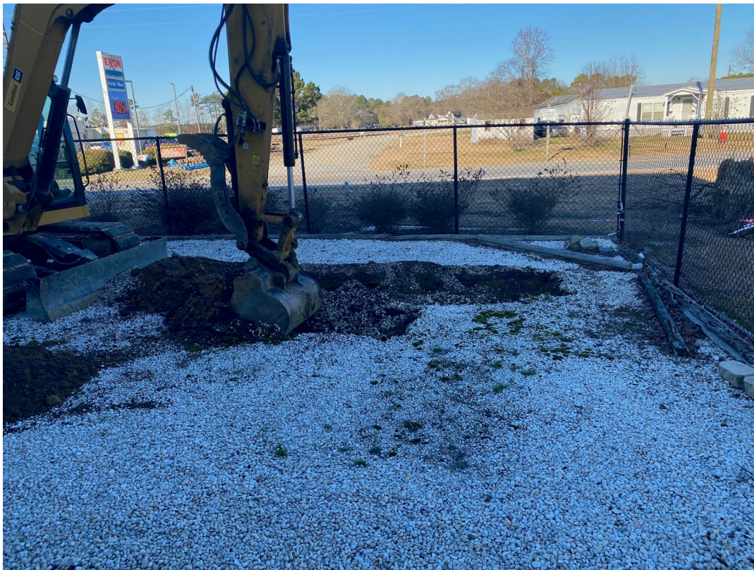
Photo 3 – View of excavation to expose top of USTs facing northeast on 1/15/2025.
