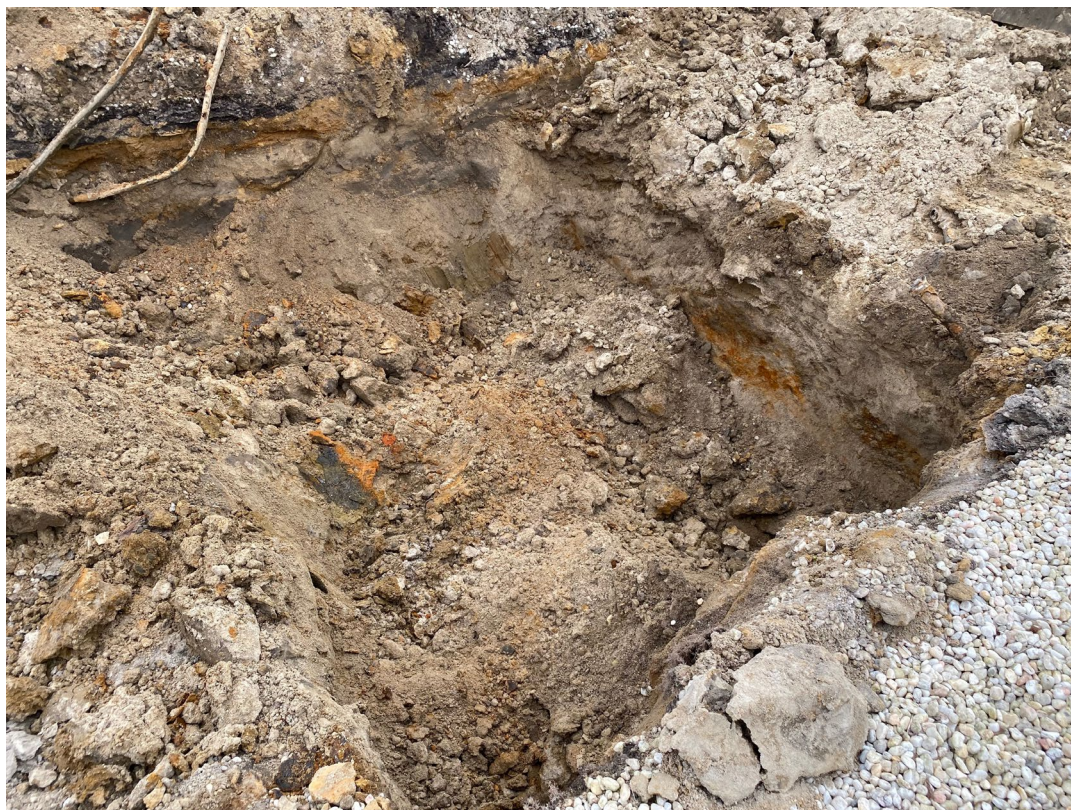
Photo 14 – View of the excavation basin following removal of UST 3 on 1/16/2025.
