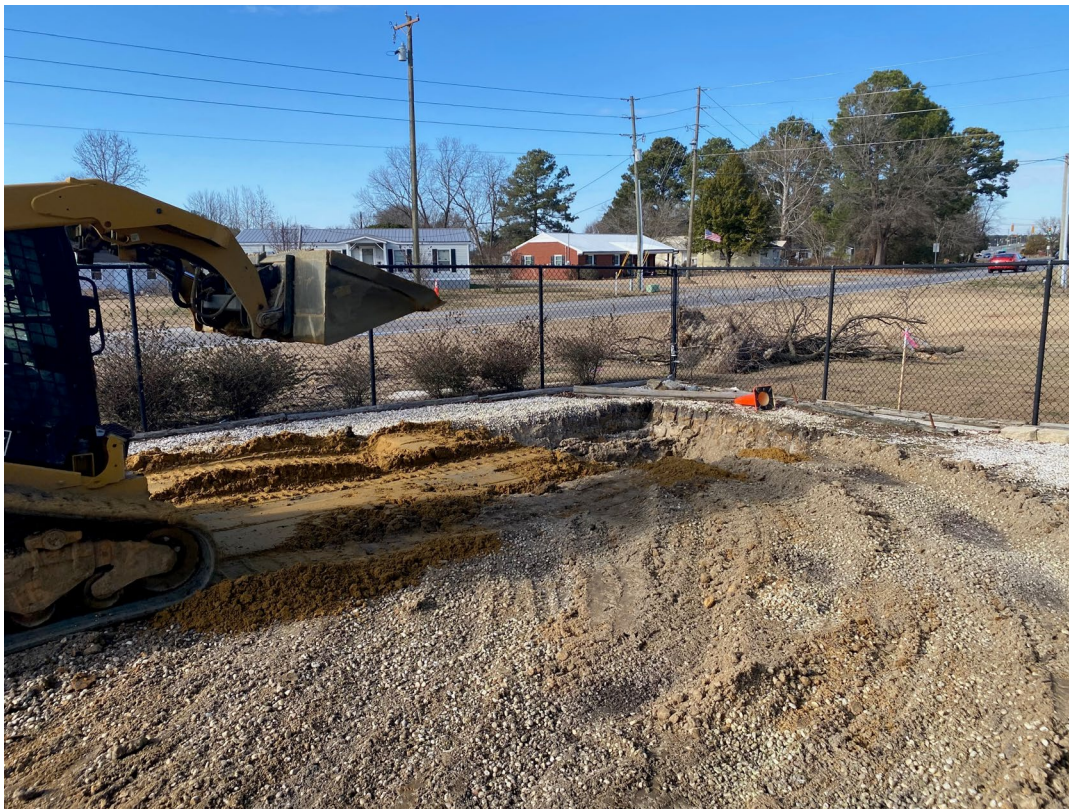
Photo 19 – View of the backfilling procedure using the stockpiled overburden material on 1/16/2025.
