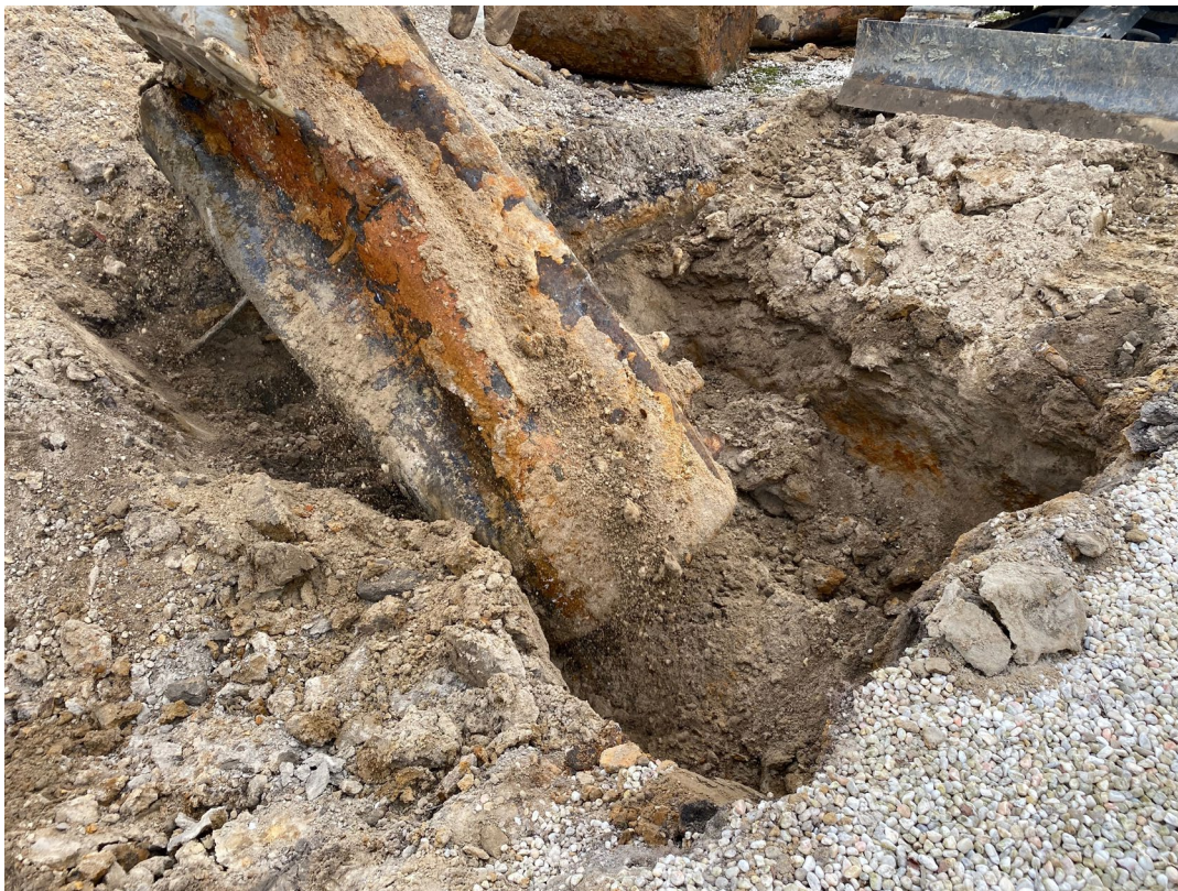
Photo 13 – View of the removal of UST 3 on 1/16/2025.
