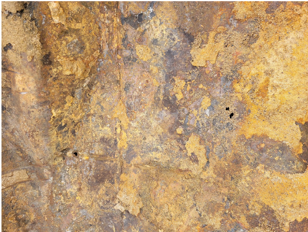
Photo 18 – View of tank with severe rusting and through holes (typical) on 1/16/2025.
