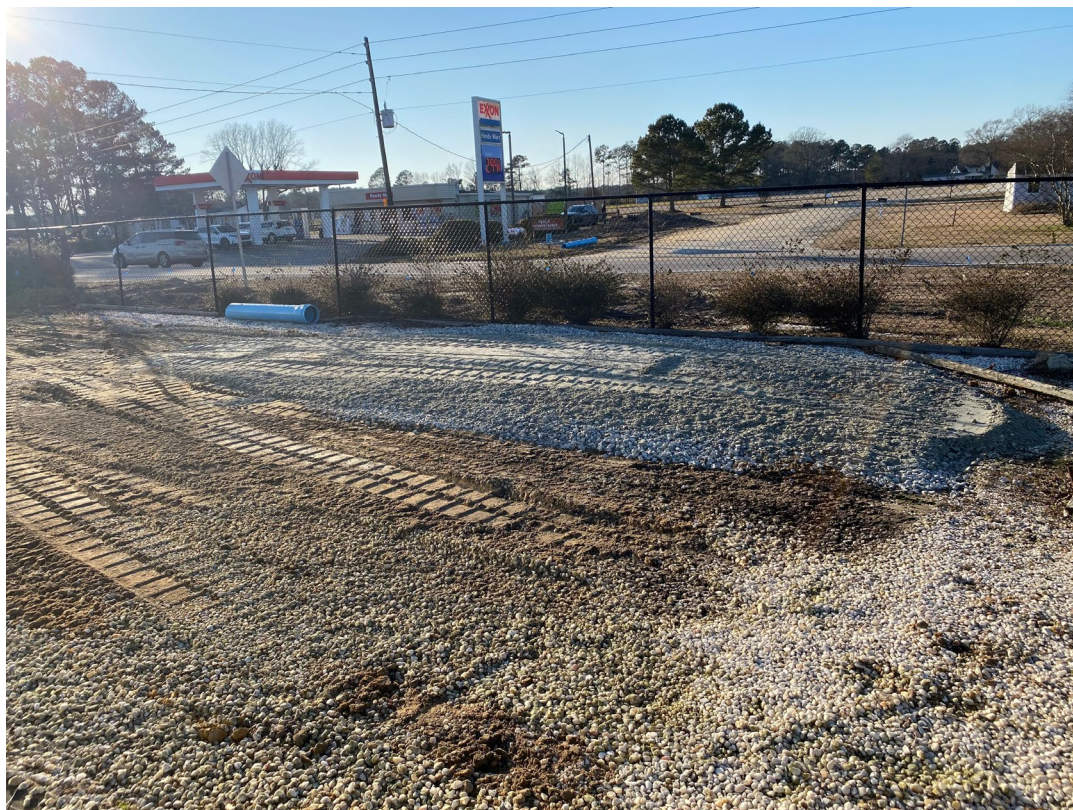
Photo 22 – View of the imported ABC stone used to cap the excavation on 1/16/2025.
