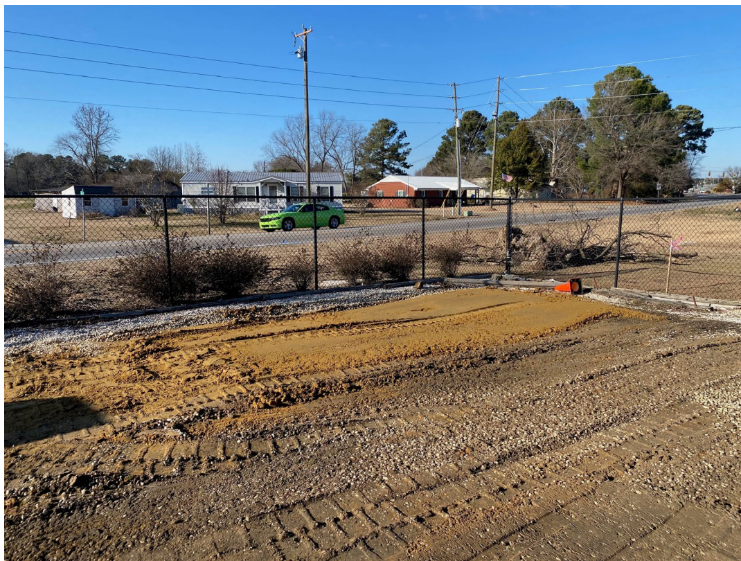
Photo 20 – View of the backfilling activities completed with imported material to replace the tank volume on 1/16/2025.
