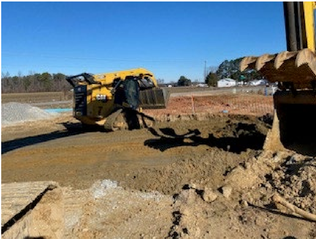
Photo 21 – View of the backfilling activities completed with imported material to replace the tank volume on 1/15/2025.
