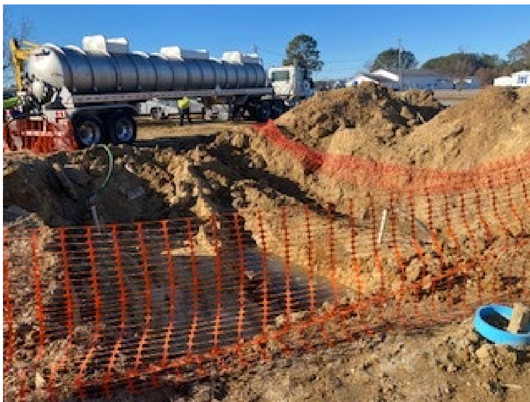
Photo 8 – View of the removal of liquids from within UST 2 using a vacuum tanker truck on 1/14/2025.
