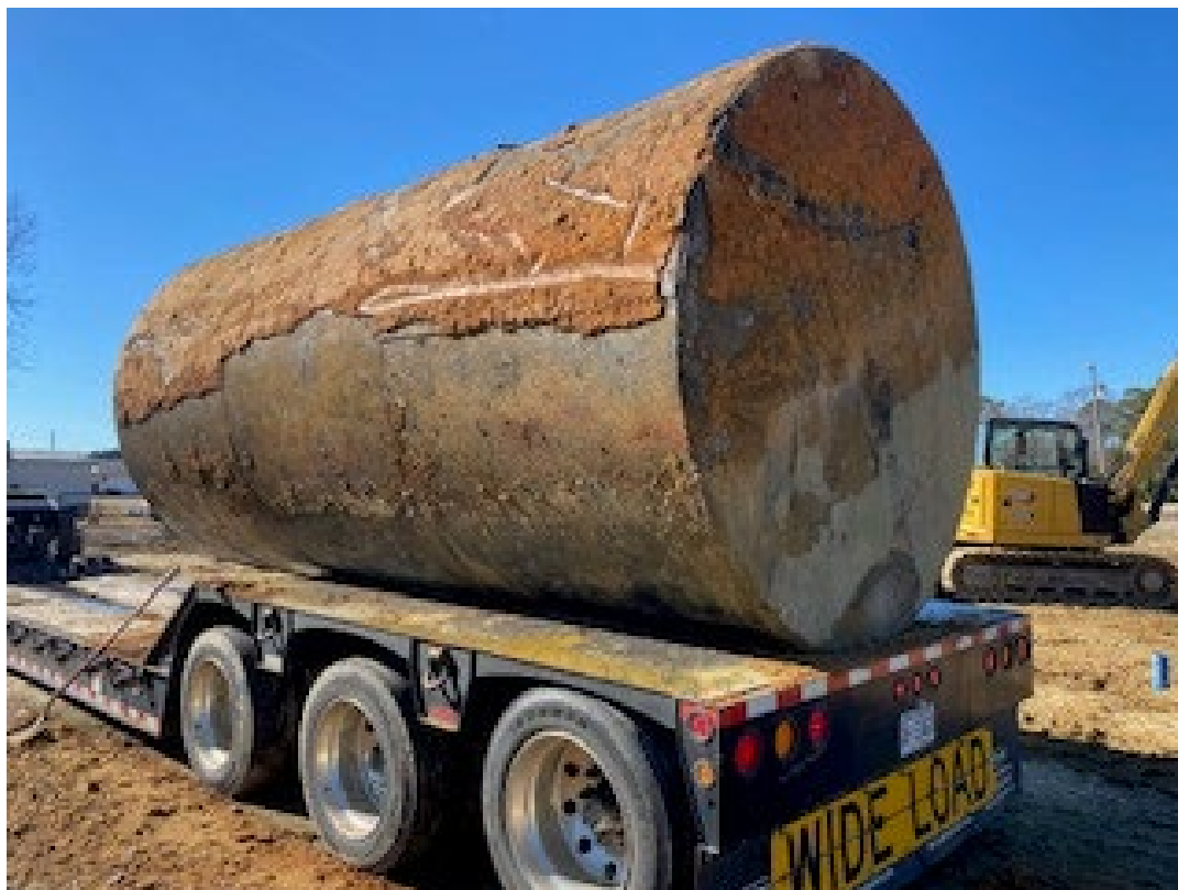
Photo 13 – View of the UST 1 loaded on to a flat bed trailer on 1/14/2025.
