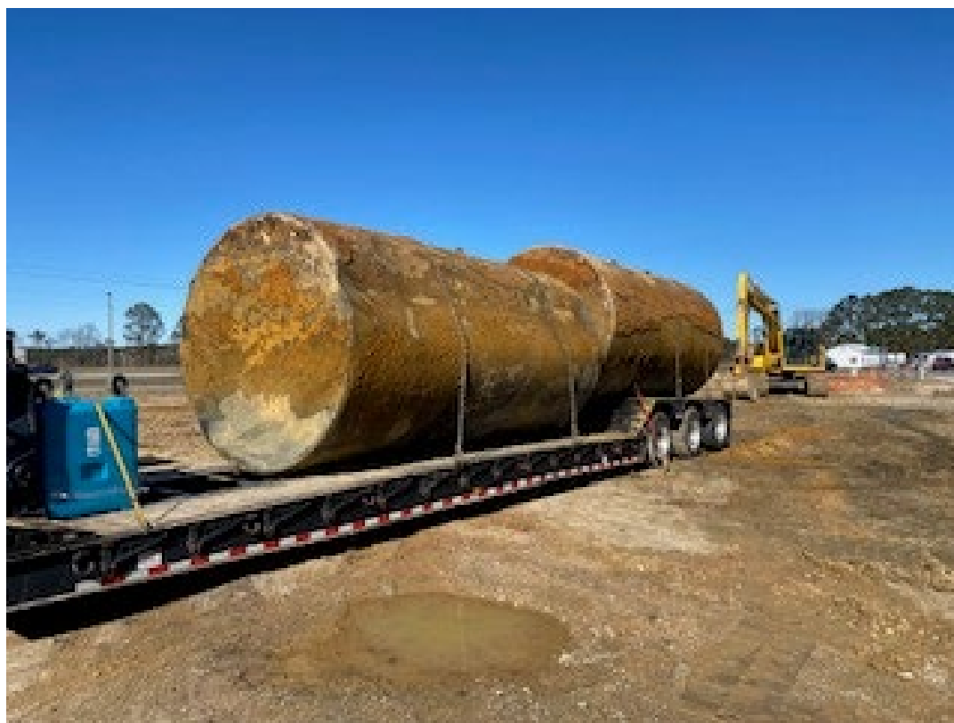
Photo 18 – View of the UST 1 and 2 loaded, secured, and ready for transport off site for disposal on 1/14/2025.
