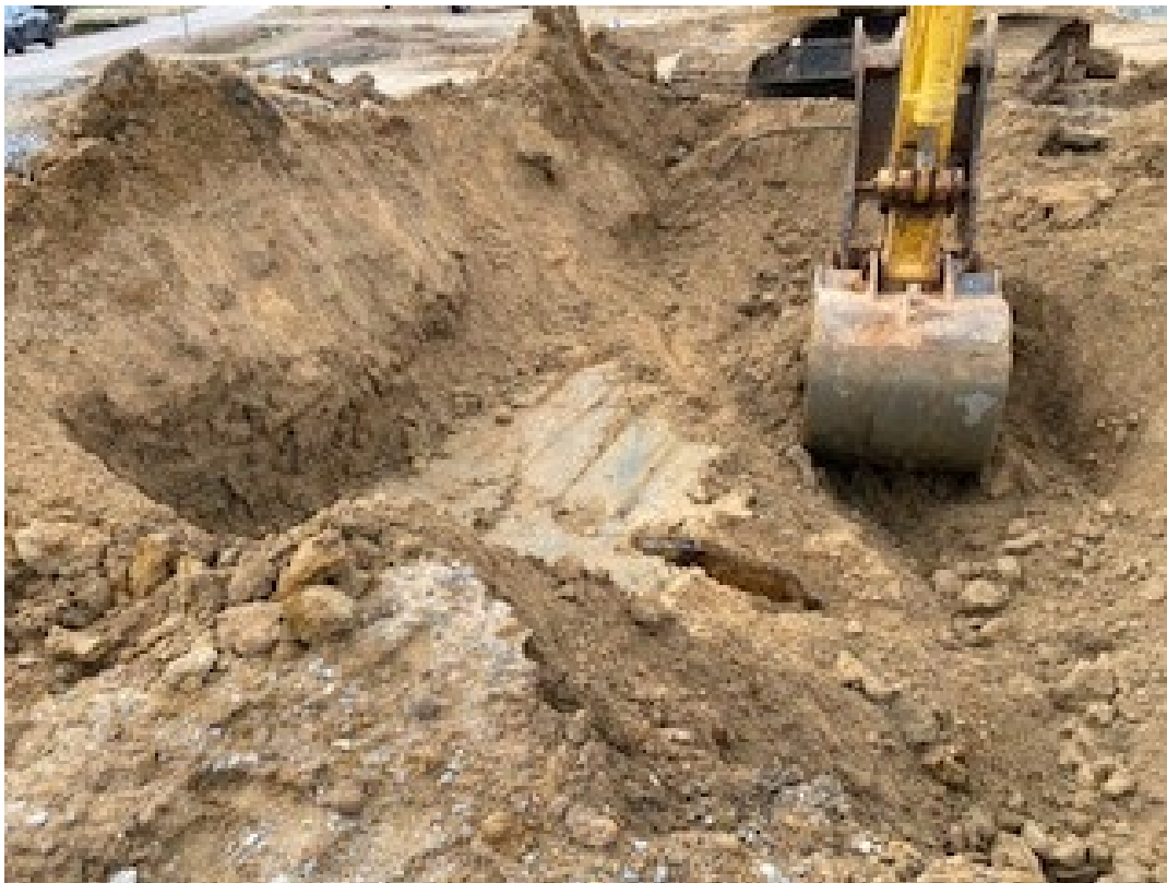
Photo 3 – View of the top of UST 1 exposed using a tracked excavator on 1/13/2025.
