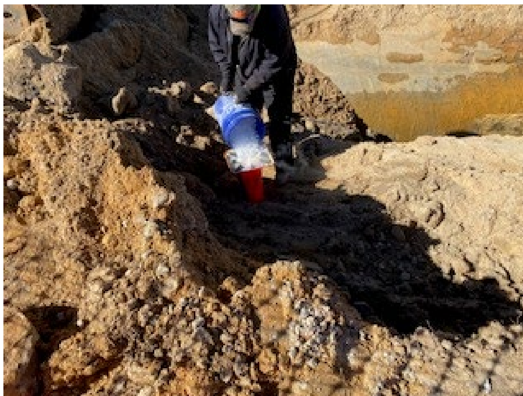
Photo 10 – View of the filling UST 2 with dry ice prior to its removal.
