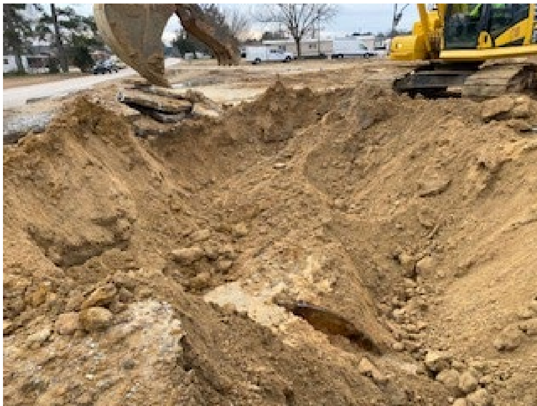
Photo 4 – View of the top of UST 1 exposed further using a tracked excavator on 1/13/2025.
