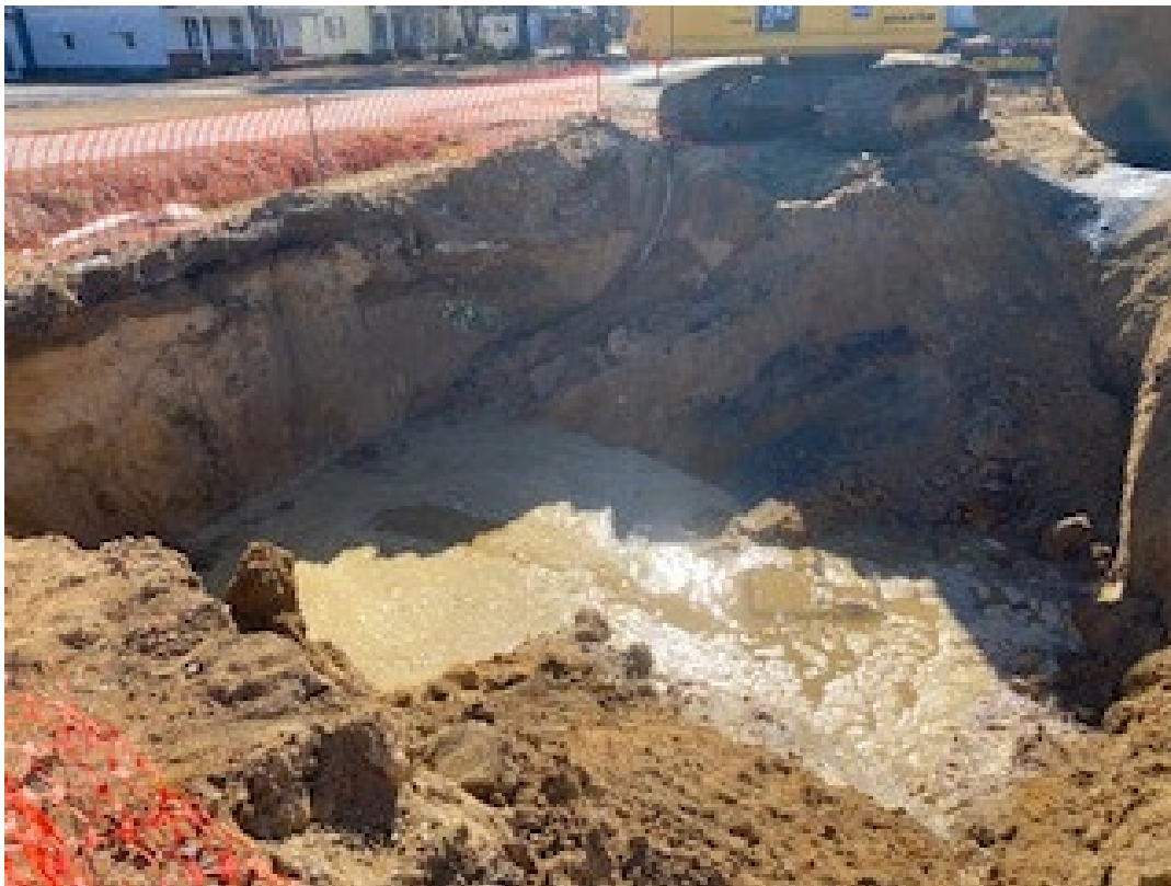
Photo 15 – View of the groundwater observed within the UST basin following removal on 1/14/2025.
