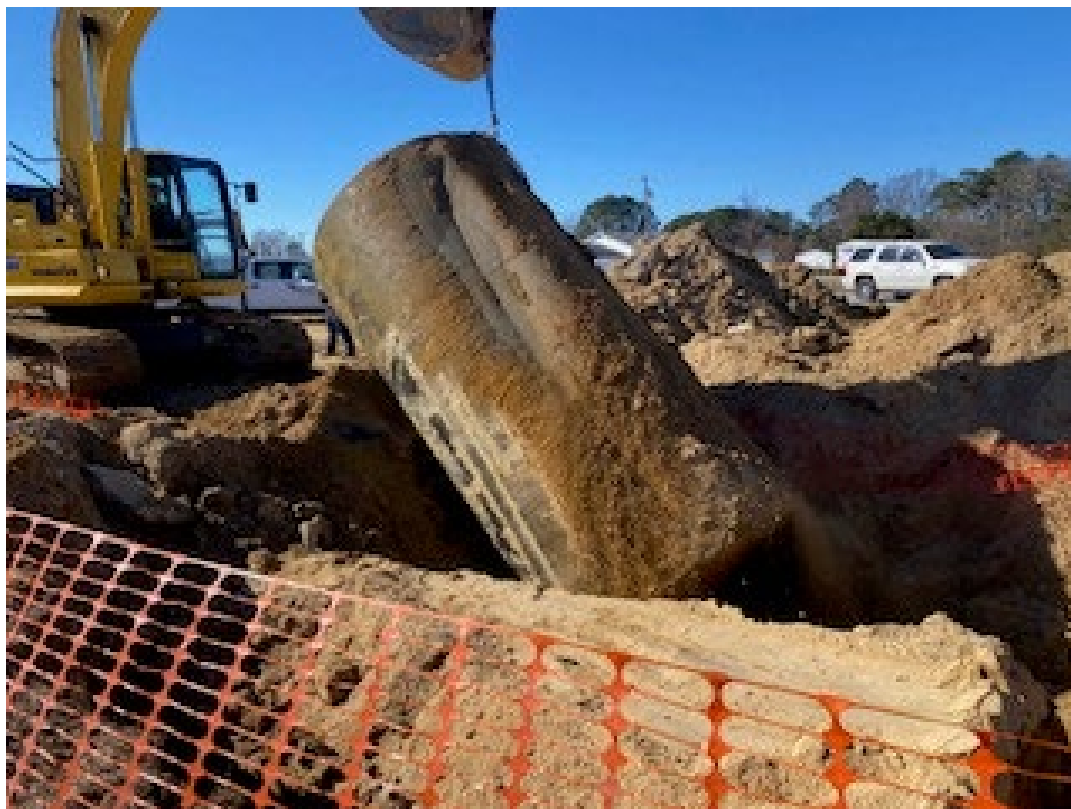
Photo 11 – View of the removal of UST 1 from its basin on 1/14/2025.
