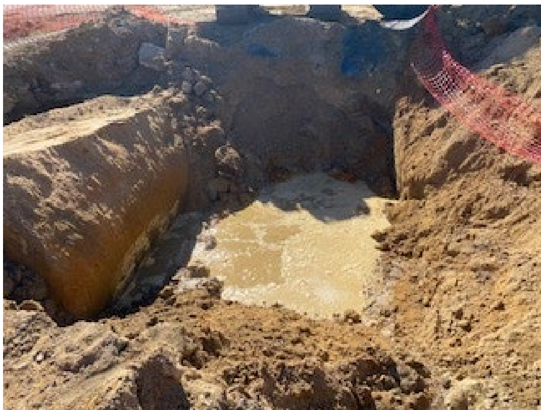
Photo 12 – View of the groundwater observed within the basin following removal of UST-1 on 1/14/2025.
