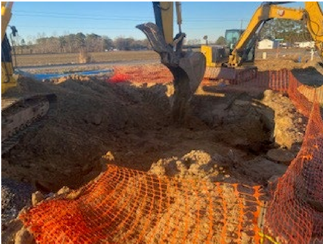
Photo 20 – View of the backfilling procedure using the stockpiled overburden material on 1/14/2025.
