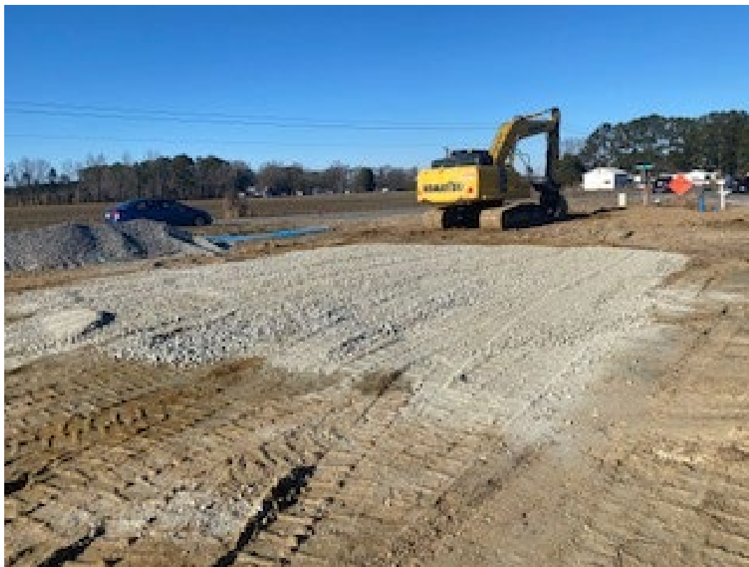
Photo 22 – View of the imported ABC stone using to cap the excavation on 1/15/2025.
