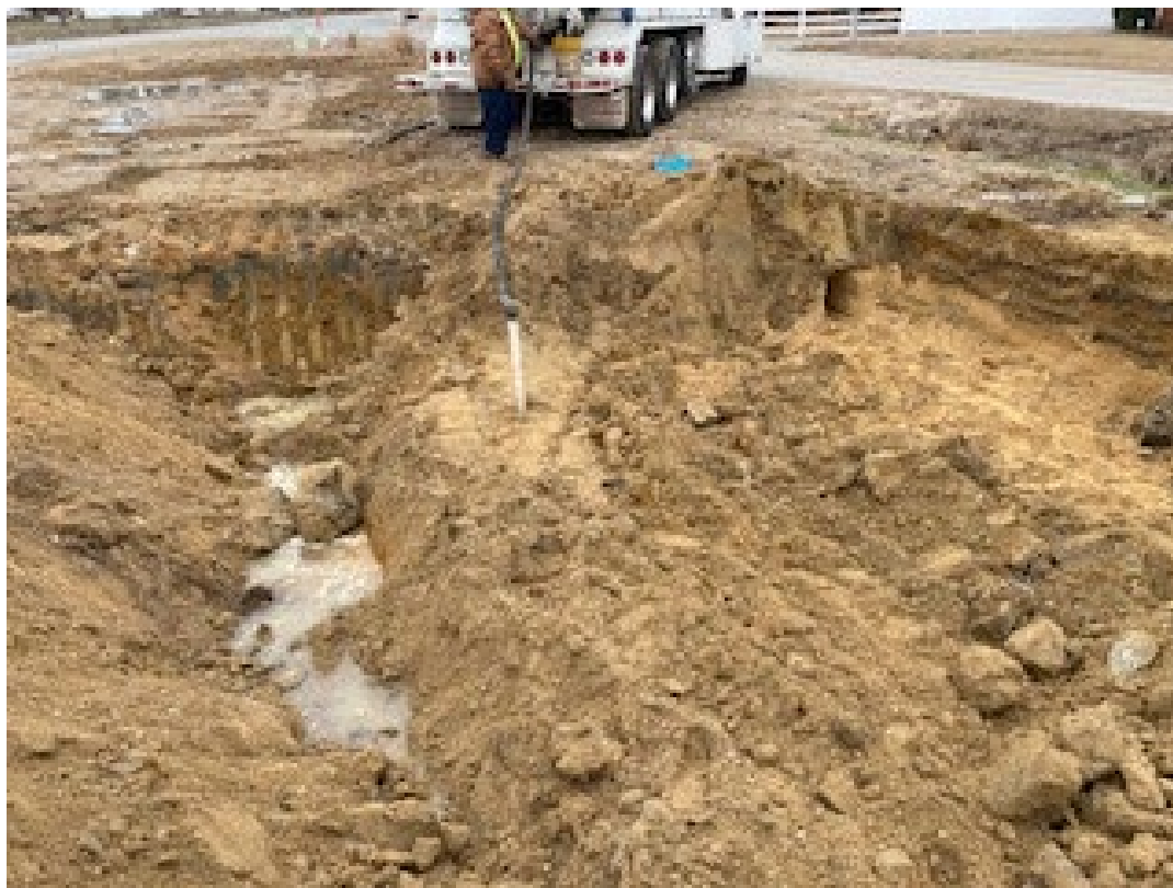
Photo 6 – View of the initial removal of liquids from within UST 1 using a vacuum truck on 1/13/2025.
