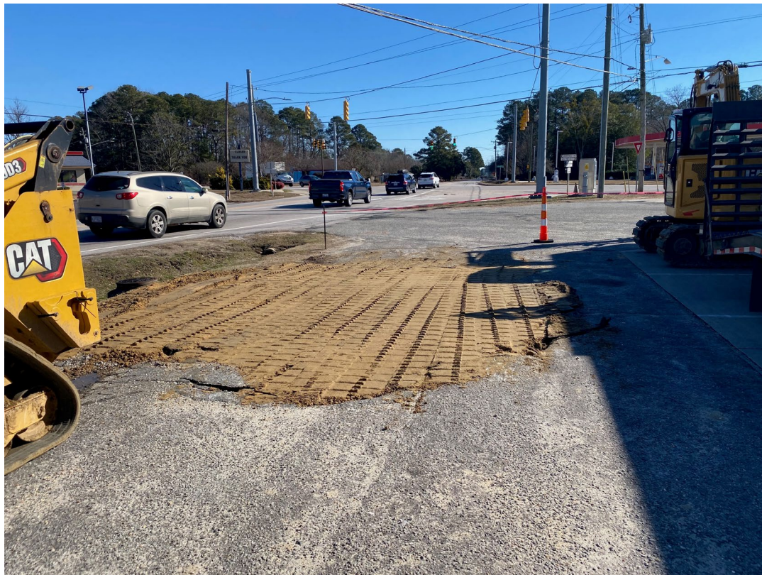
Photo 14 – View of the excavation backfilled with the stockpiled excavated material.
