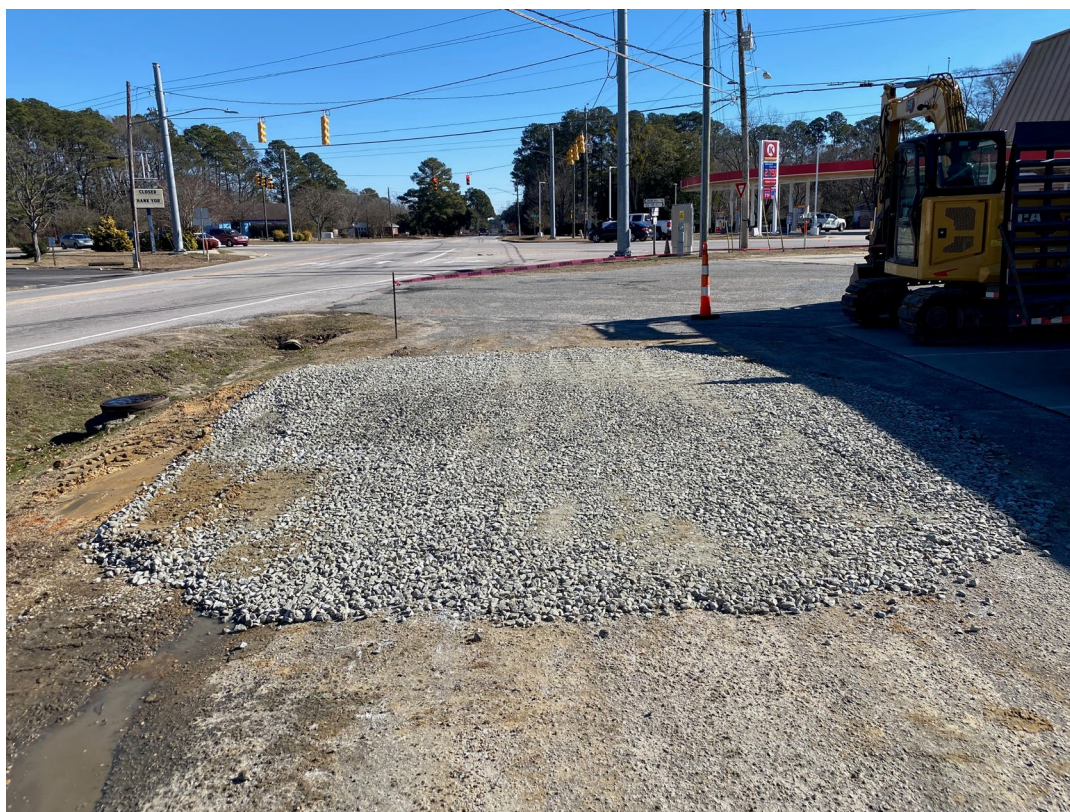
Photo 16 – Another view of the excavated area capped with approximately 6 inches of ABC stone.
