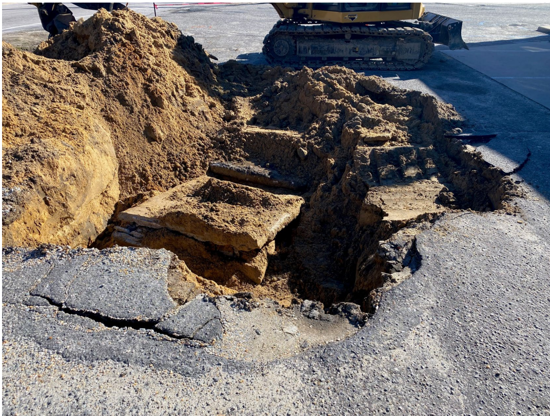
Photo 13 – View of the concrete debris and stockpiled excavated material placed back in the excavation.
