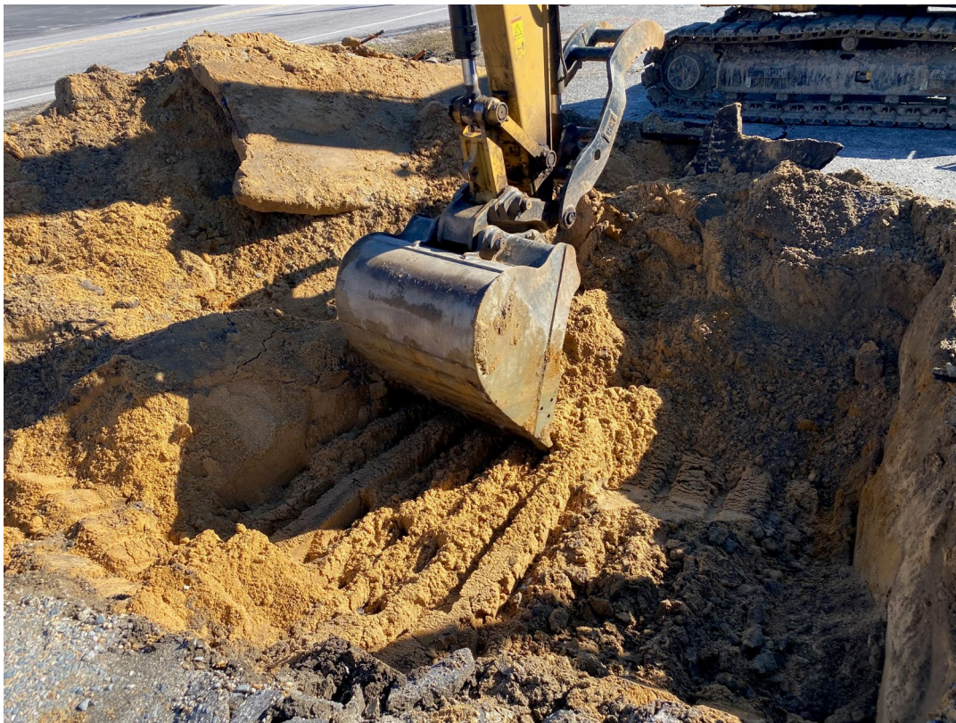
Photo 3 – View of the excavation revealing tan sand fill material, concrete, and construction debris on 1/20/2025.
