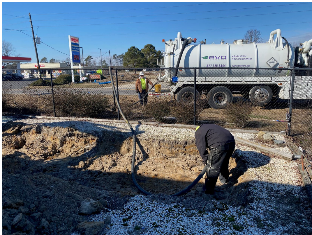
Photo 7 – View of vacuum truck used to pump residual liquids from the USTs facing northwest on 1/16/2025.
