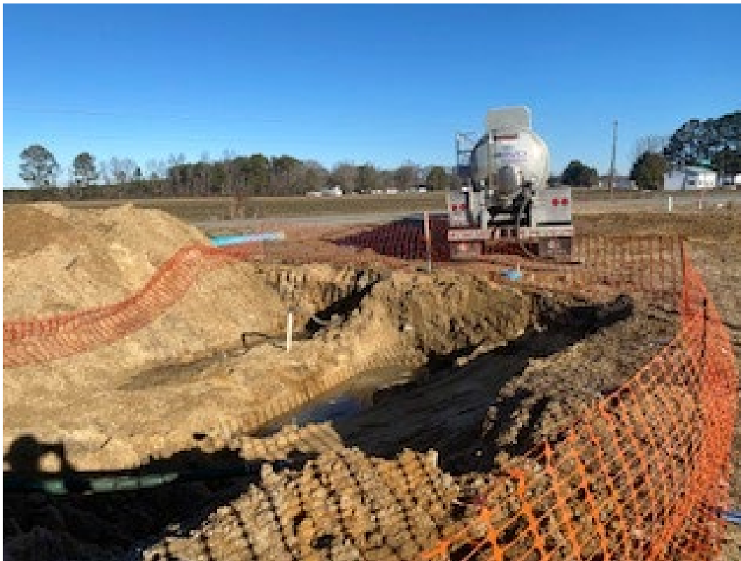
Photo 7 – View of the removal of liquids from within UST 1 using a vacuum tanker truck on 1/14/2025.
