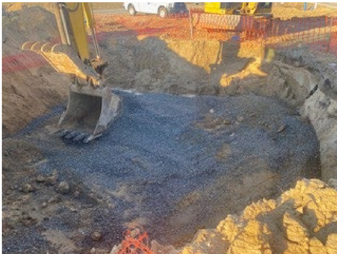
Photo 19 – View of the imported 57 stone placed in the bottom of the excavation to bridge over the groundwater.
