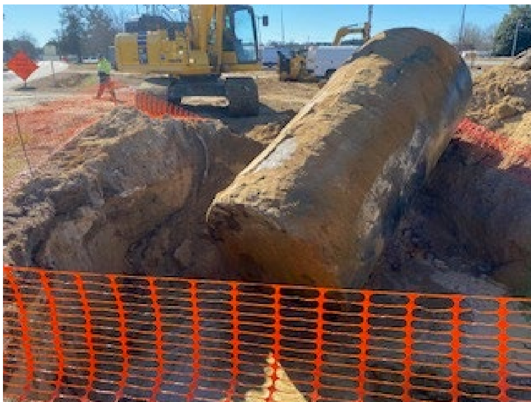
Photo 14 – View of the removal of UST 2 from its basin on 1/14/2025.
