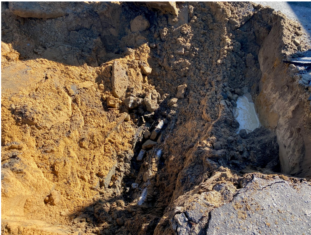
Photo 5 –View of the excavation revealing concrete and other construction debris on 1/20/2025.
