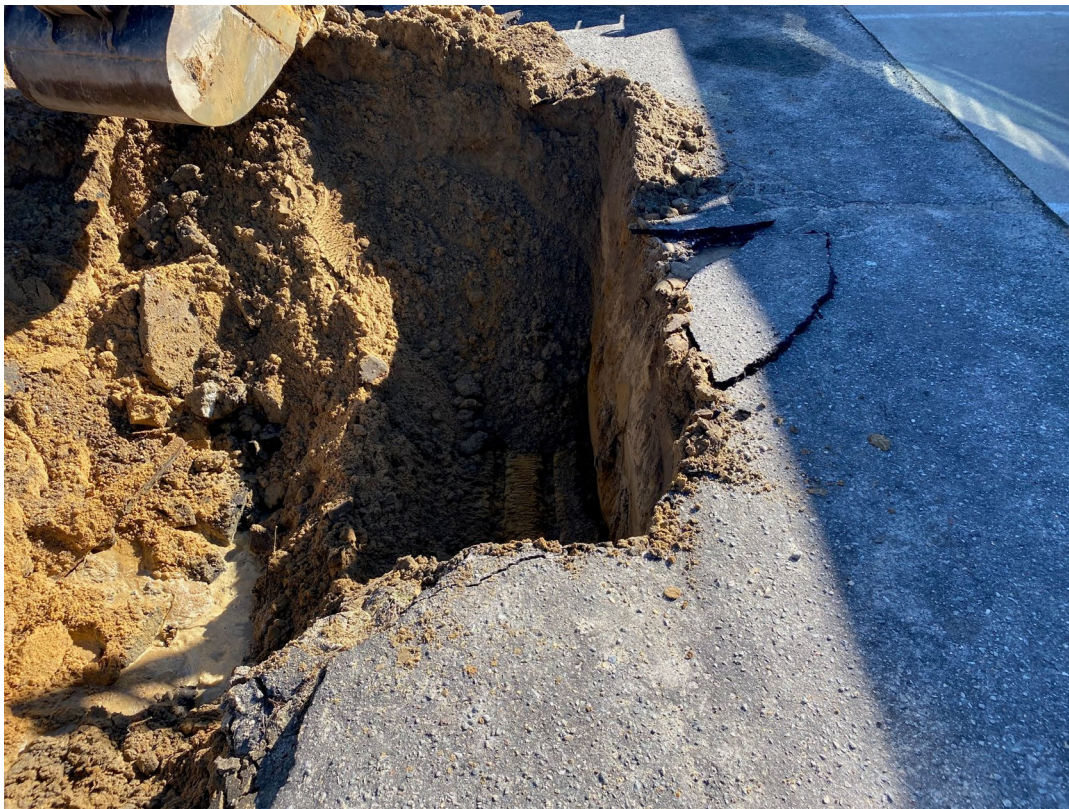
Photo 9 – View of the excavated extended another 3-4 feet to the south in an effort to locate the potential USTs.
