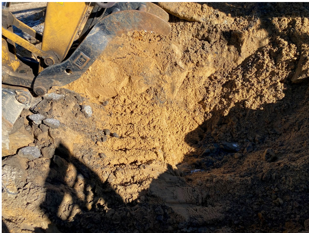
Photo 4 – Another view of the excavation revealing tan sand fill material, concrete, and construction debris on 1/20/2025.
