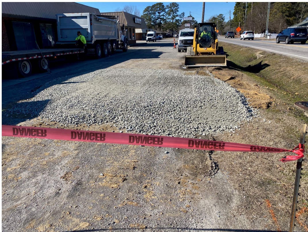
Photo 15 – View of the excavated area capped with approximately 6 inches of ABC stone.
