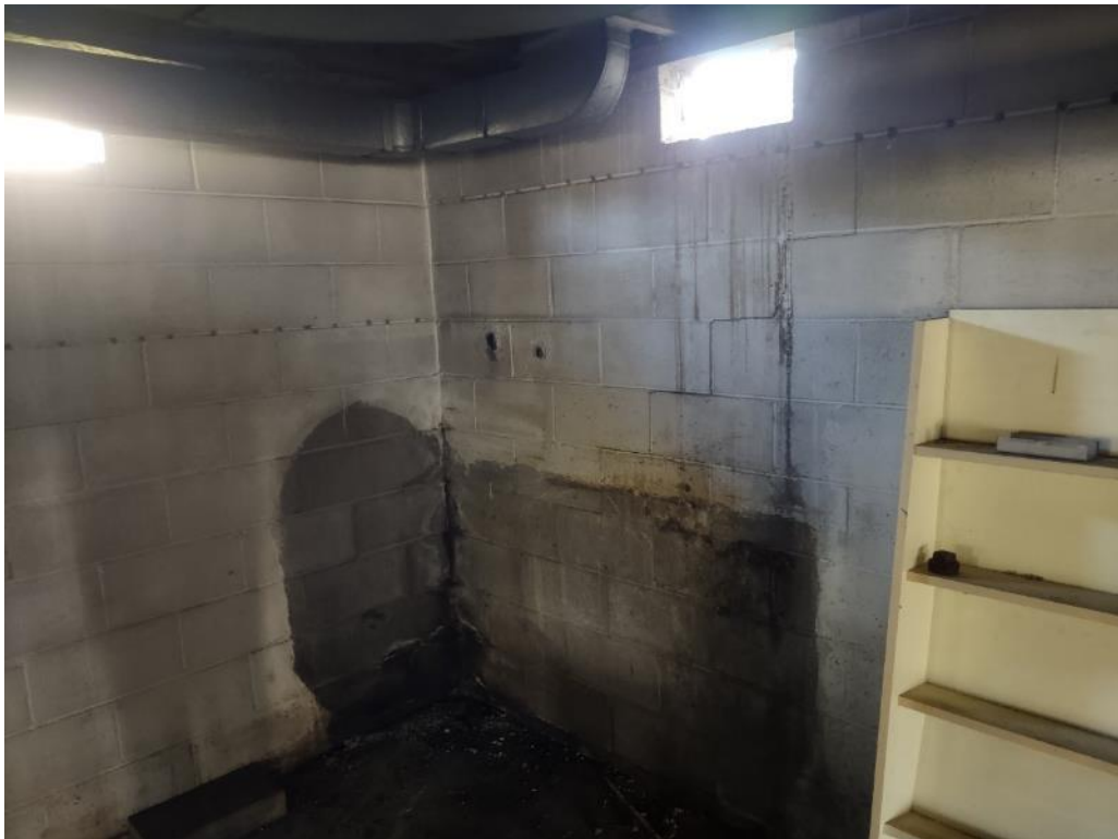
D. Photo of AST location after removal with piping cut flush to the wall inside and to the outside ground surface.
