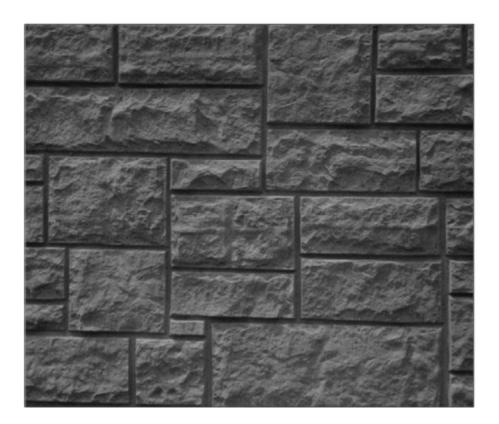
All texture is to be in addition to the nominal thickness of each element within tolerances. Maximum relief of the textured surface shall be  $1\frac{1}{4}$  inch or less.
