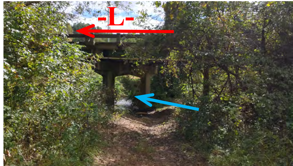
Facing South from North of Existing Bridge
