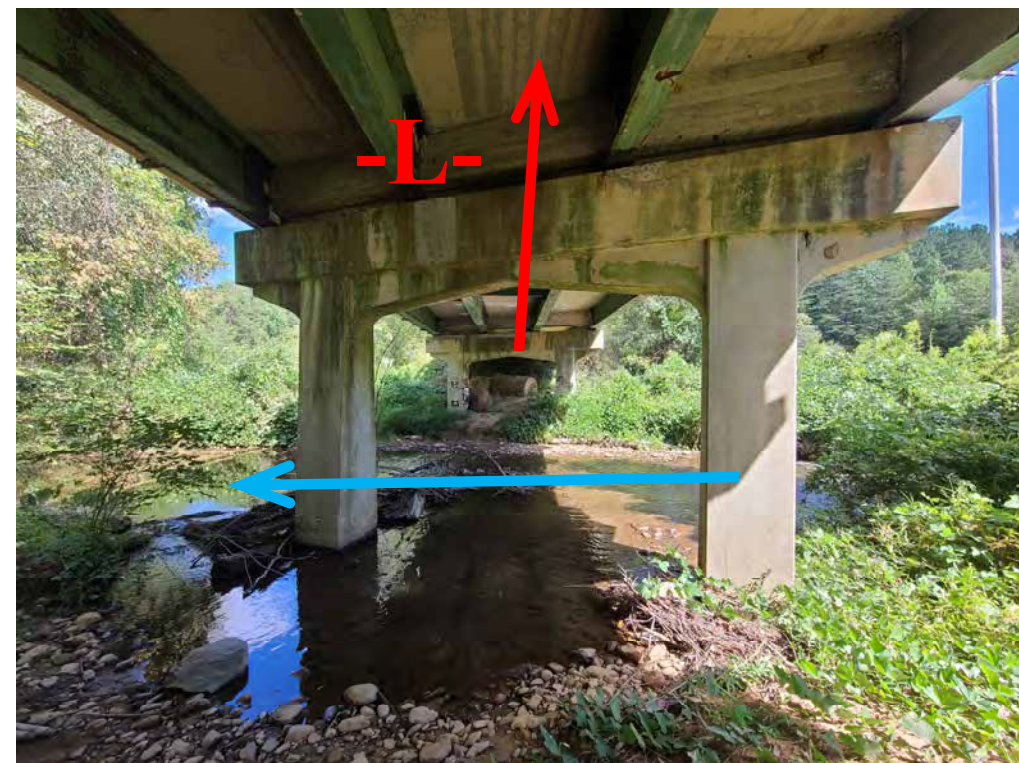
Facing West towards End Bent No. 1
