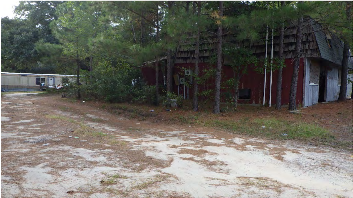
Side of the store building
