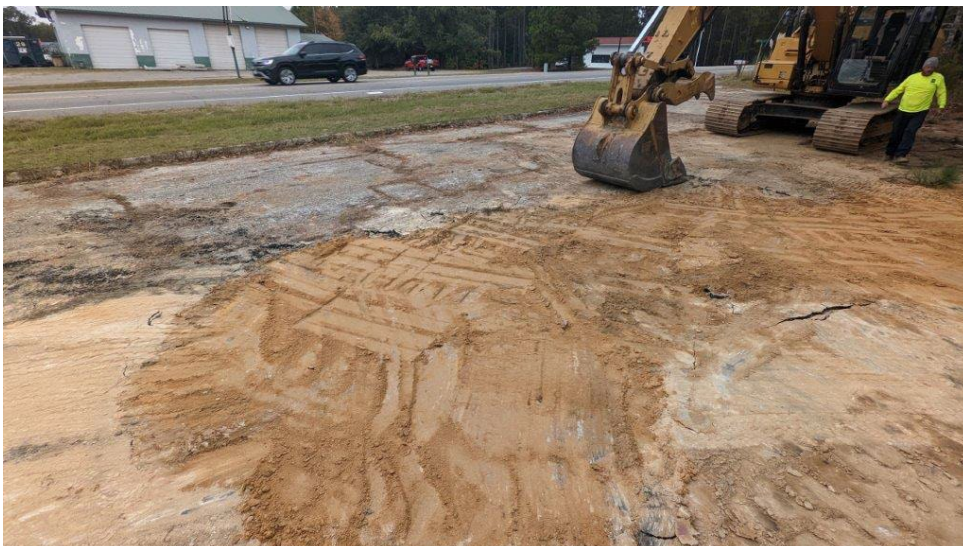
Photograph 7: Former dispenser island area after backfilling excavation.
