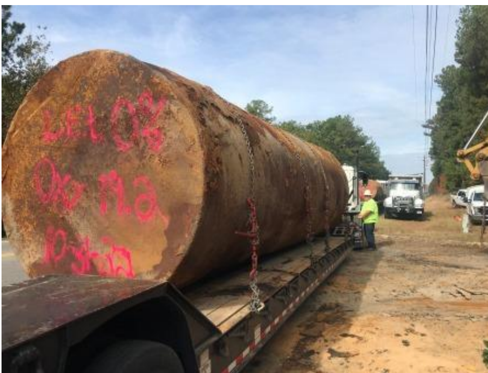
Photograph 8: Evo loading UST#3 on to trailer. UST in good condition, no pitting or holes.
