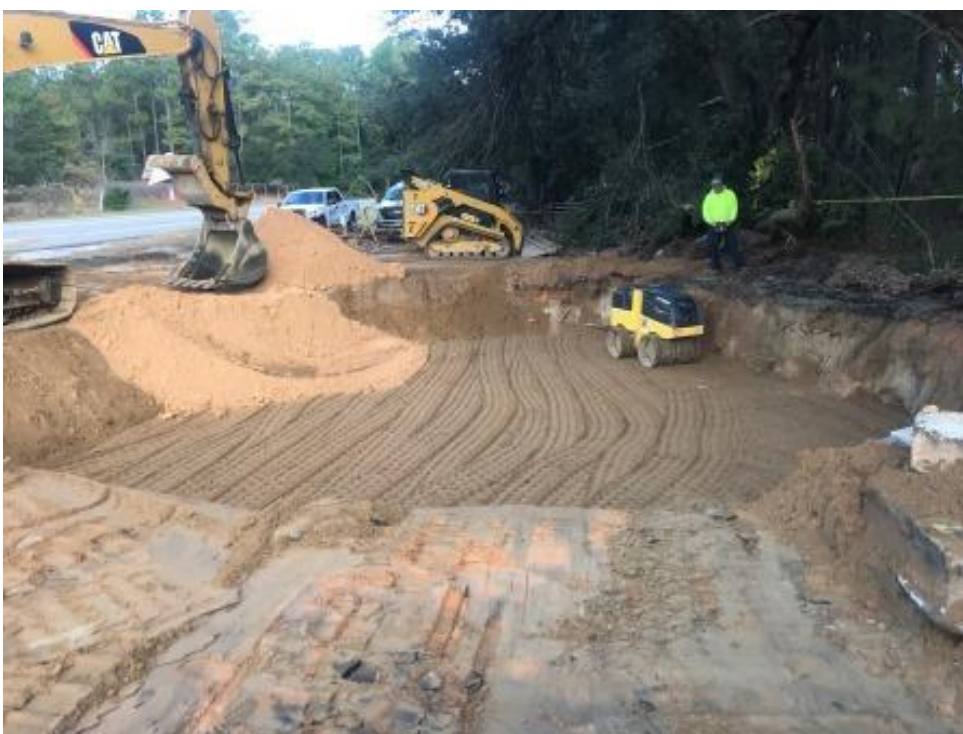
Photograph 12: Evo performing compaction on excavation.
