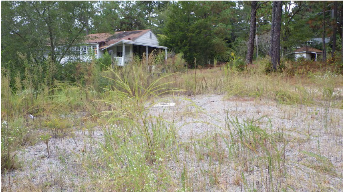
UST removal area.
