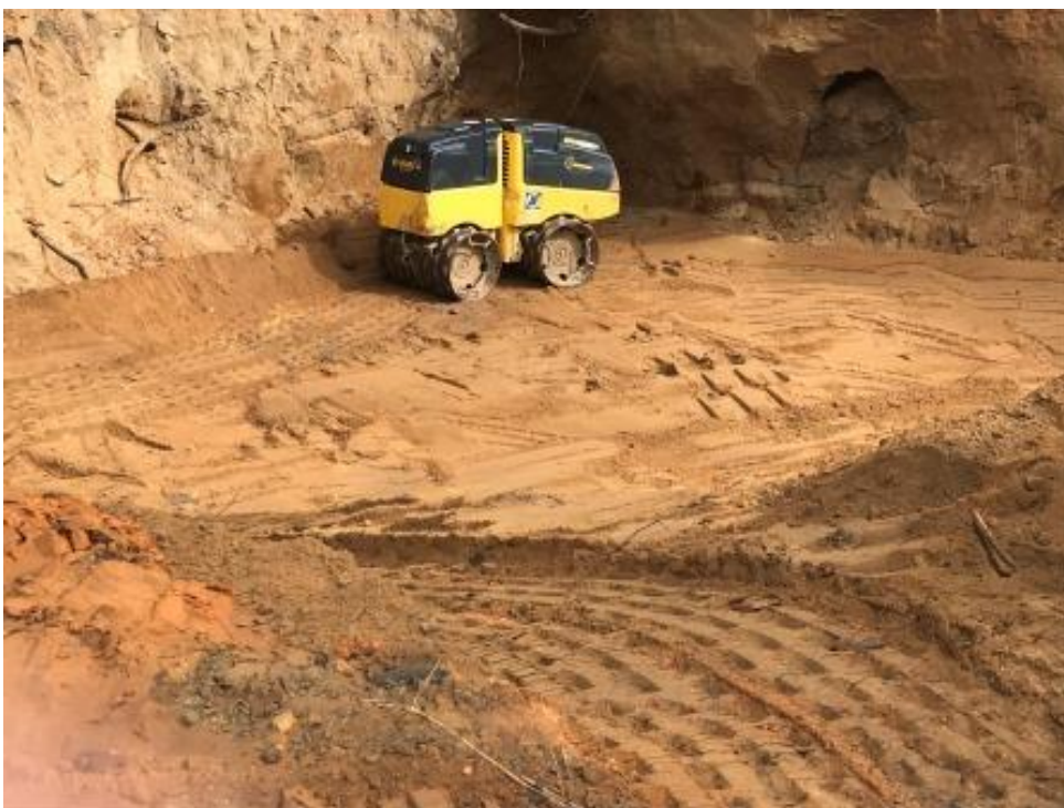
Photograph 9: EVO compacting excavation with remote compactor.
