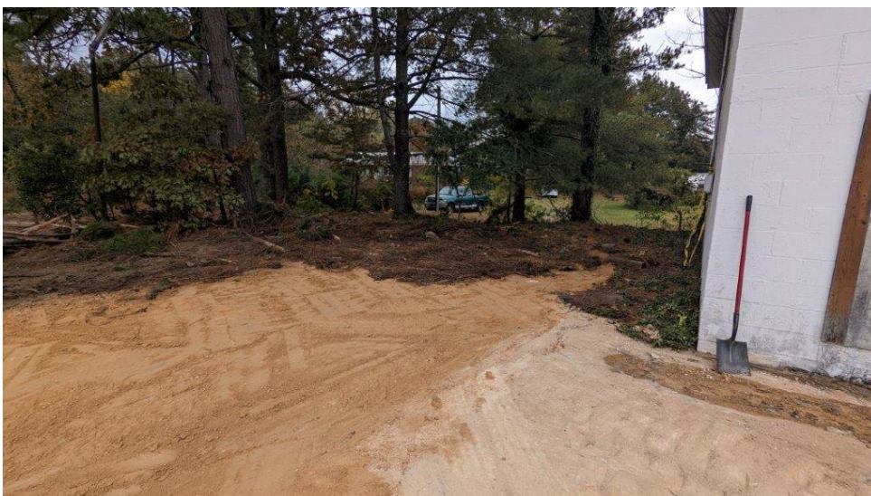
Photograph 8: Former UST area after backfilling excavation.
