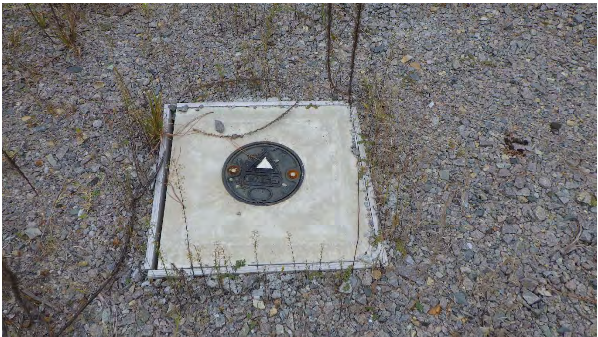
Recently installed monitoring well
