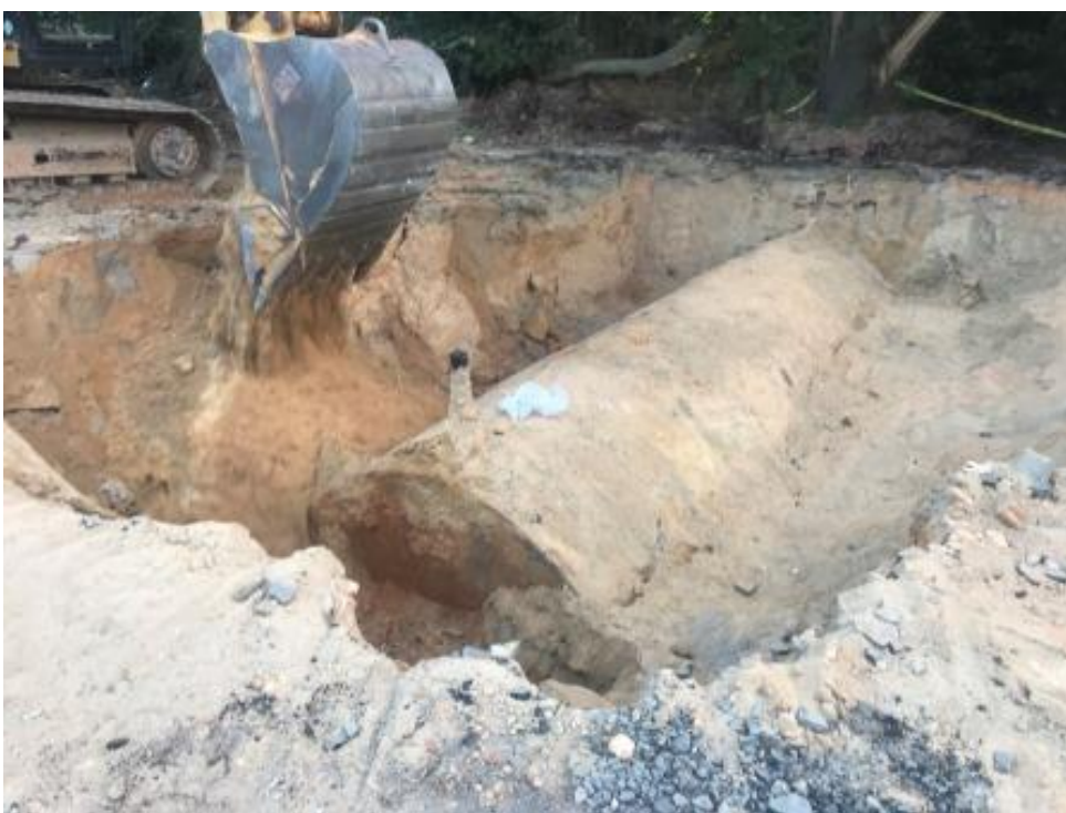
Photograph 2: EVO uncovering UST#1.
