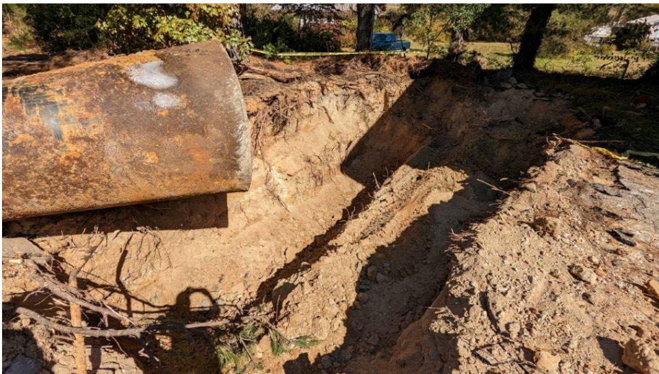
Photograph 2: Removing USTs from the excavation.
