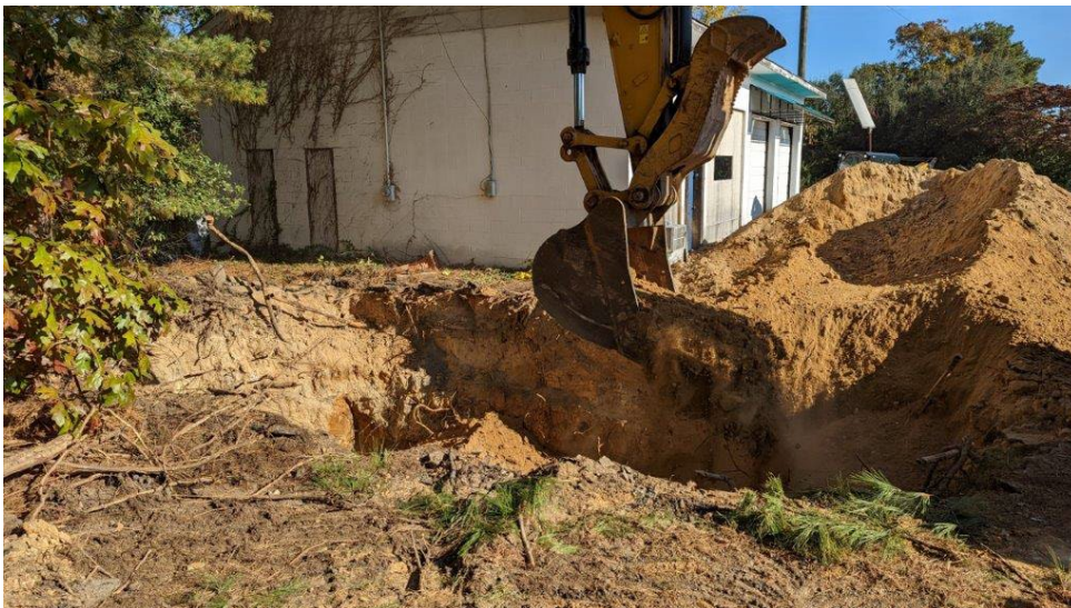
Photograph 6: Backfilling UST excavation.
