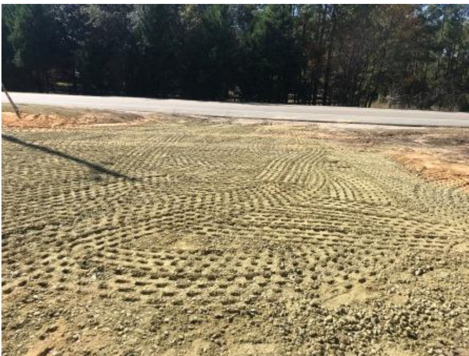
Photograph 16: Photograph of final backfilled excavation.
