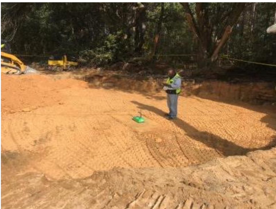
Photograph 13: Ken Thorpe performing compaction testing.
