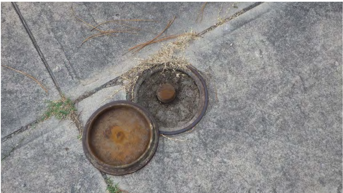
UST fill port uncovered.
