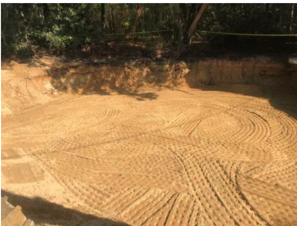
Photograph 10: Open excavation, awaiting compaction testing.
