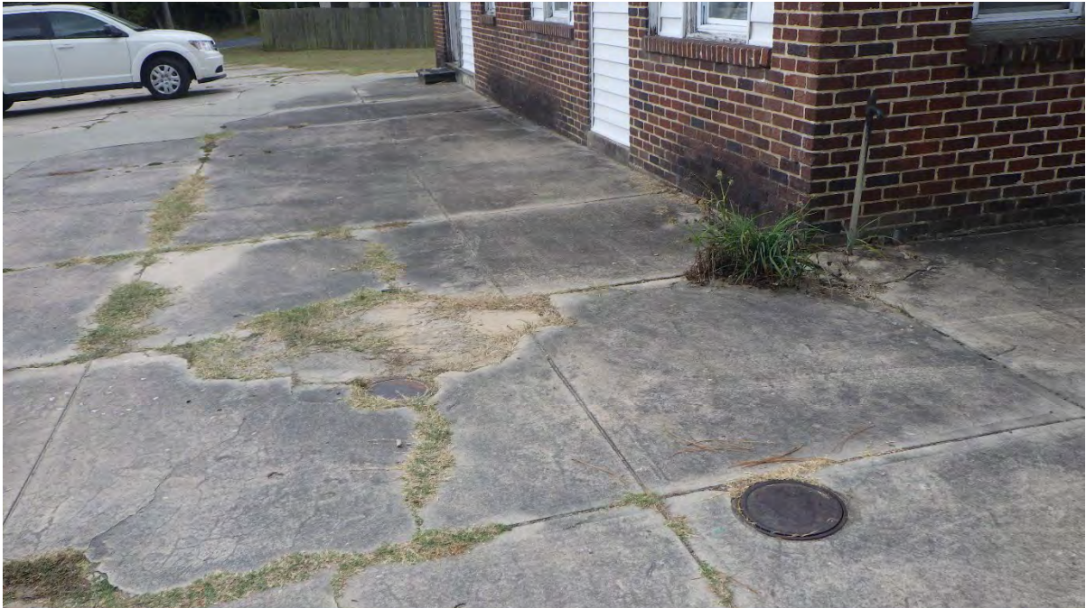
UST fill port with cover
