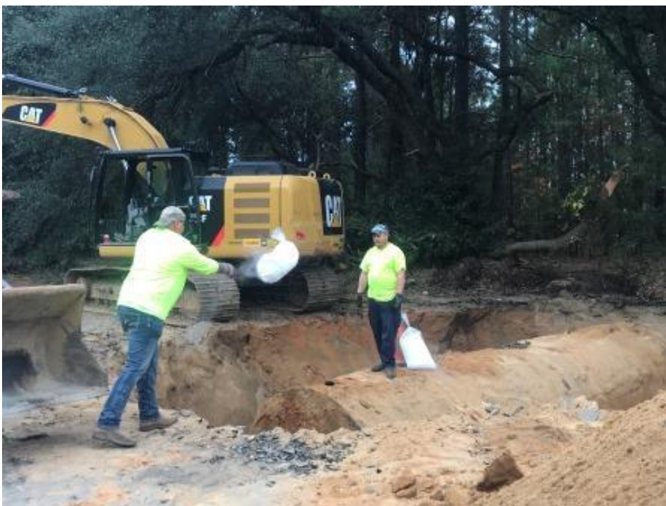
Photograph 3: EVO personnel preparing to add dry ice to inert UST#1.
