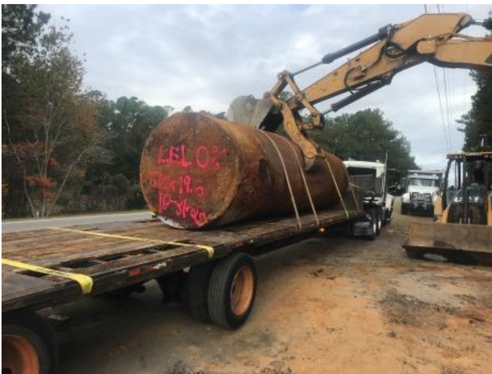
Photograph 7: EVO loading UST#2 on trailer. UST was in good condition, no holes or pitting.
