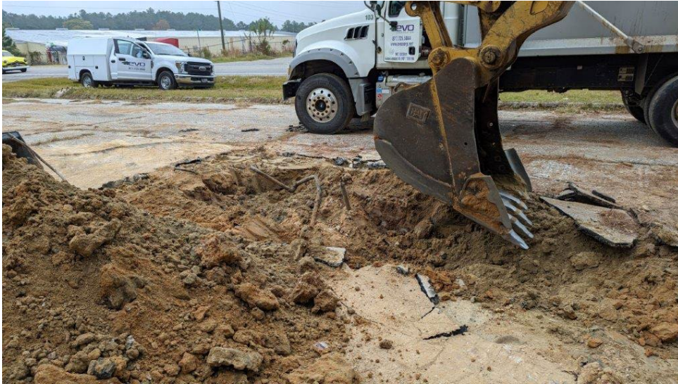
Photograph 5: Removing product lines and dispenser island.
