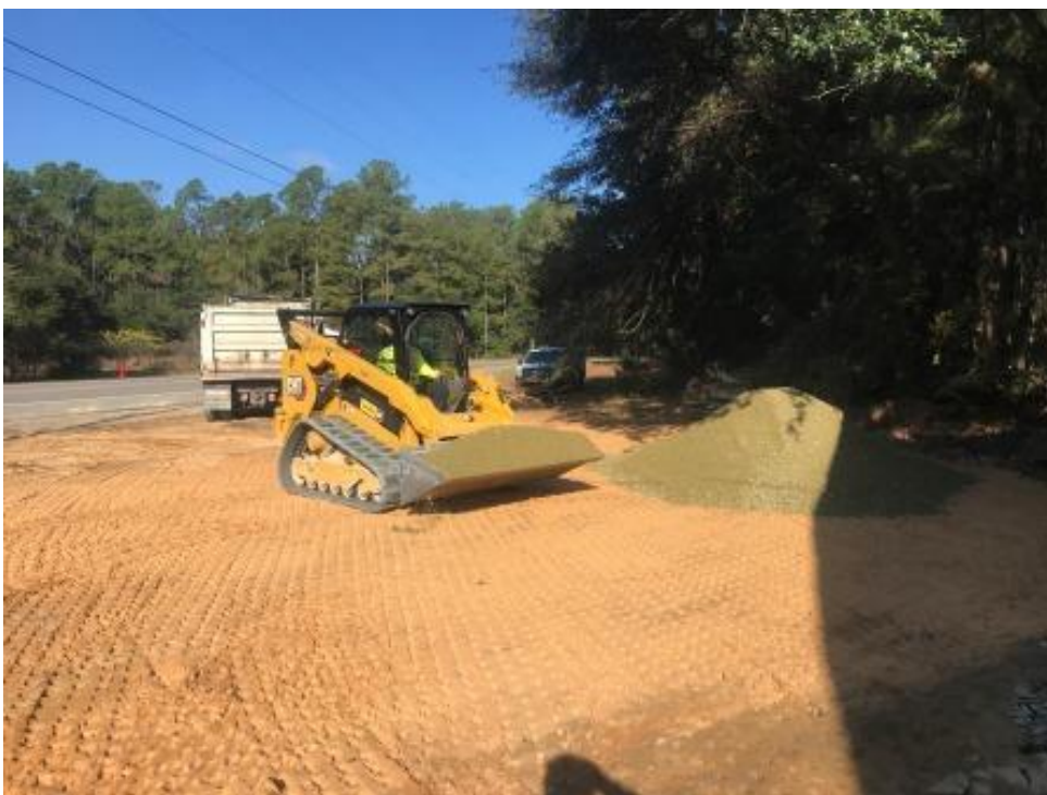
Photograph 15: EVO placing ABC stone at the top of the backfill.
