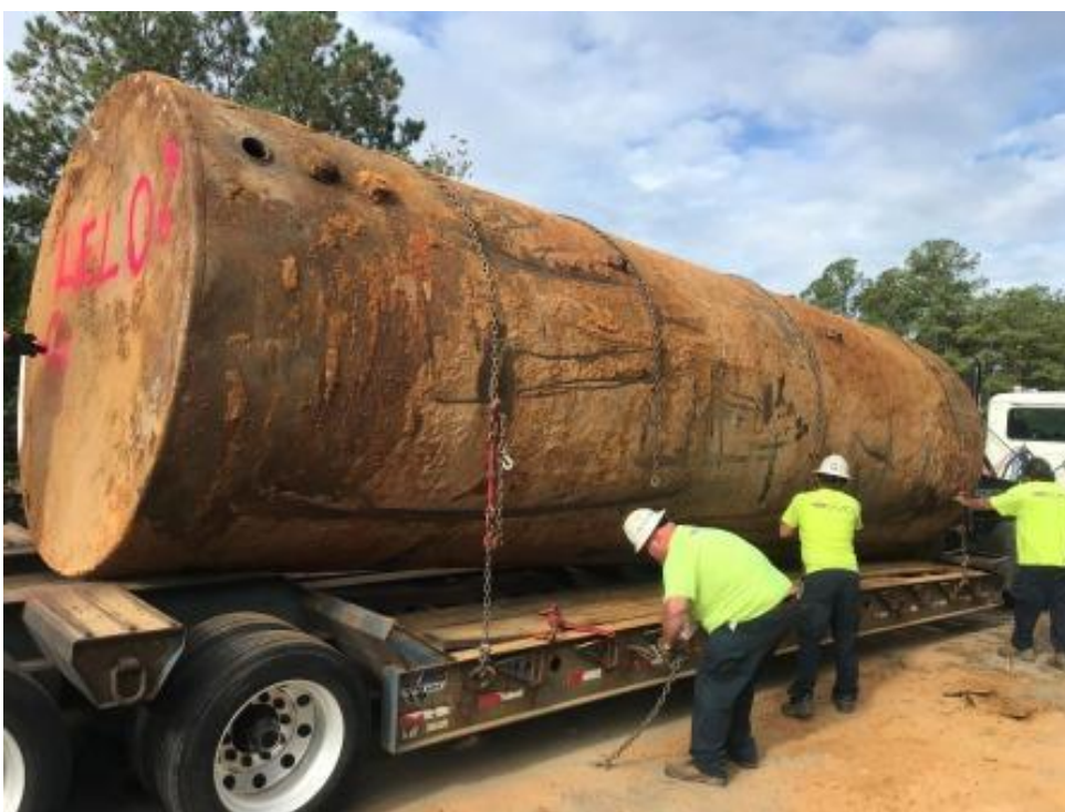
Photograph 6: EVO loading UST#1 on trailer. UST was in good condition, no holes or pitting.
