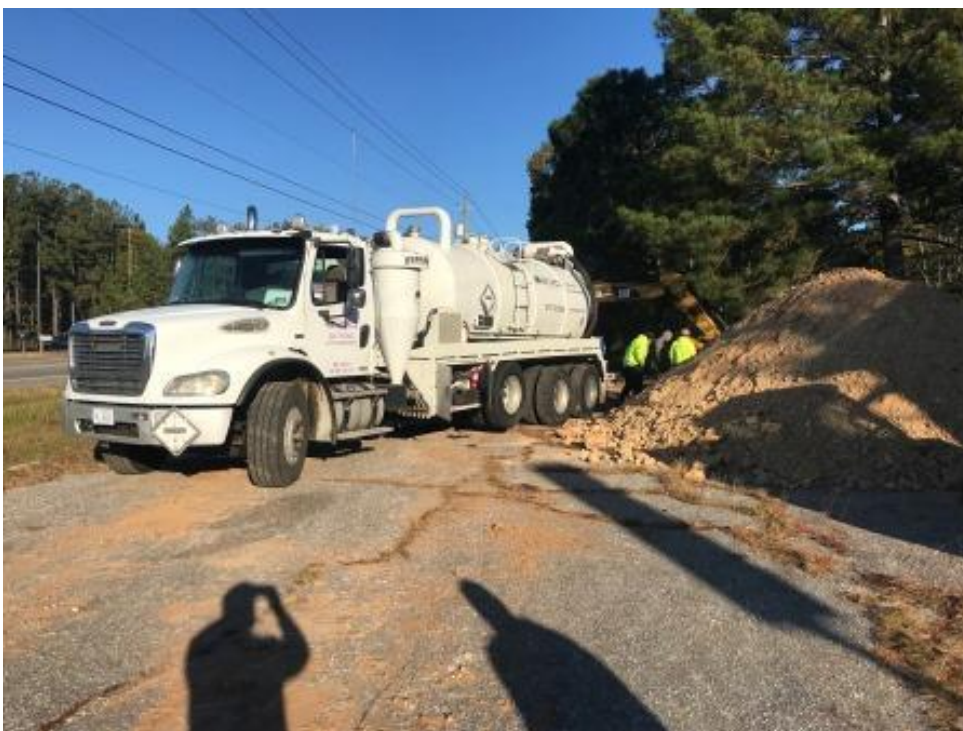
Photograph 1: EVO vacuum truck preparing to extract remaining liquids in USTs.
