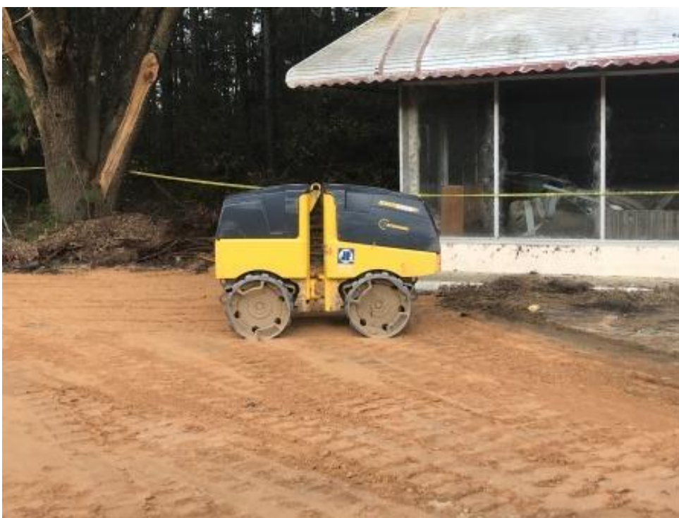
Photograph 14: Photograph of excavation backfilled to the surface.
