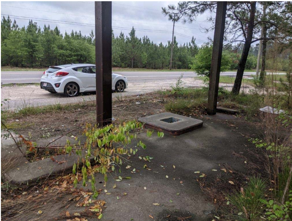
Photograph 3: Suspected dispenser islands at parcel 285, facing southeast.
