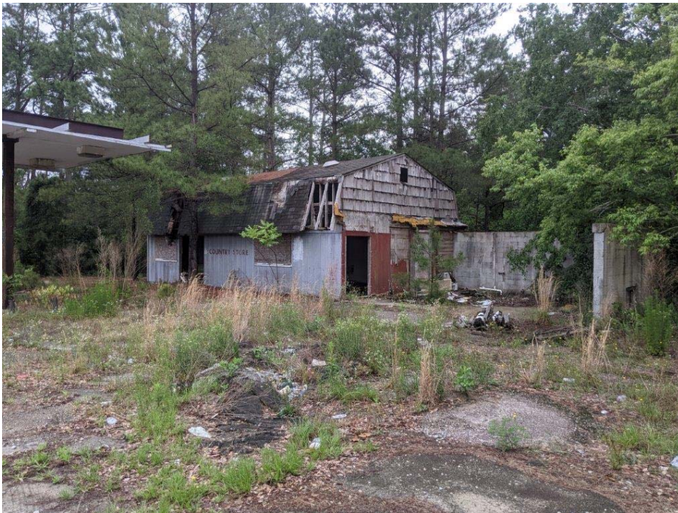
Photograph 2: Building and canopy at parcel 285, facing southwest.
