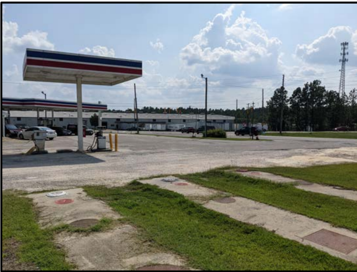
View of Survey Area (Facing Approximately South)
