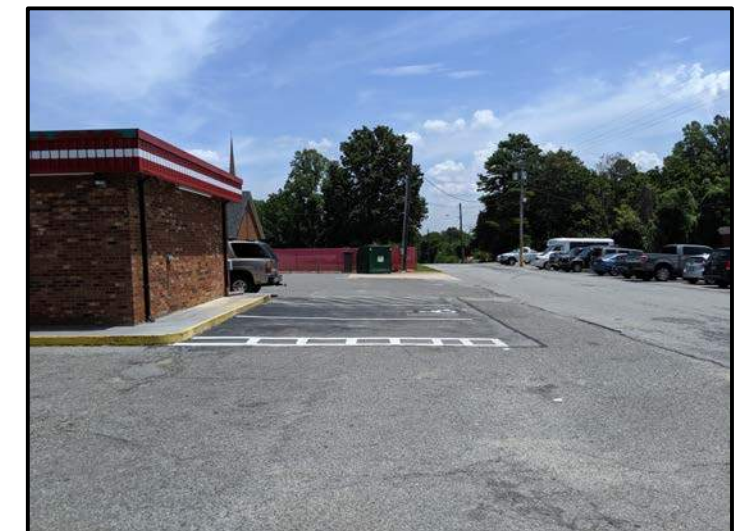
View of Survey Area (Facing Approximately East)
