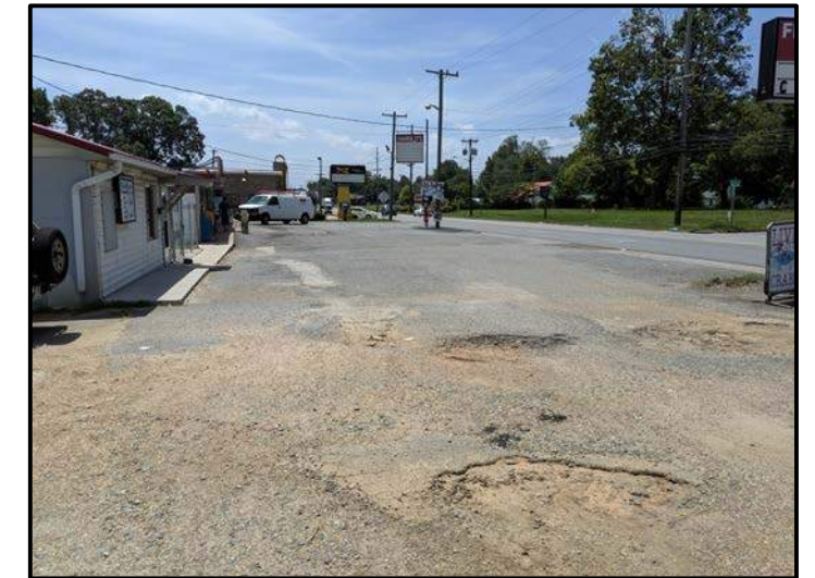
View of Survey Area (Facing Approximately South)
