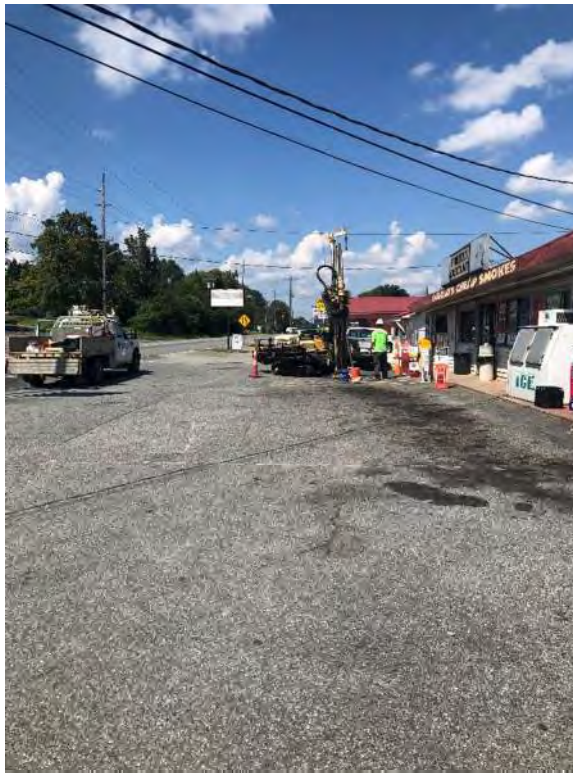
View facing northerly of Parcel 26 toward Parcels 28, 29, and 37.
