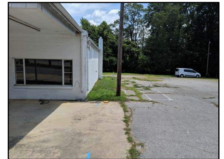
View of Survey Area (Facing Approximately East)
