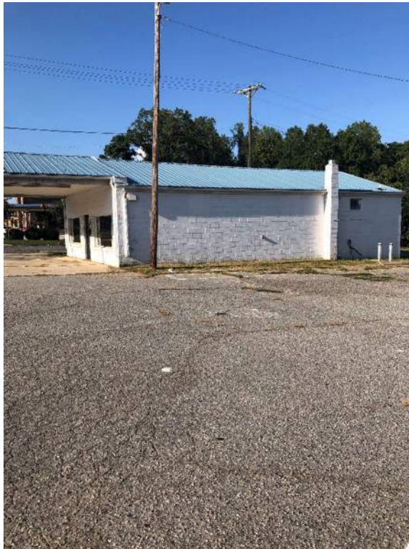
View facing northeasterly toward the vacant building on Parcel 22.
