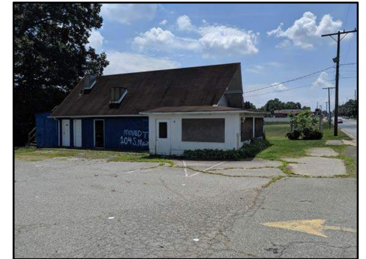
View of Survey Area (Facing Approximately South)
