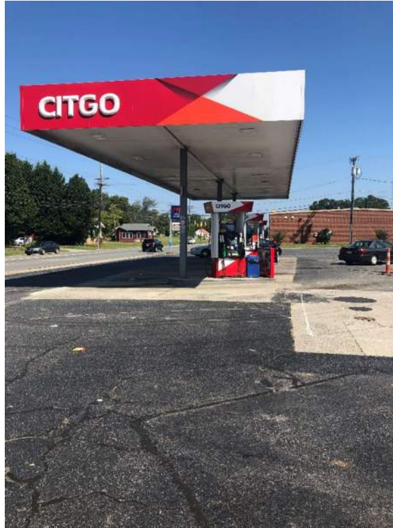
View facing north-northwesterly of the fuel canopy on Parcel 13.
