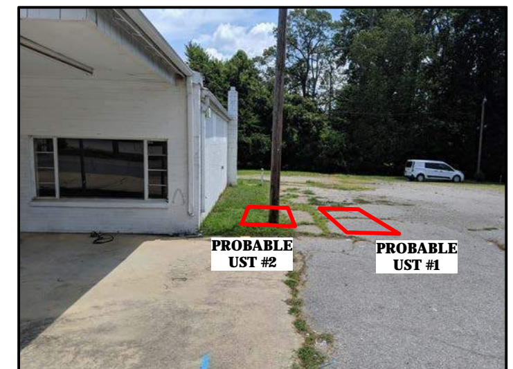
View of Two Possible USTs Facing Approximately East
