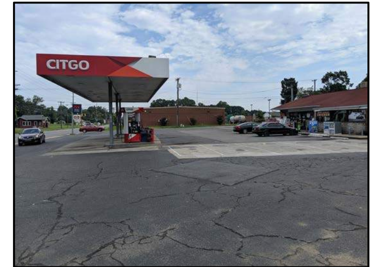
View of Survey Area (Facing Approximately North)
