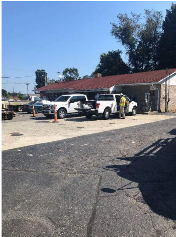
View facing northeasterly toward the convenience store located on the eastern portion of Parcel 13, featuring the UST vent pipes (center-right).
