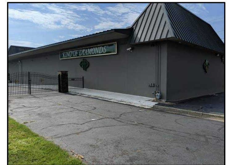
View of Survey Area (Facing Approximately East)
