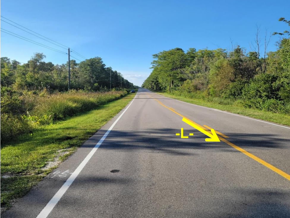
View of NC 133 looking North.
