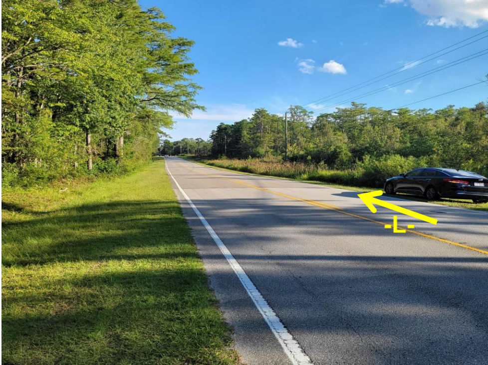
View of NC 133 looking south.
